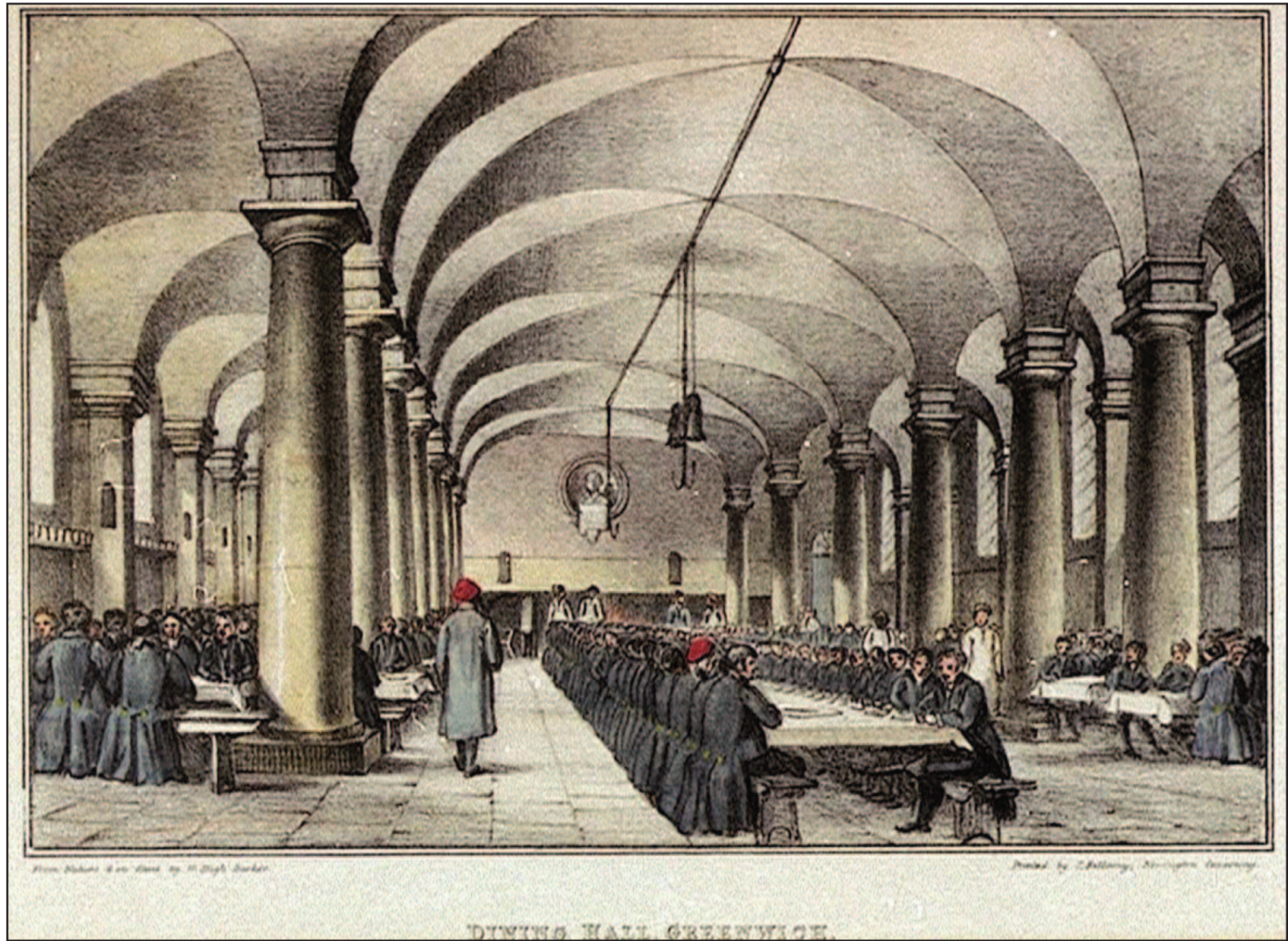
Plate 2: The dining hall of the Royal Hospital Greenwich
