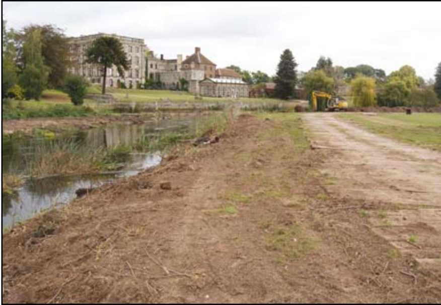
Plate 93: General view during re-profiling of river bank
