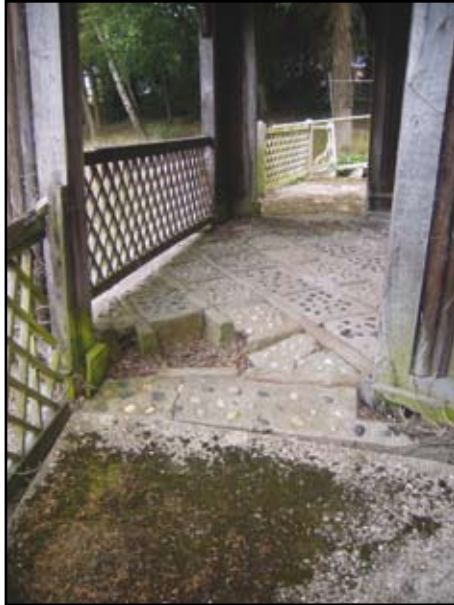
Plate 59: Gazebo Bridge, floor detail within summer house
