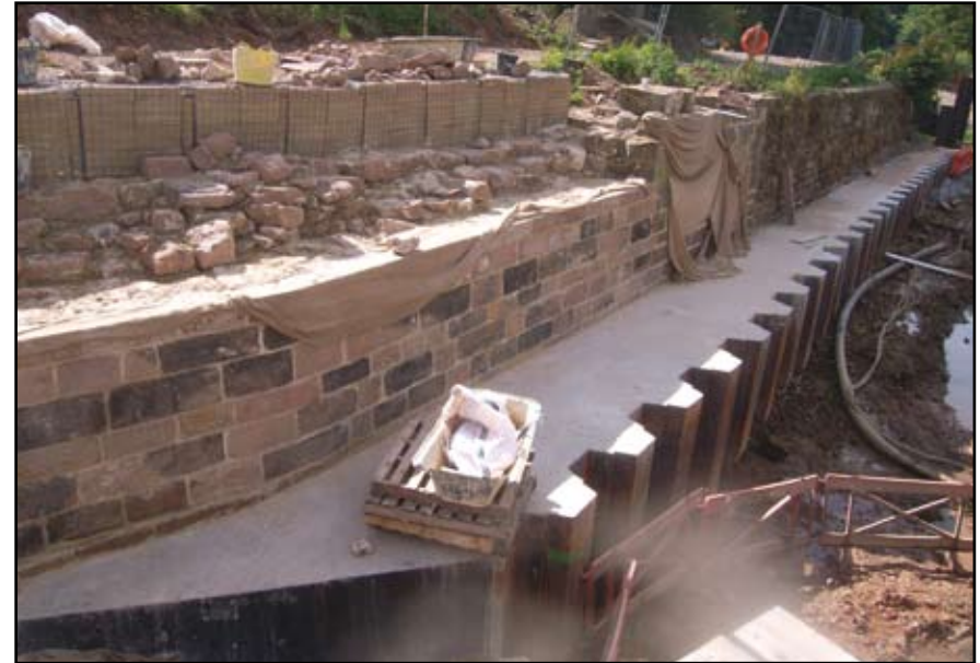
Plate 18: West Park Weir west wall during reconstruction with new concrete apron
