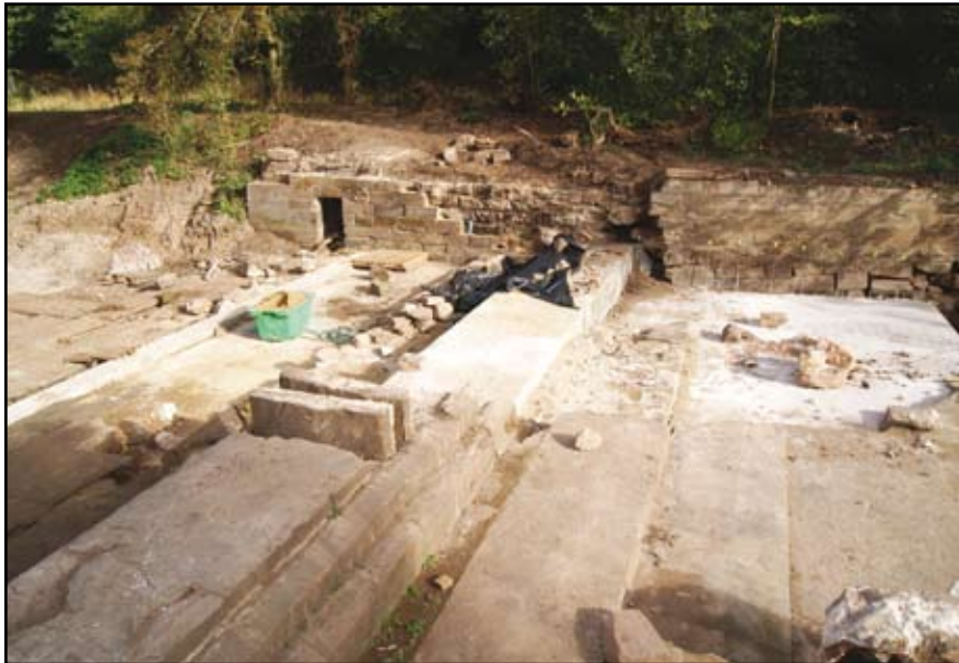
Plate 41: Island Weir, general view to north during works
