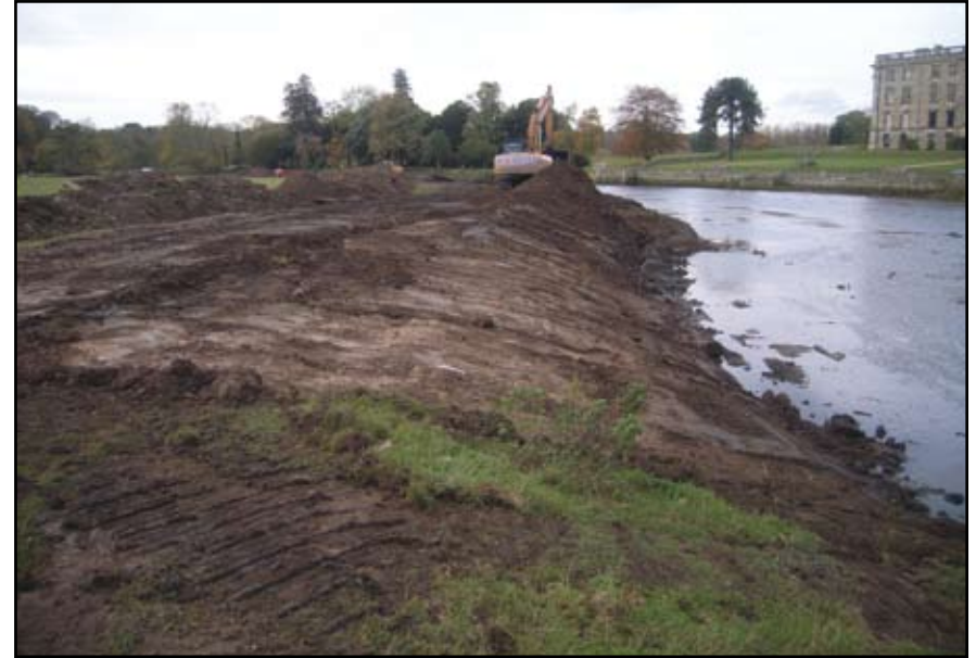
Plate 94: General view during re-profiling of river bank
