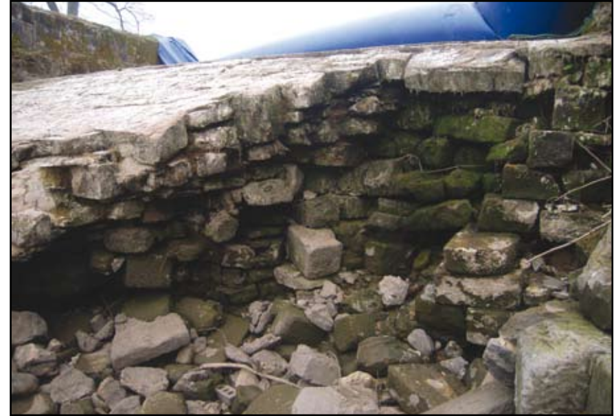
Plate 6: West Park Weir spillway detail prior to works
