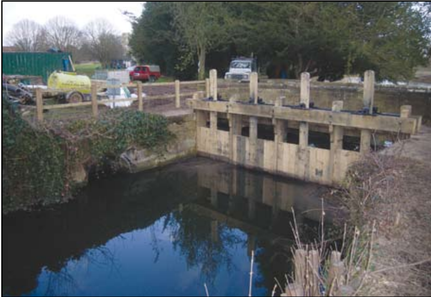
Plate 87: Abbey Mill Bridge, new replica sluice gates installed
