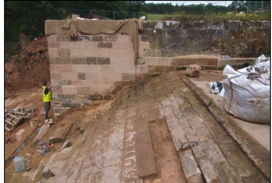
Plate 20: West Park Weir, spillway and rebuilt west wing wall
