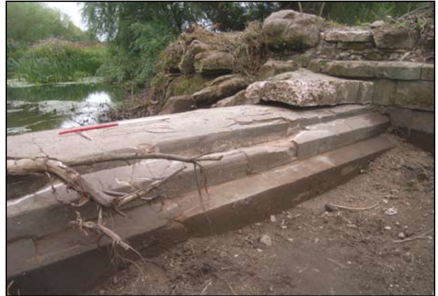
Plate 26: Island Weir, surviving stonework
