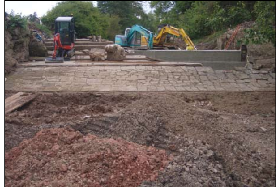
Plate 40: Island Weir, lower spillway
