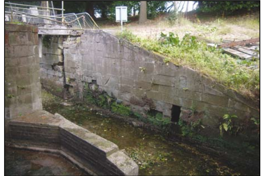
Plate 56: Gazebo Bridge, northern wall
