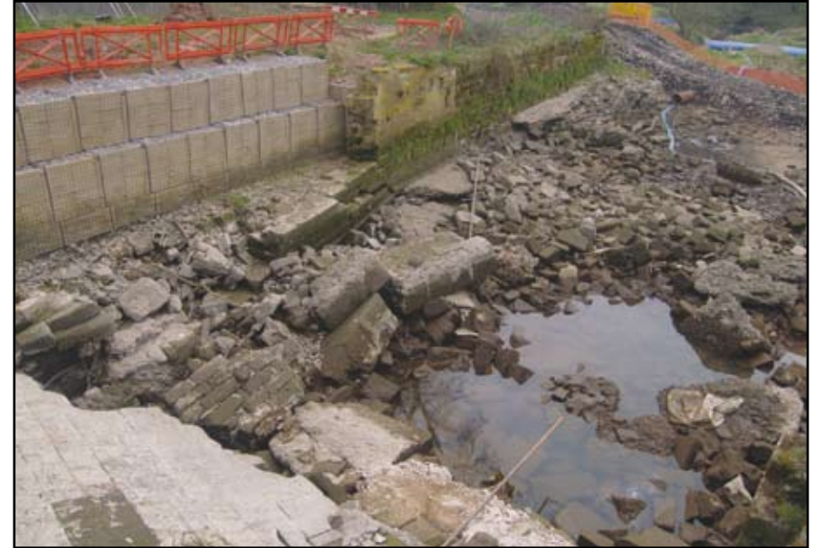
Plate 4: West Park Weir general view prior to works
