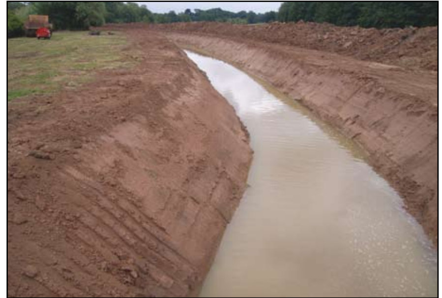
Plate 90: View of bypass channel looking east
