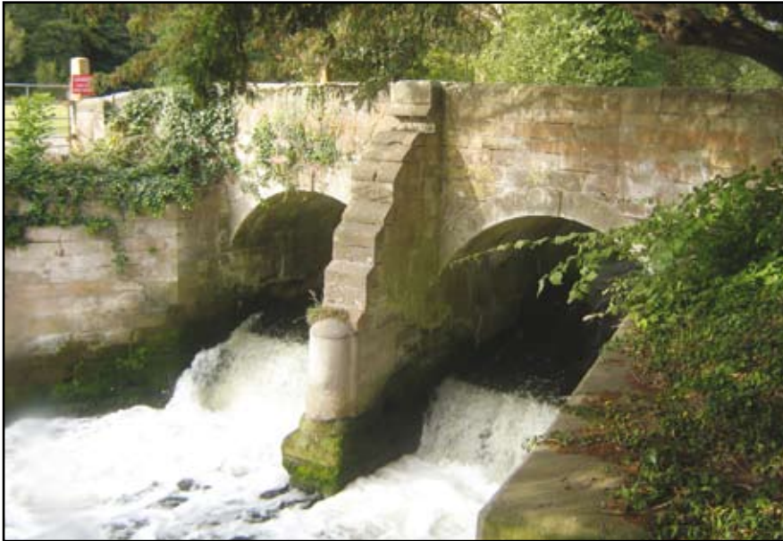
Plate 81: Abbey Mill Bridge, east portals
