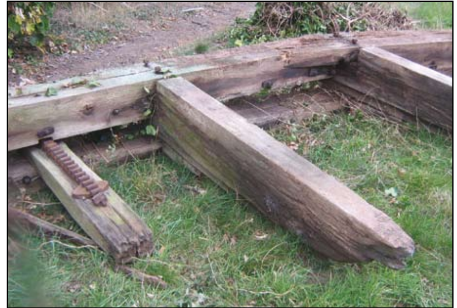
Plate 82: Abbey Mill Bridge, ex-situ sluice gate structure
