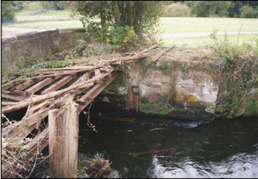
Plate 85: Abbey Mill Bridge, general view to south prior to works
