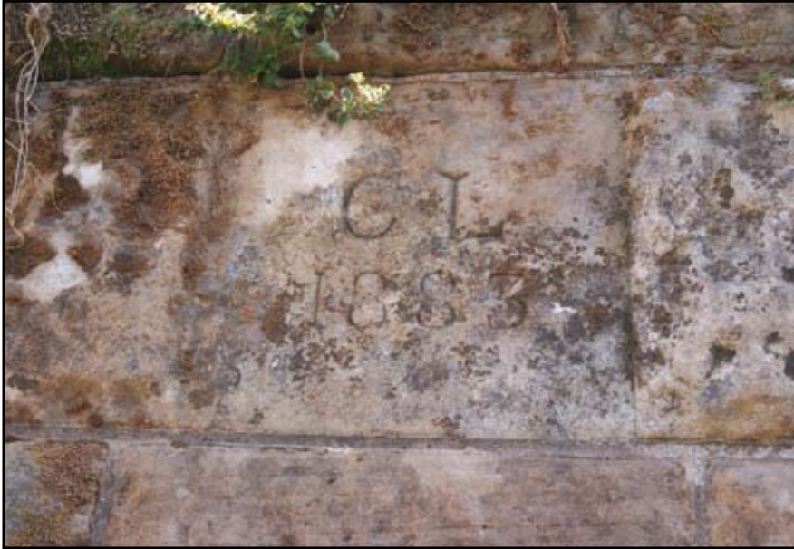
Plate 21: West Park Weir, 1883 date stone on east wall
