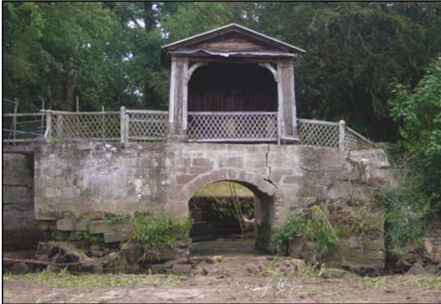
Plate 63: Gazebo Bridge, general view after de-watering
