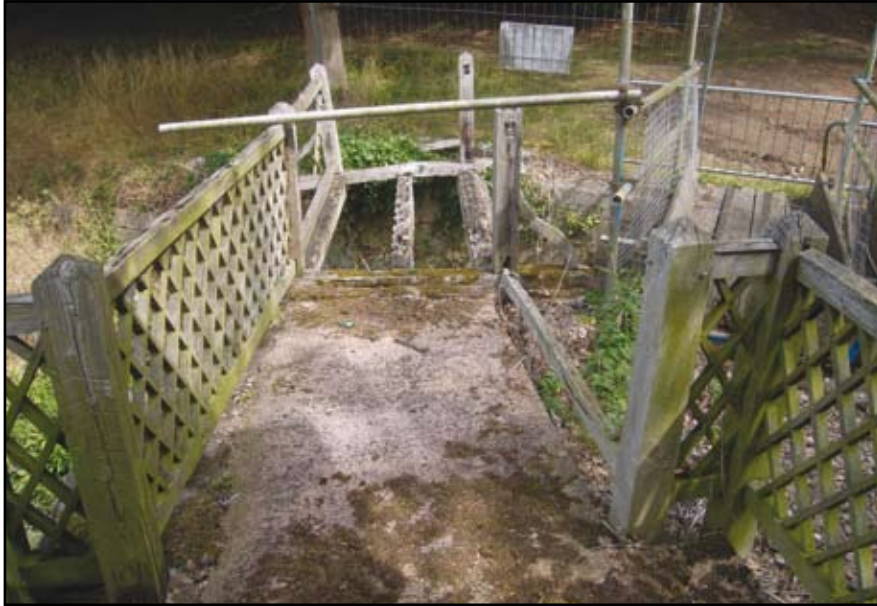
Plate 61: Gazebo Bridge, bridge floor detail
