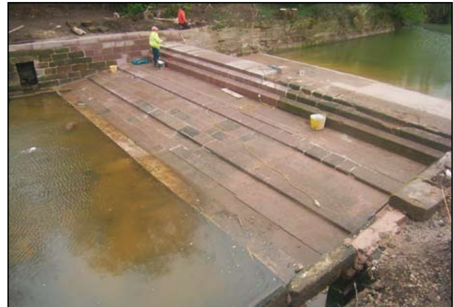
Plate 44: Island Weir, general view of rebuilt weir looking north-east
