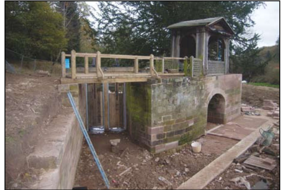
Plate 74: Gazebo Bridge, general view during works
