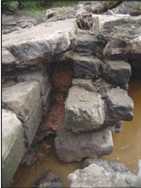
Plate 39: Island Weir, clay puddling between the upper and lower spillways
