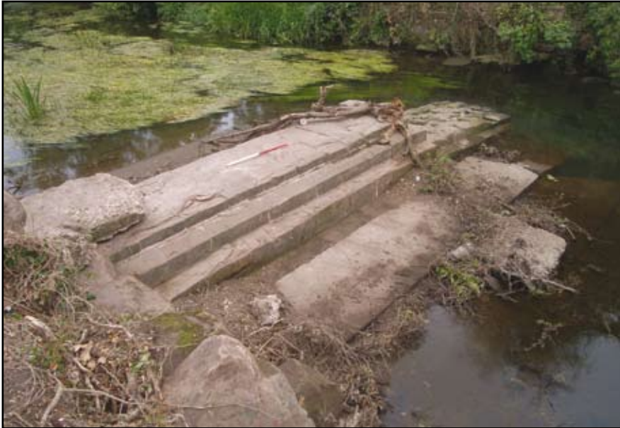
Plate 23: Island Weir, general view from SE prior to works
