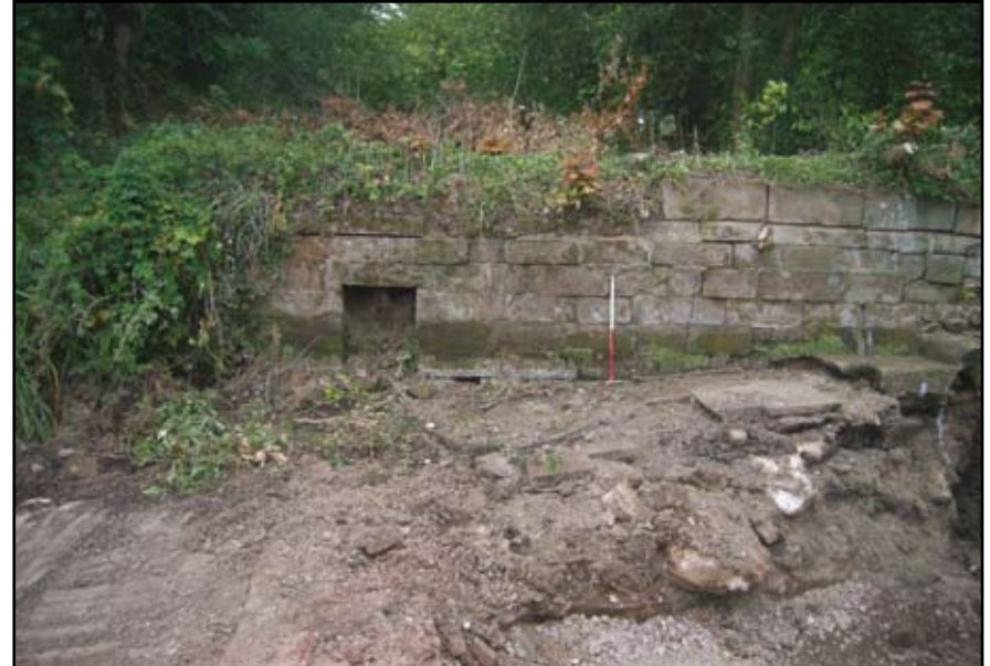
Plate 36: Island Weir, view of north wall to west of weir
