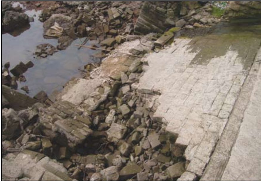
Plate 9: West Park Weir spillway before start of conservation works
