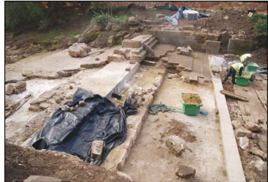
Plate 42: Island Weir, general view to south during works
