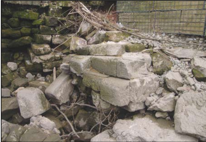
Plate 7: West Park Weir, detail of stonework to east of weir
