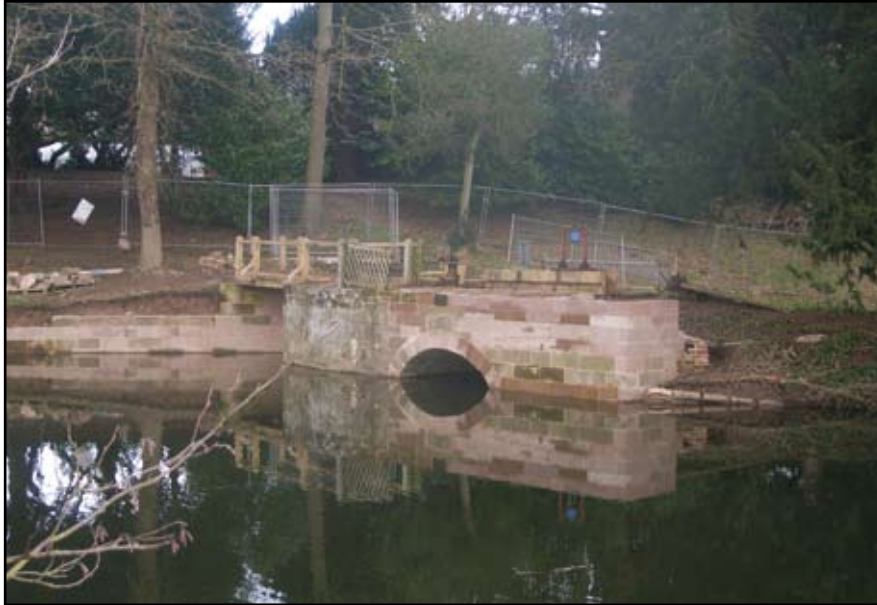
Plate 75: Gazebo Bridge, view after conservation works
