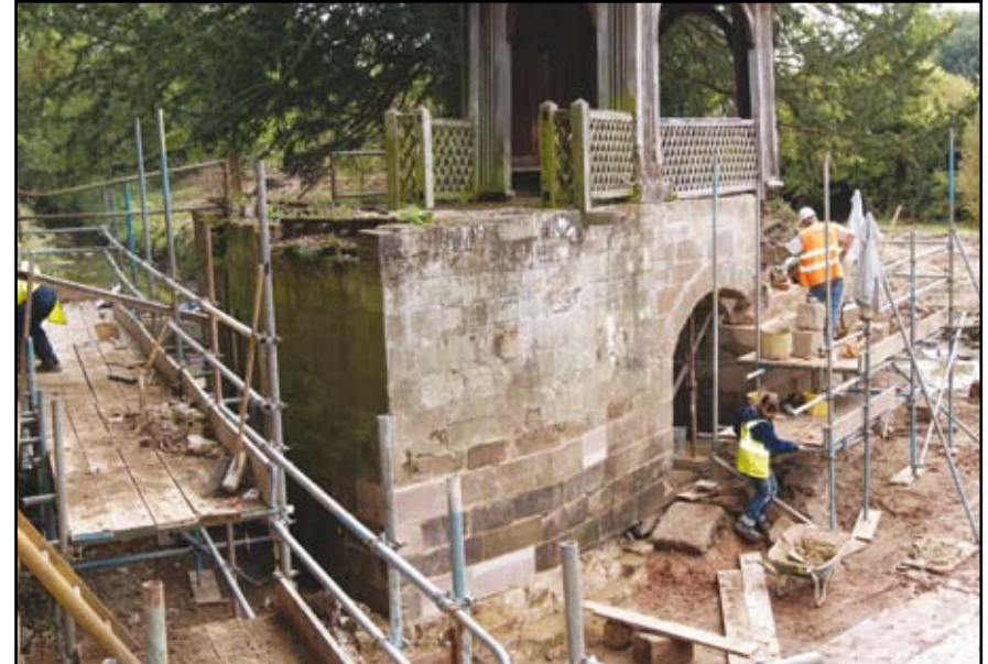
Plate 68: Gazebo Bridge, general view during conservation
