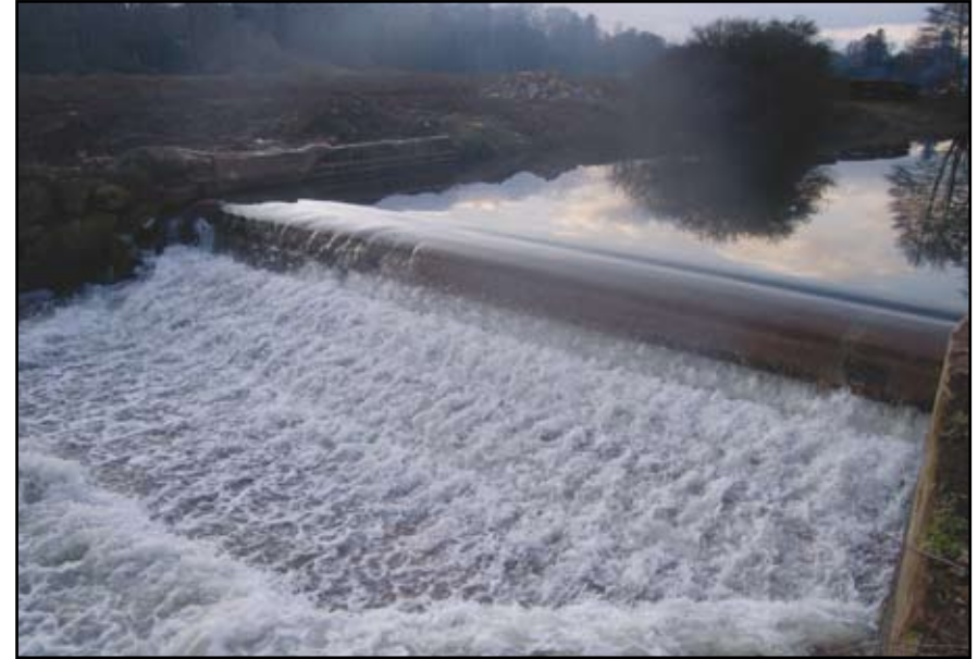
Plate 46: Island Weir, rebuilt weir from north-east
