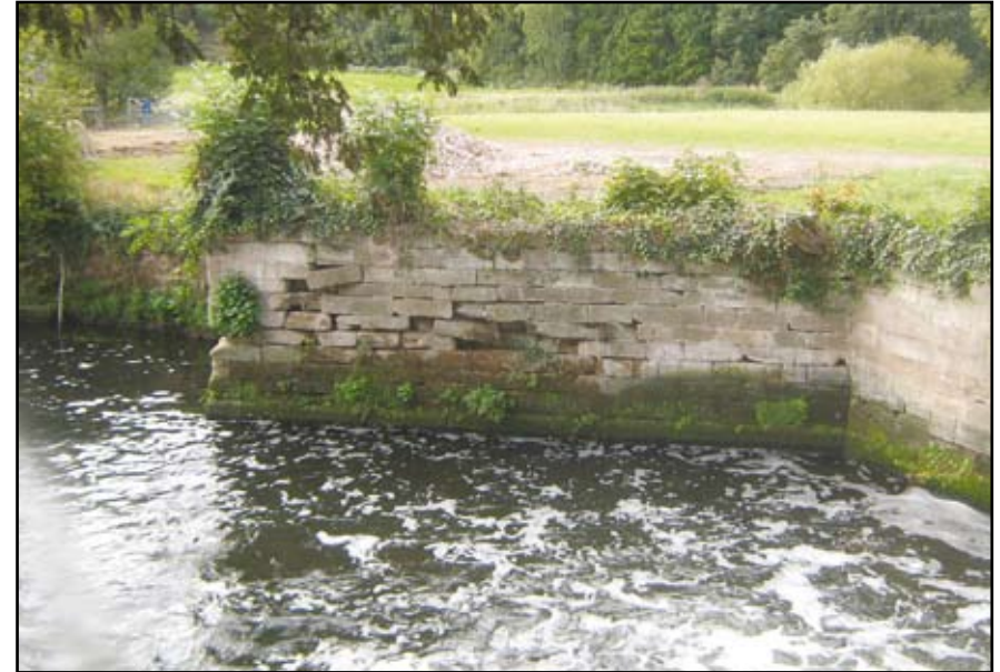
Plate 80: Abbey Mill Bridge, south wall to east of bridge
