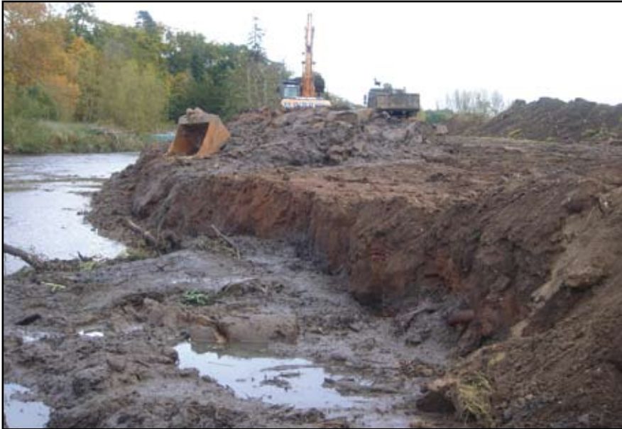
Plate 95: General view during re-profiling of river bank
