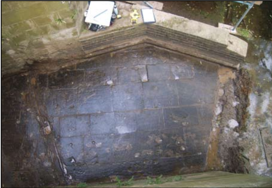
Plate 71: Gazebo Bridge, floor at SE corner
