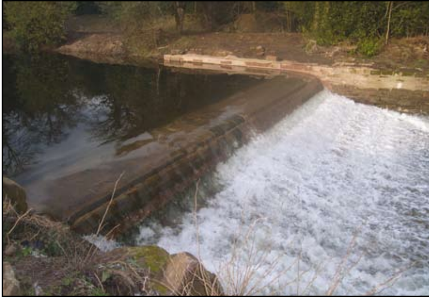
Plate 45: Island Weir, rebuilt weir from south-east
