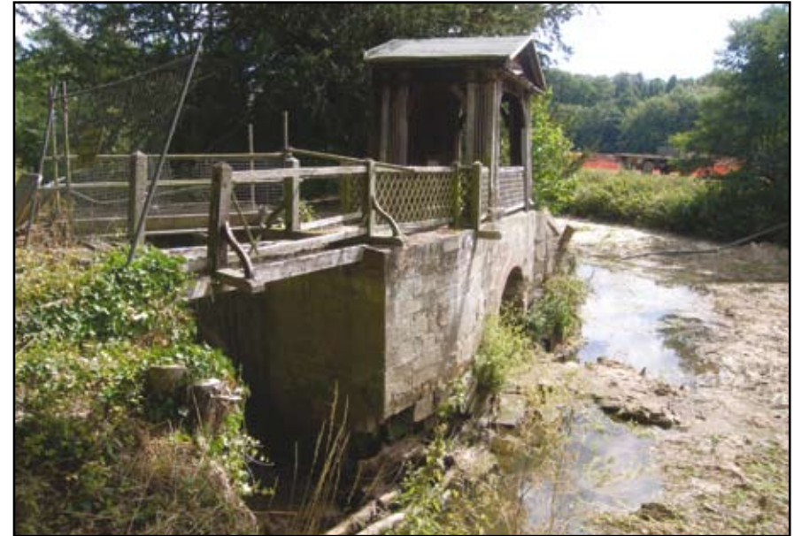
Plate 50: Gazebo Bridge, general view from north prior to work
