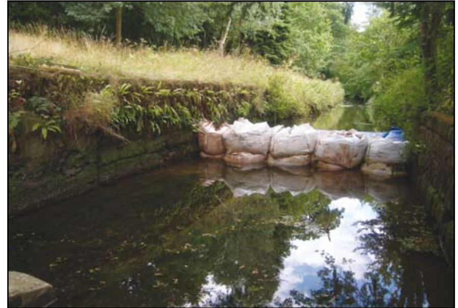
Plate 48: Gazebo Bridge, view of channel to east
