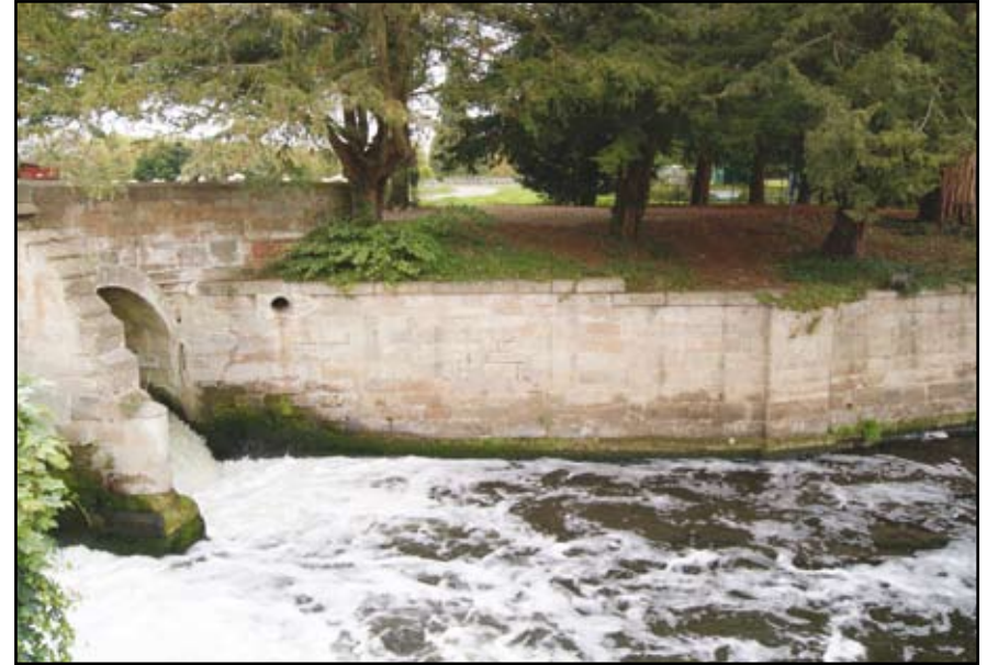
Plate 86: Abbey Mill Bridge, north wall to east of bridge
