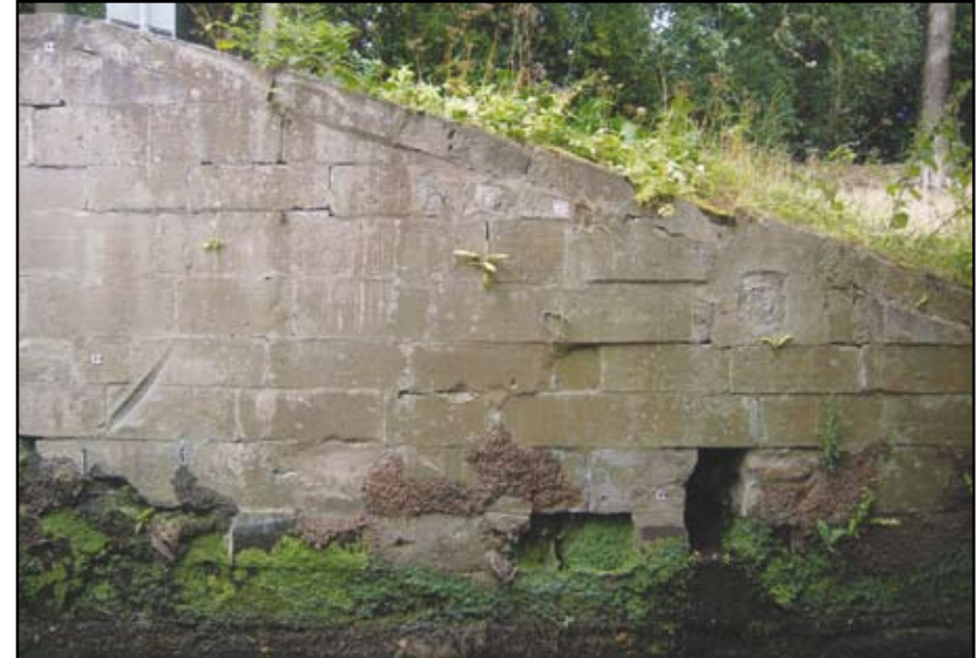
Plate 52: Gazebo Bridge, east end of north wall
