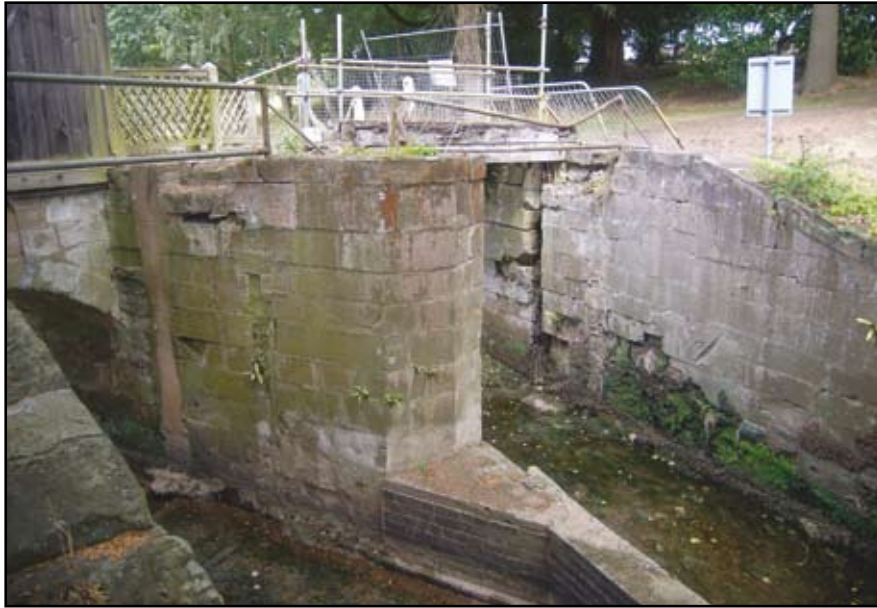
Plate 57: Gazebo Bridge, general view from south-east
