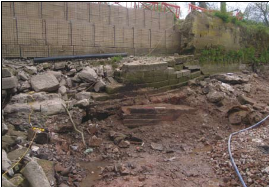
Plate 11: West Park Weir exposed masonry on east side of weir
