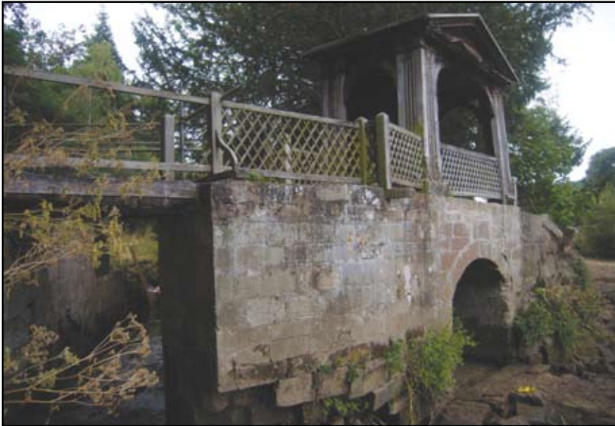
Plate 65: Gazebo Bridge, general view prior to main work
