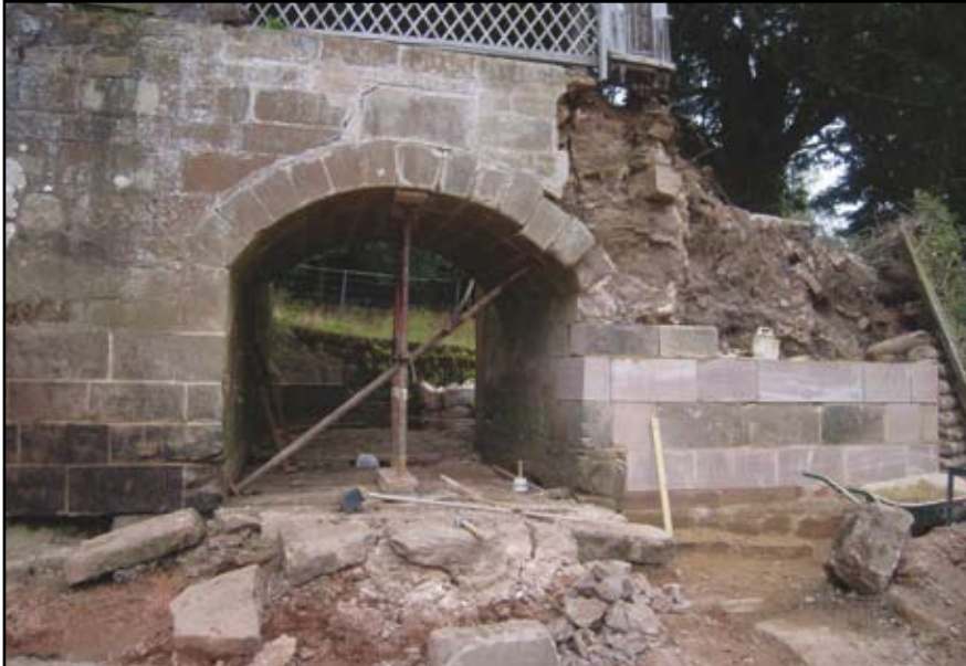
Plate 67: Gazebo Bridge, view from west during repairs
