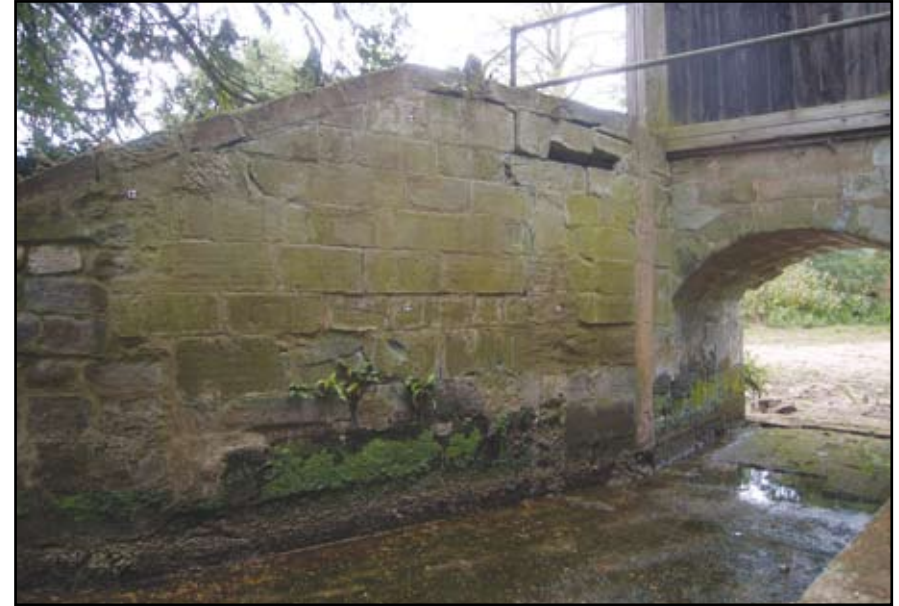
Plate 54: Gazebo Bridge, southern wall
