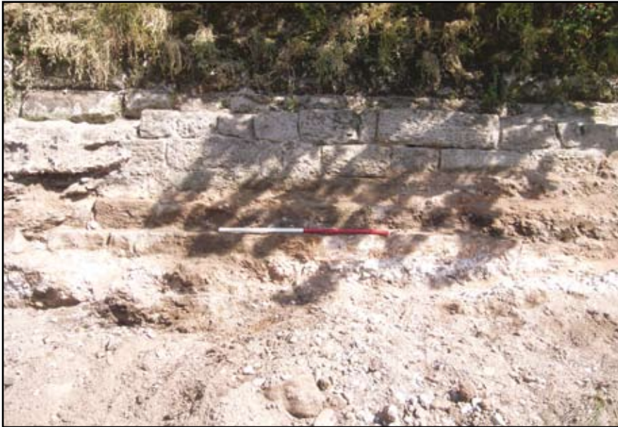
Plate 17: West Park Weir base from earlier wall along east side
