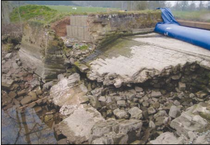
Plate 5: West Park Weir general view prior to works
