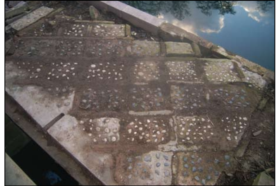
Plate 76: Gazebo Bridge, floor detail after removal of summer house
