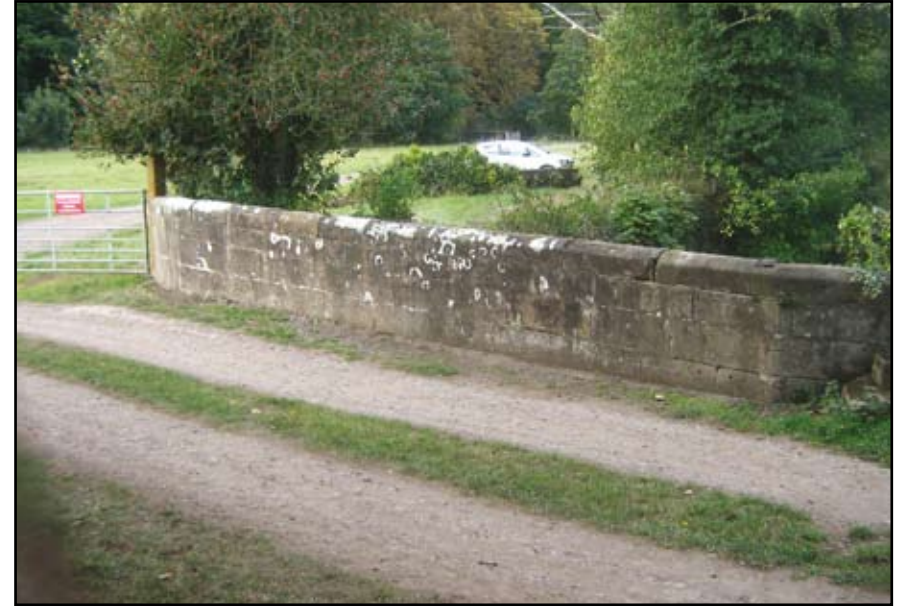
Plate 78: Abbey Mill Bridge, west parapet
