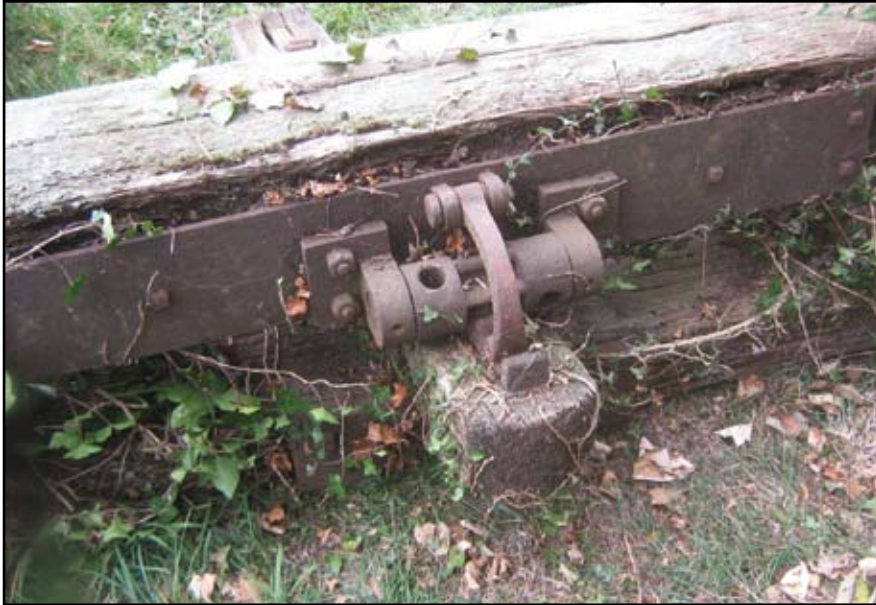
Plate 83: Abbey Mill Bridge, detail of ex-situ sluice gate structure
