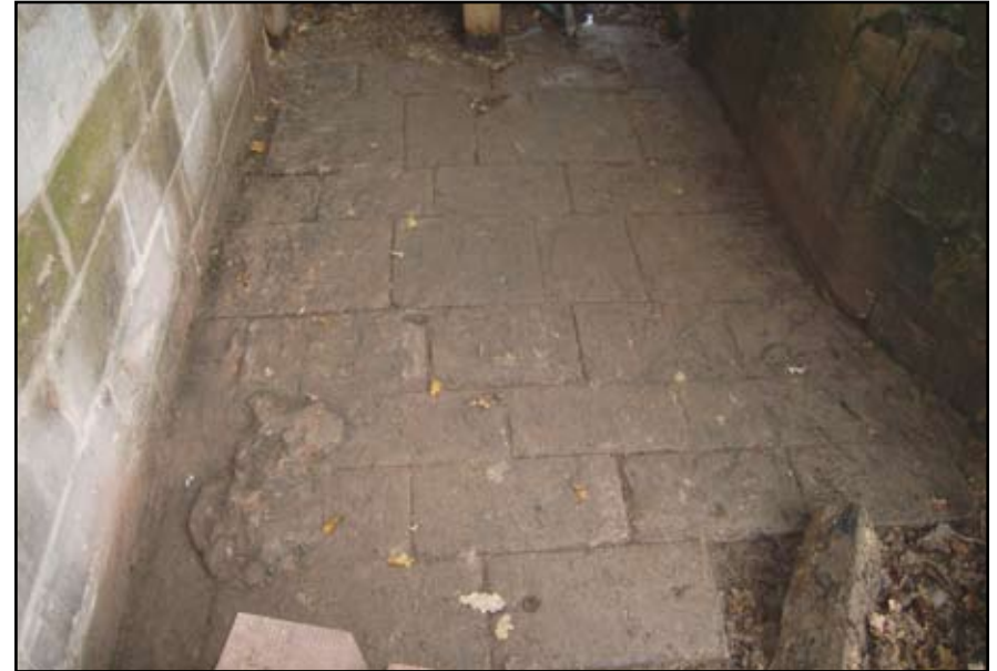
Plate 72: Gazebo Bridge, floor in southern channel beneath bridge
