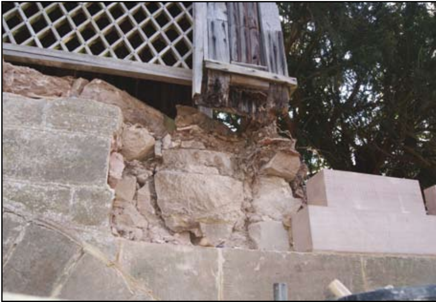
Plate 69: Gazebo Bridge, detail of summer house corner
