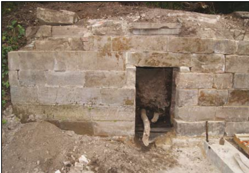
Plate 43: Island Weir, culvert portal in north wall
