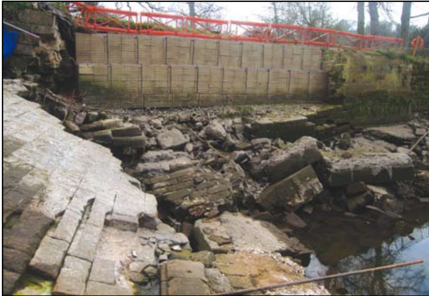
Plate 1: West Park Weir general view prior to works
