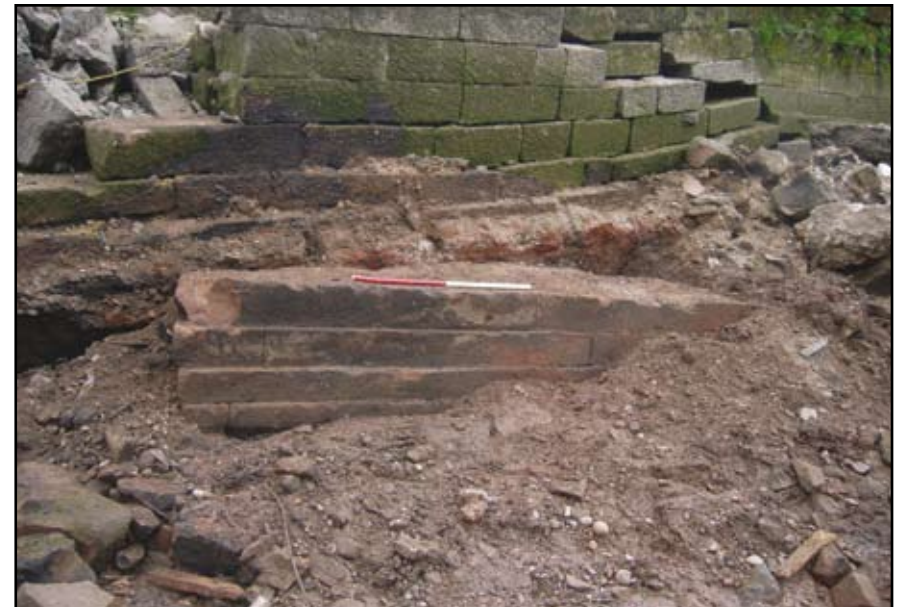
Plate 12: West Park Weir exposed masonry on east side of weir
