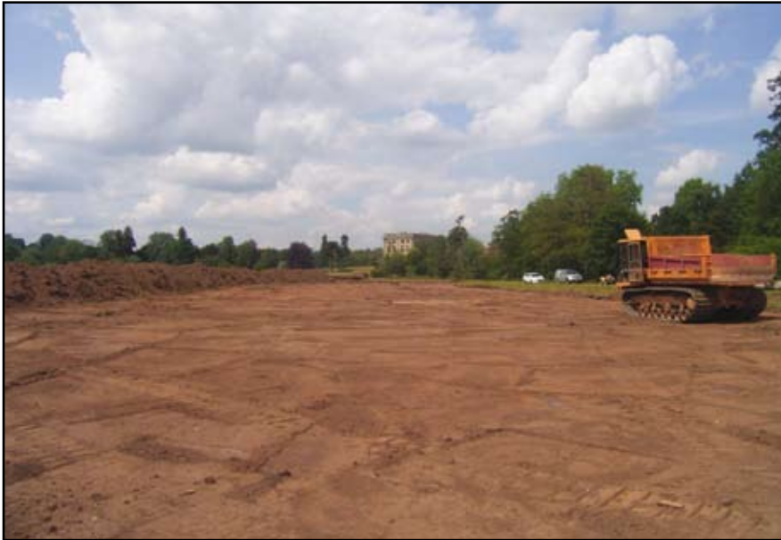
Plate 89: General view during top soil stripping for new channel
