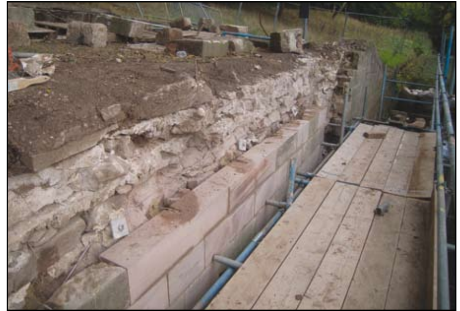
Plate 70: Gazebo Bridge, north wall during rebuilding
