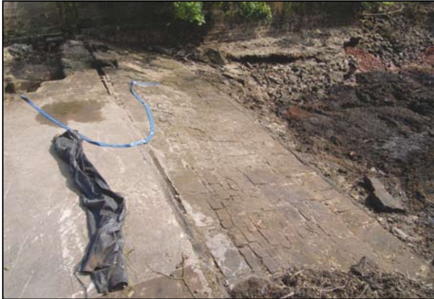
Plate 31: Island Weir, lower spillway looking north
