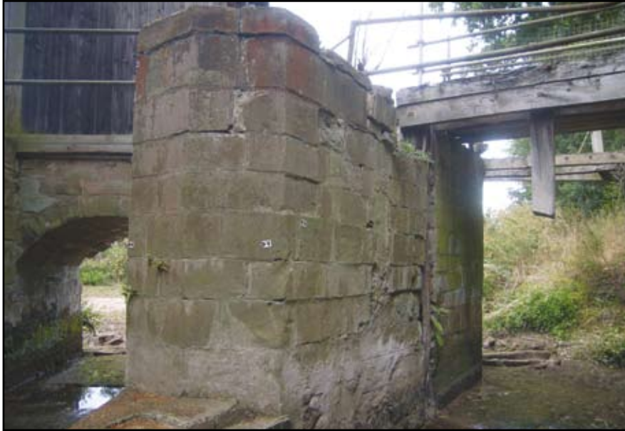
Plate 53: Gazebo Bridge, central pier
