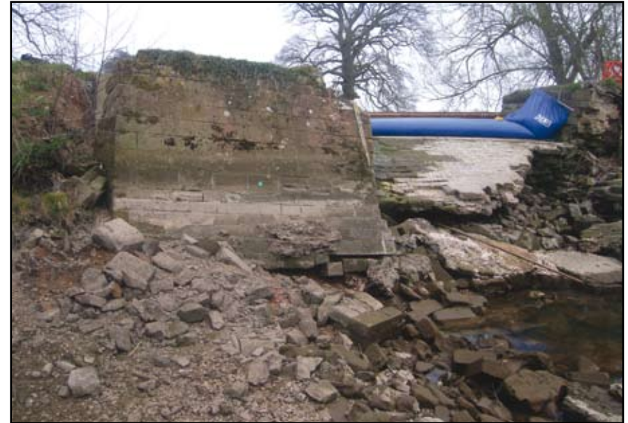
Plate 2: West Park Weir general view from south prior to works
