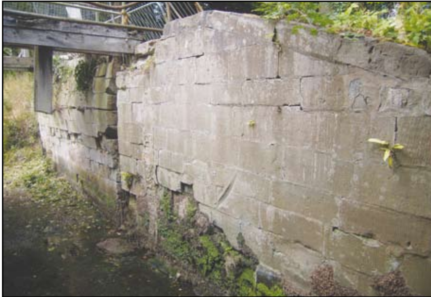
Plate 49: Gazebo Bridge, north wall
