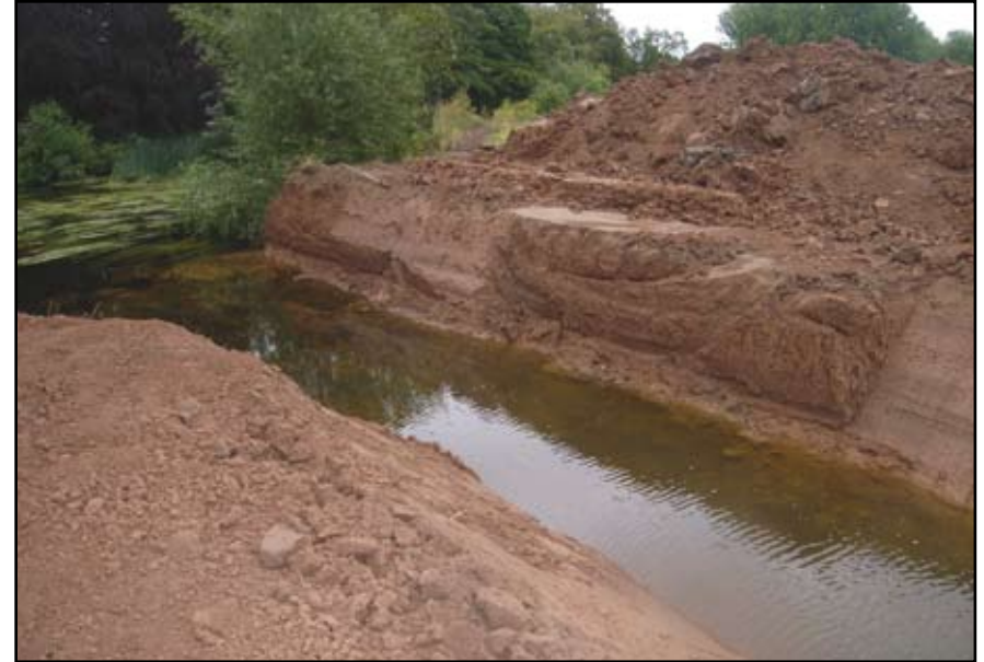
Plate 92: South-eastern end of bypass channel
