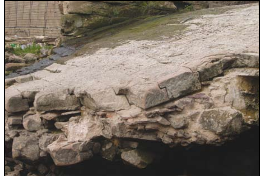
Plate 8: West Park Weir detail of spillway before works
