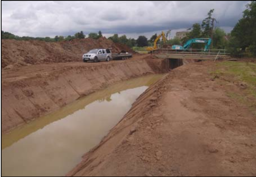
Plate 91: View during construction of bypass channel looking west
