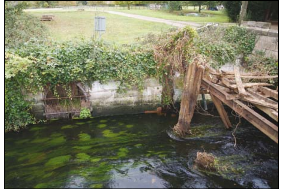
Plate 84: Abbey Mill Bridge, north wall to west of bridge
