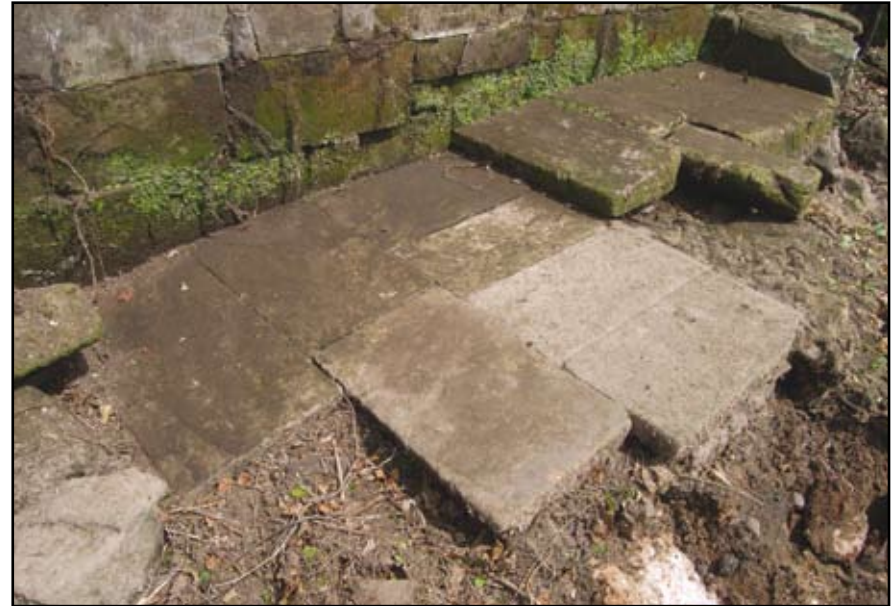
Plate 34: Island Weir, surviving fragments of spillway against north wall
