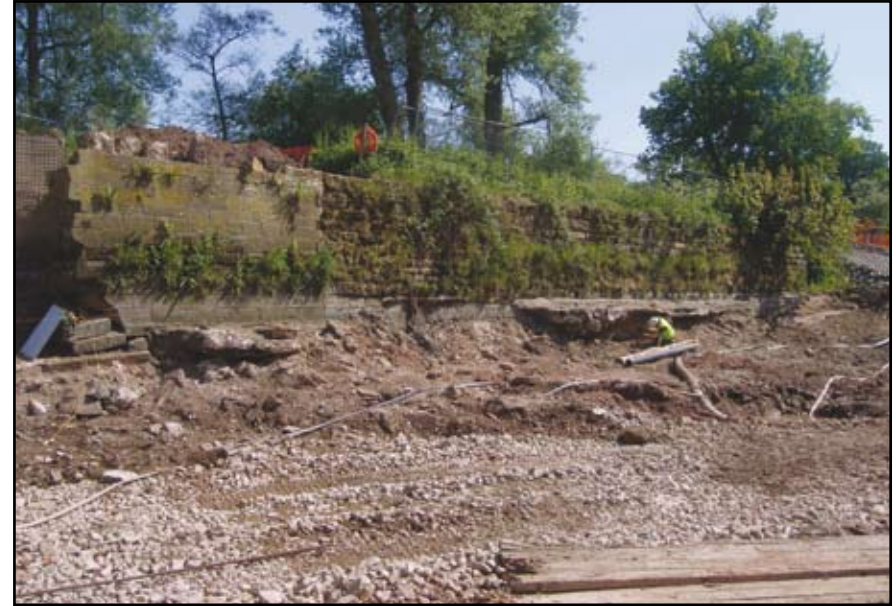
Plate 14: West Park Weir, long east wall stretching south from weir
