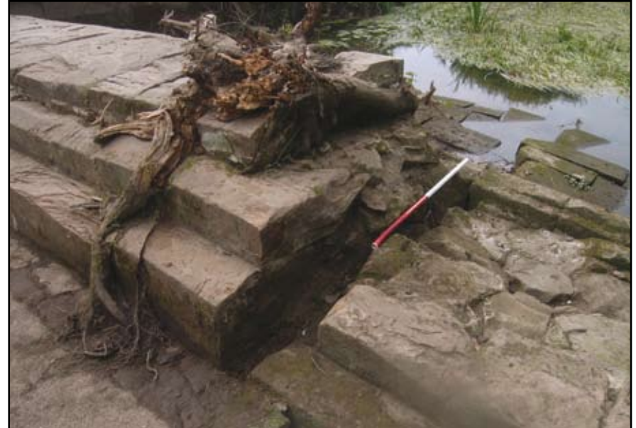
Plate 28: Island Weir, detail of truncated weir prior to works
