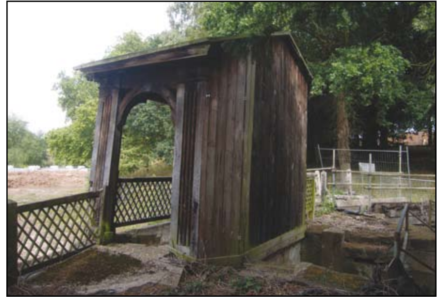
Plate 58: Gazebo Bridge, view of gazebo
