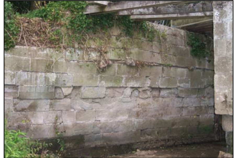
Plate 64: Gazebo Bridge, north wall prior to works
