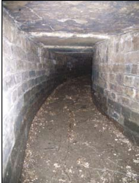
Plate 35: Island Weir, culvert by south-east corner of weir
