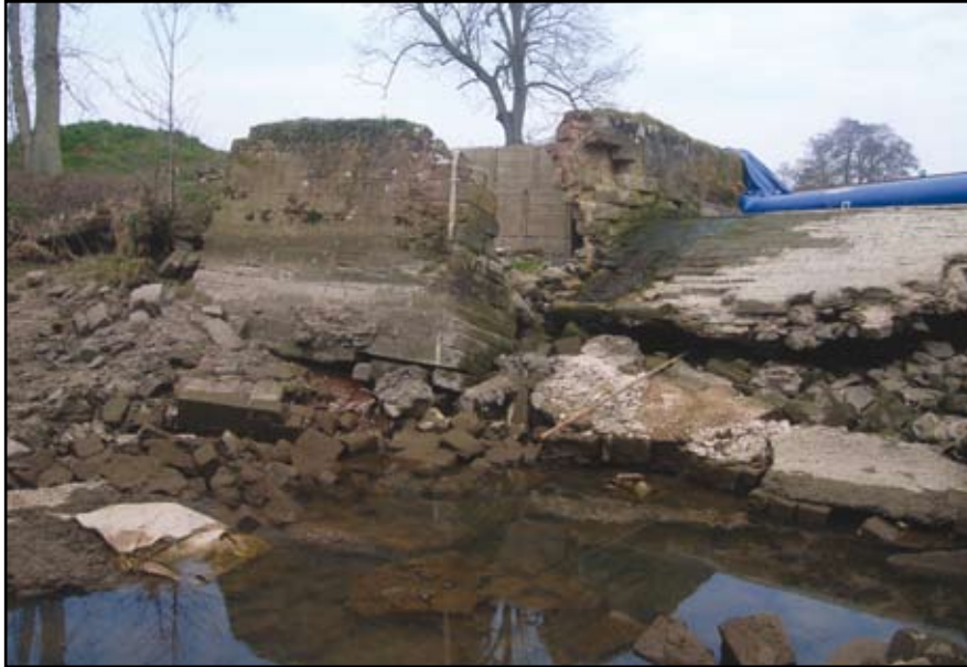
Plate 3: West Park Weir general view from south prior to works
