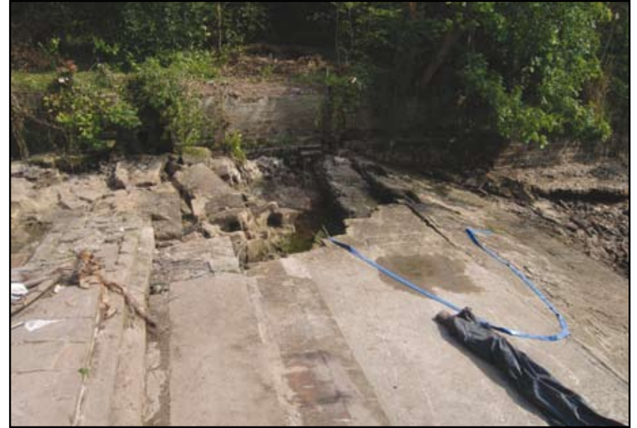
Plate 30: Island Weir, general view looking north prior to work
