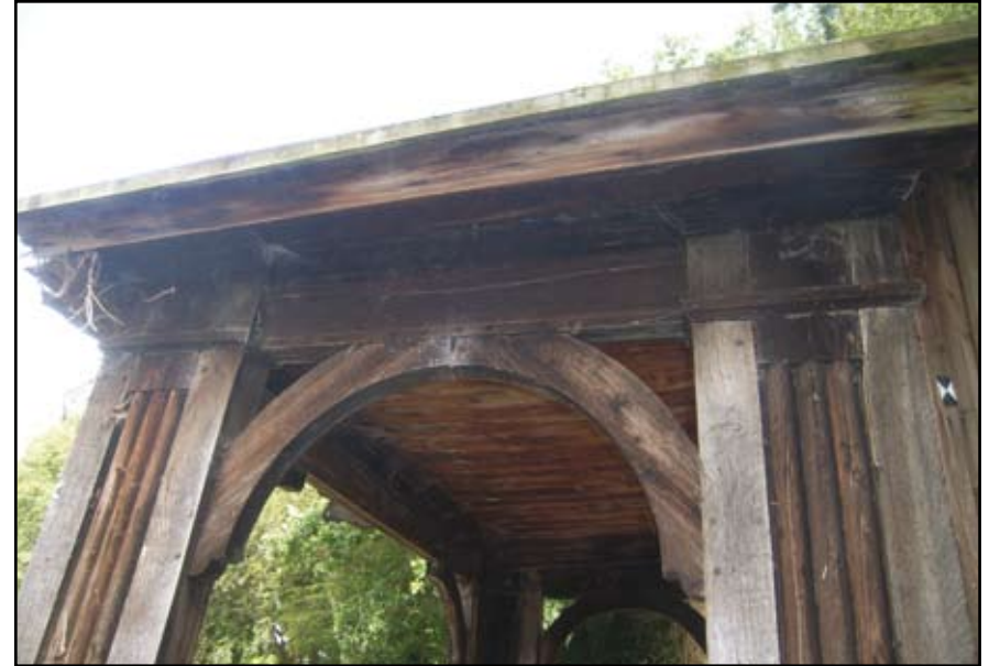
Plate 60: Gazebo Bridge, detail of summer house roof
