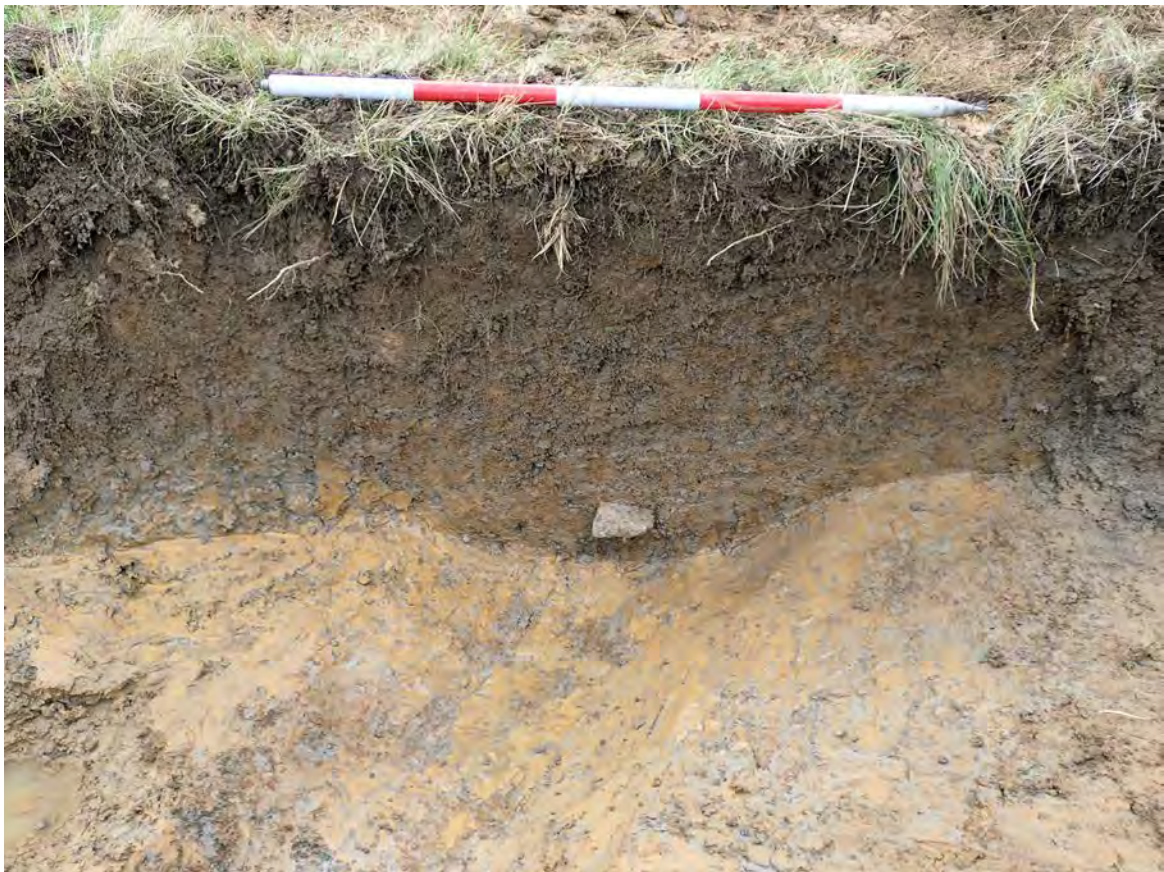
Plate 12: Ditch 5305, view to S
