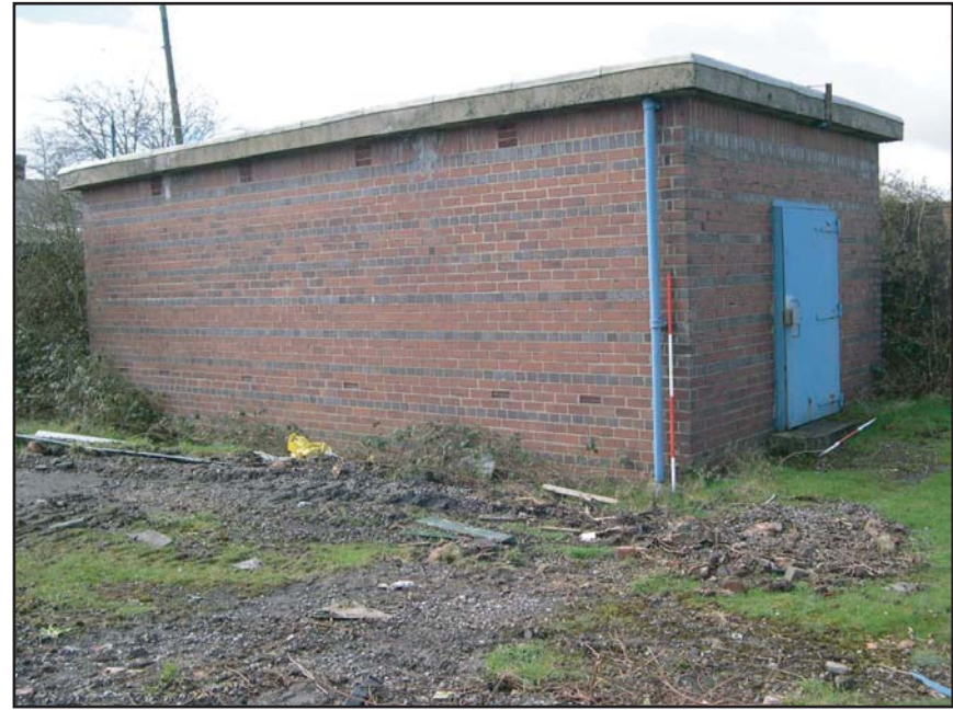
Plate 18: Substation viewed from North
