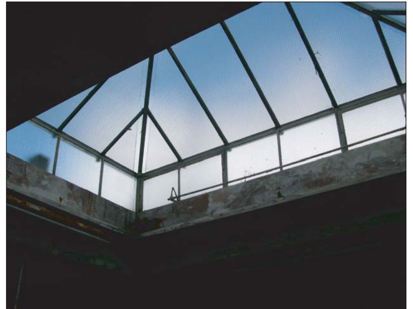
Plate 16: View of skylight in Room 1
