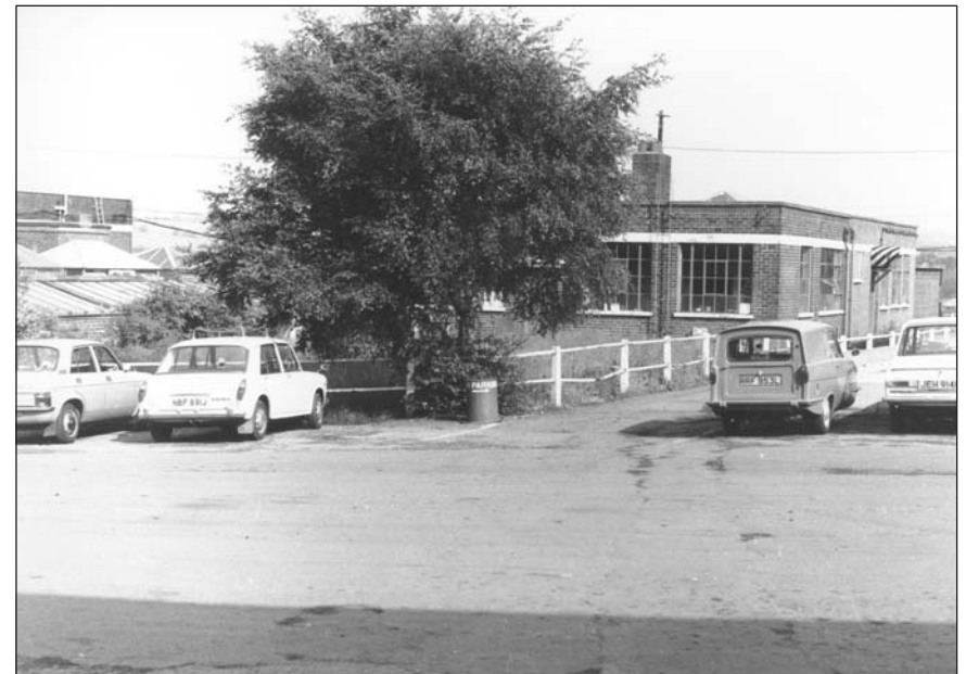
Plate 8: The upper laboratory external elevation facing NW
