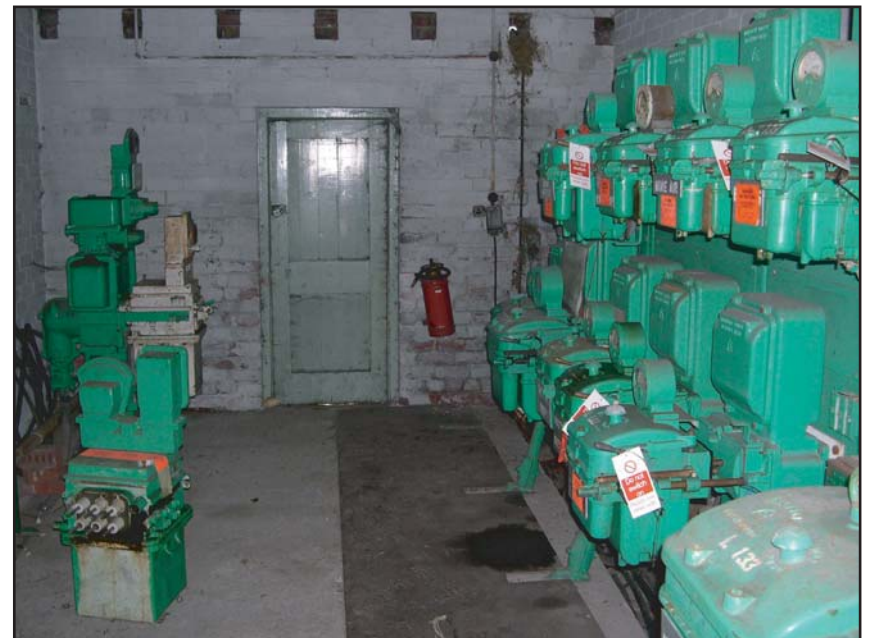
Plate 24: View from the south-east
