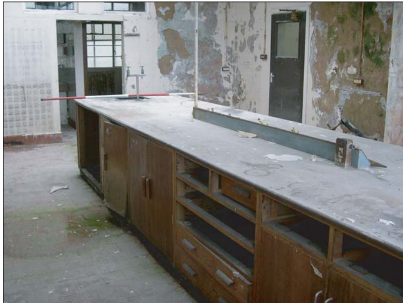
Plate 15: View from west in Room 1
