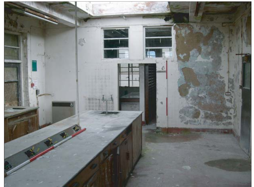
Plate 12: View from south within Room 1
