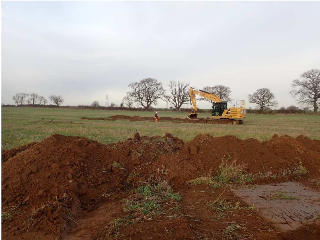
Plate 1: Working shot of trench excavations
