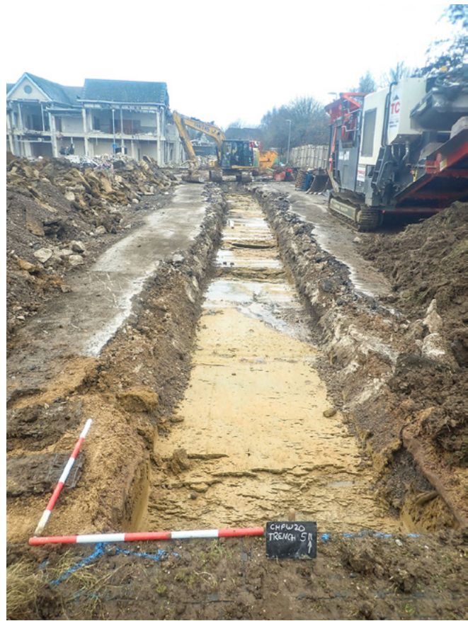
Plate 1: Overall shot of Trench 5
