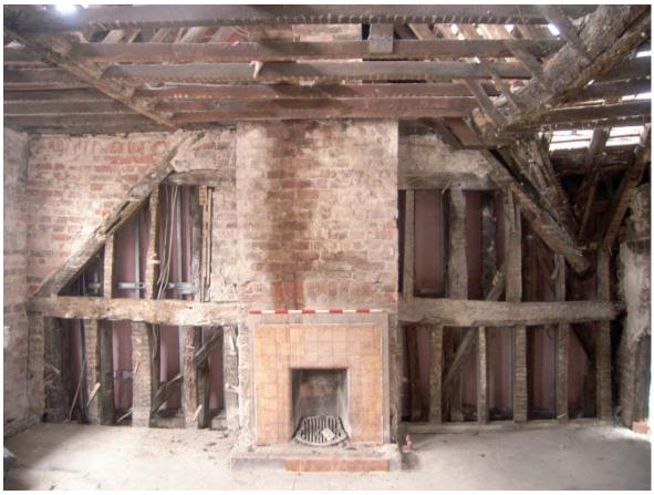
Plate 13: North wall incorporating truss three and later chimneybreast and additions; note empty joints for original clasped purlins
