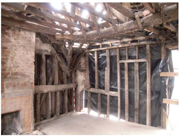
Plate 17: North east corner showing framing of east wall in north bay on right
