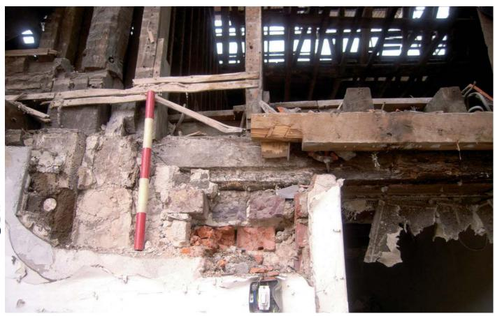
Plate 7: Main post and plate with rebate in rear wall exposed during works
