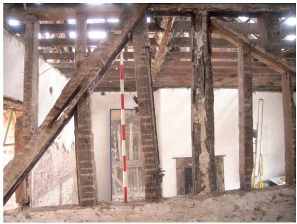
Plate 11: Reused ovolo moulded window jambs and east queen strut in truss one, note also mortice for windbrace in pricipal rafter
