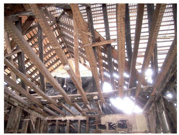
Plate 18: View of roof east from central bay showing early smoke blackened rafters and later gable and ceiling joists
