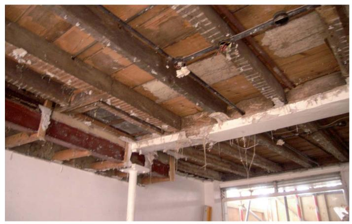
Plate 8: Floor structure; note girder and stanchion supporting bridging beam and chimney breast
