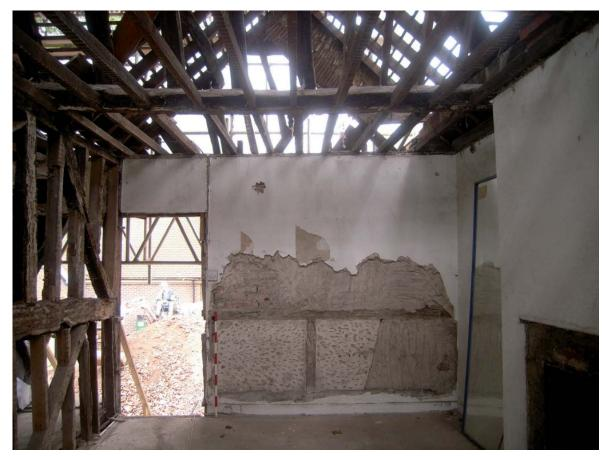
Plate 14: East wall in south bay showing old wallplate and earlier infill in lower panels
