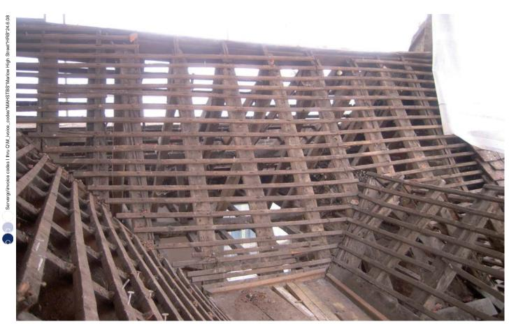
Plate 5: Rear slope of roof at north end with later gable extensions
