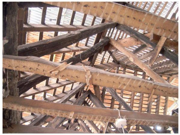
Plate 12: Smoke blackened rafters above later ceiling joists
