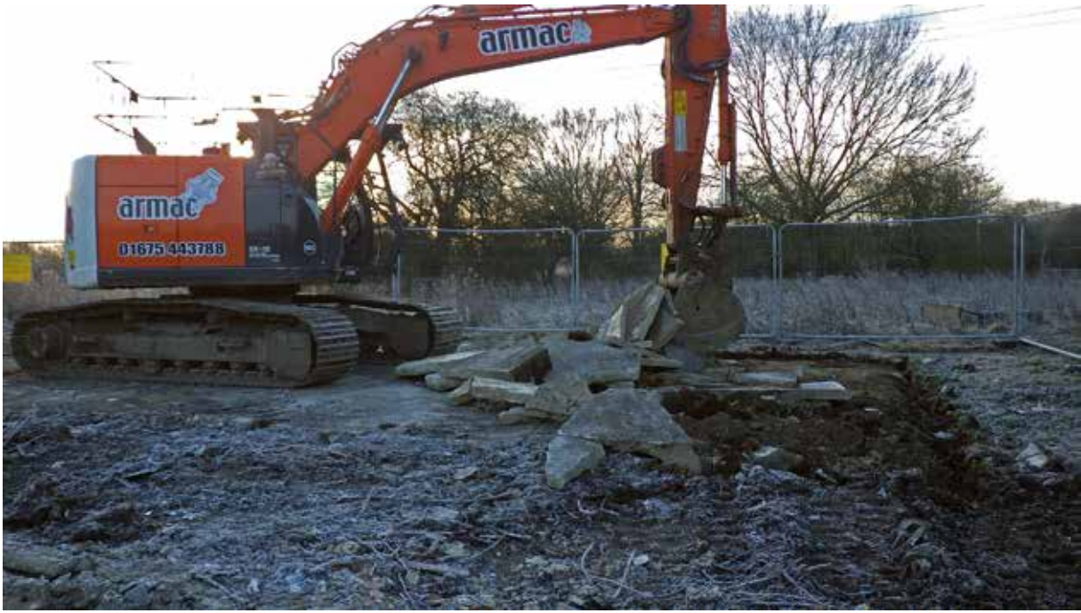
Plate 1: Rodney House concrete slab removal
