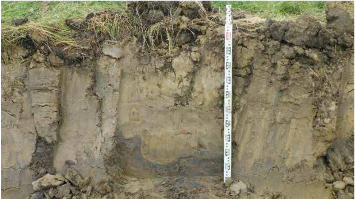
Plate 6: Trench 64 section showing the thickness of the redeposited natural clay
