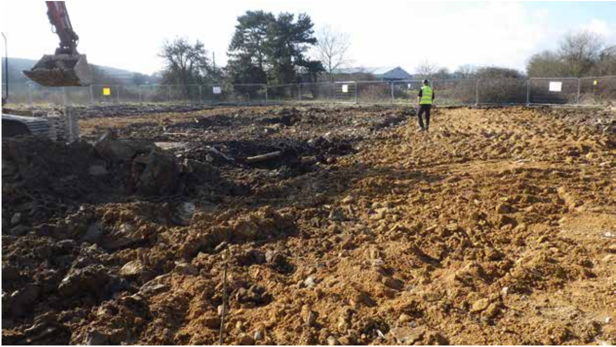
Plate 3: Rodney House view SSW showing exposed hard core rubble layers
