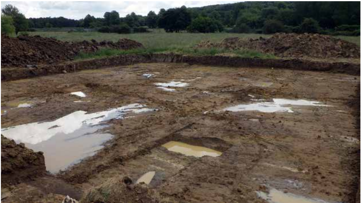
Plate 7: Trench 64 general view SE following rain
