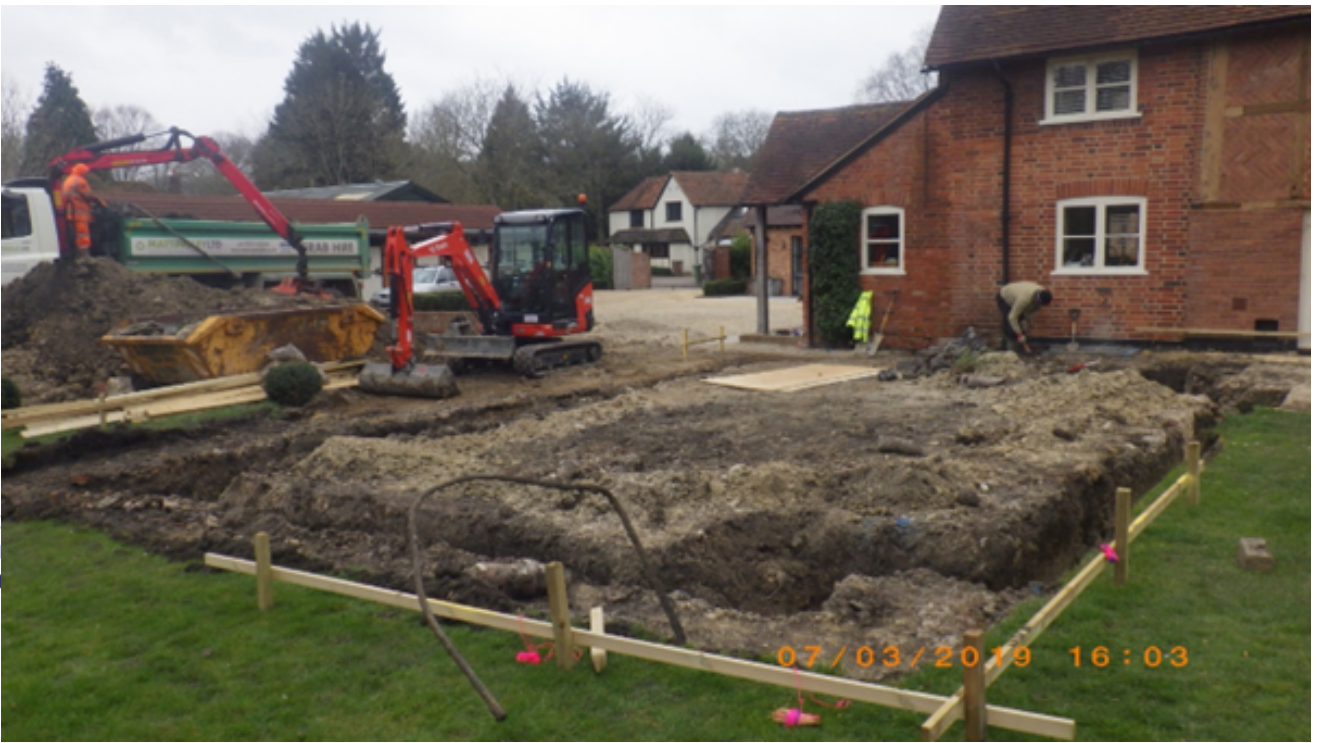
Plate 1: General shot works, view to west
