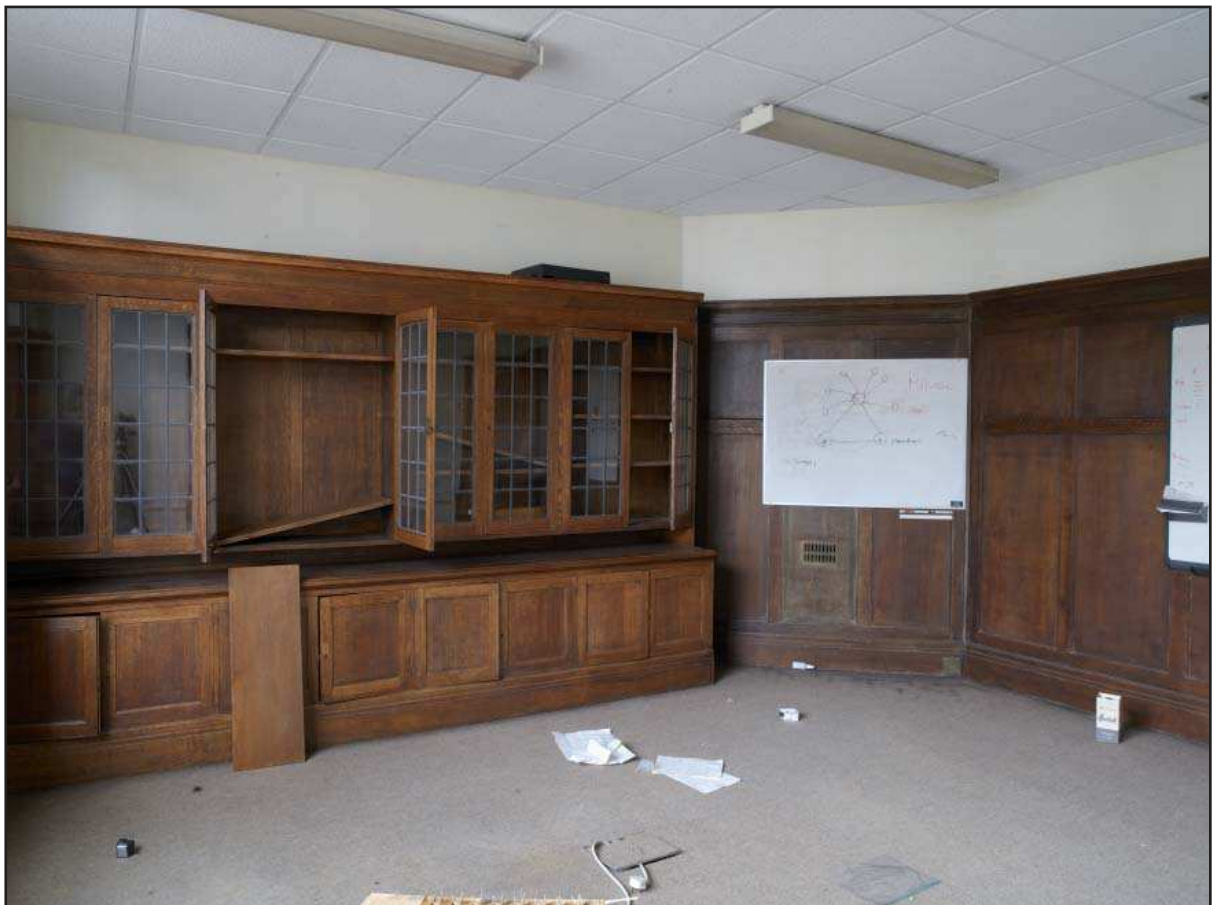
Plate 10: Office within Block B
