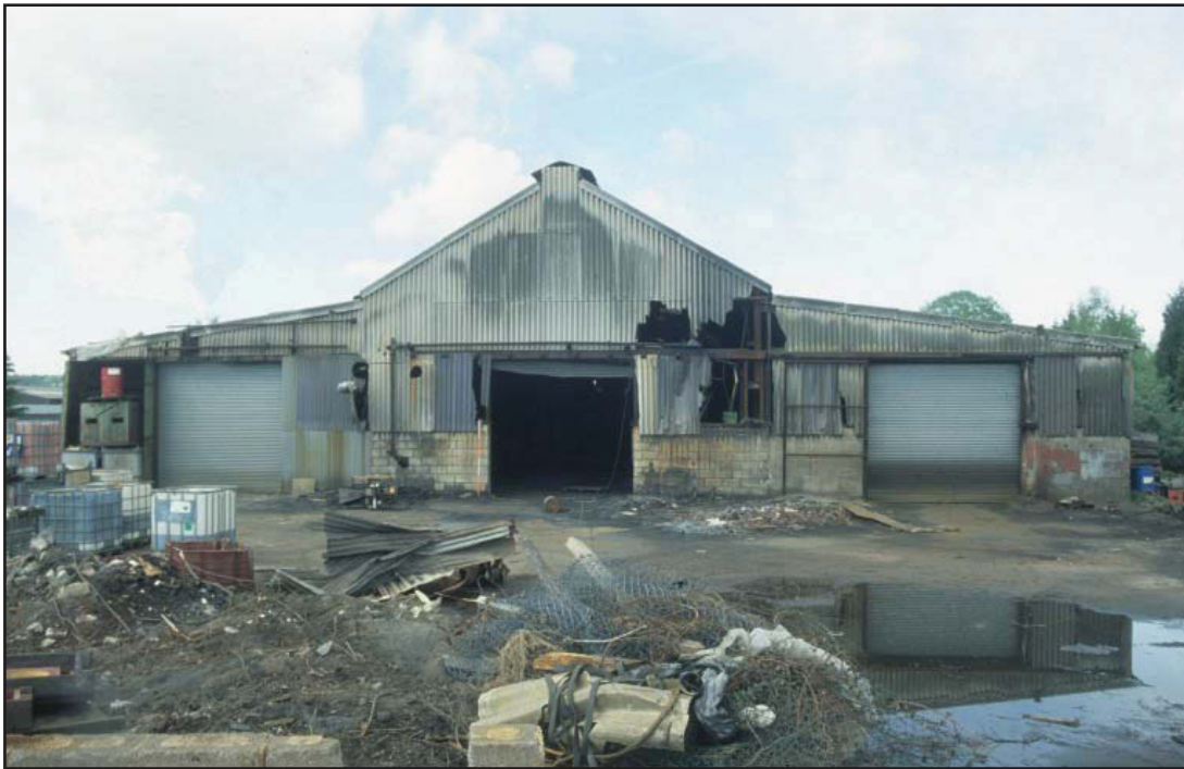
Plate 3: South end of foundry, showing extension 3, 4 and 5
