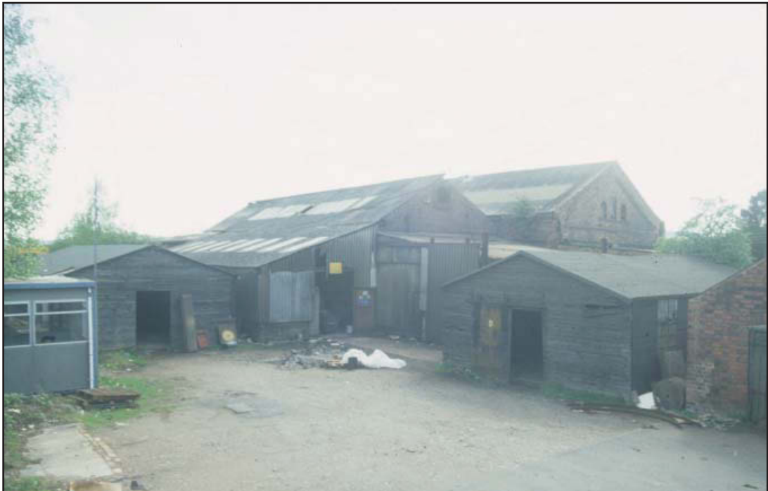
Plate 2: North end of foundry, showing buildings 1, 3, 5, 6 and 7
