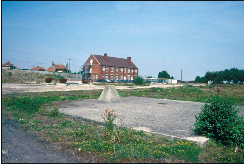
Plate 3: General view of the site from the south. Capped shaft in the foreground, main offices to the rear.
