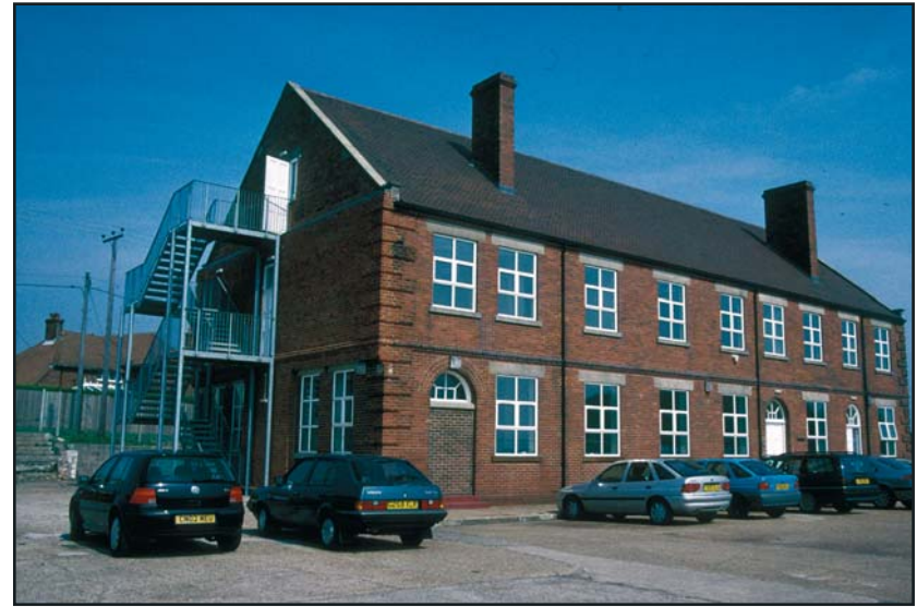
Plate 4: Main offices from the south
