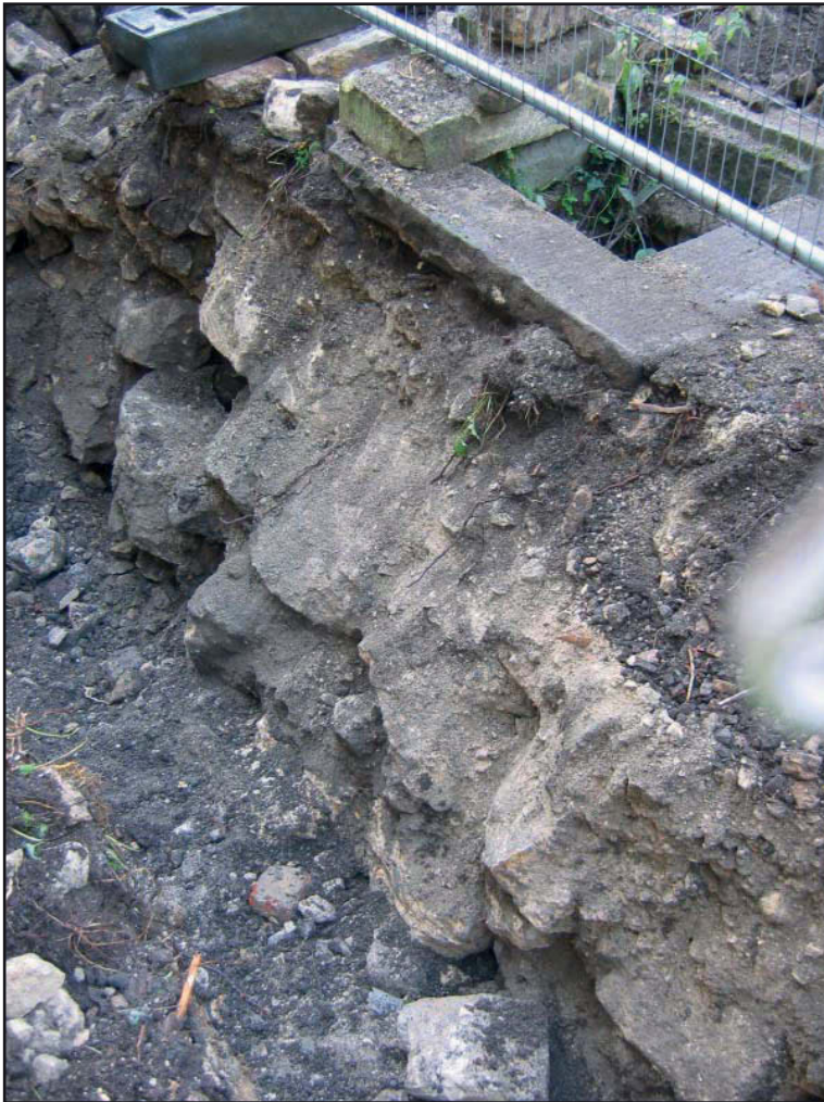
Plate 10: The west side of Trench 1b, showing the water tank's robbed (?) east side and the pennant framed manhole, 133
