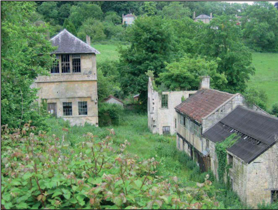
Plate 1: General view of mill from west with Building 2 to left rear and roofless Building 4 to right rear. The low range bottom right is Building 1, subject of a separate report
