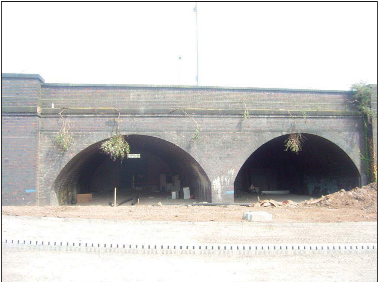
Plate 12 : Spans 10 & 11 View to North
