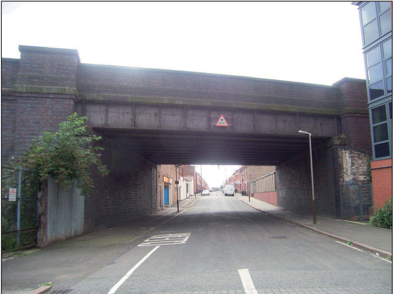
Plate 14 : Span 12 View to South
