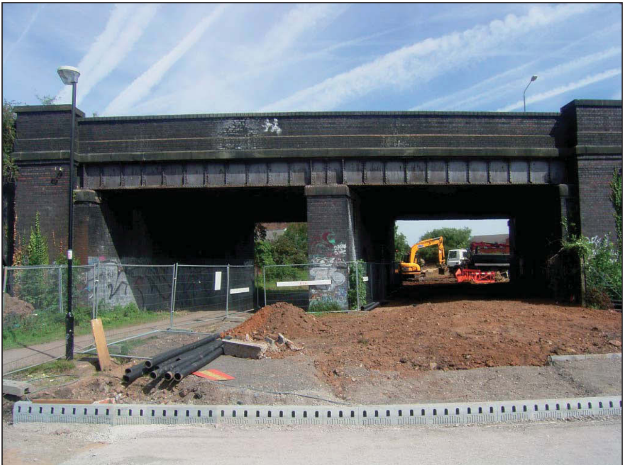
Plate 10 : Spans 8 & 9 View to North
