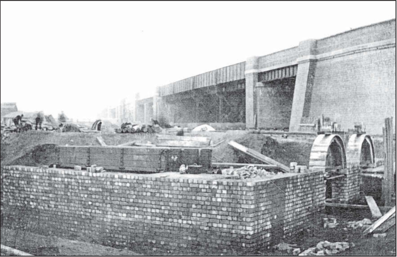
Plate 3 : Construction of Engine Shed View to NW c.1897-1903 by S.W.A. Newton
