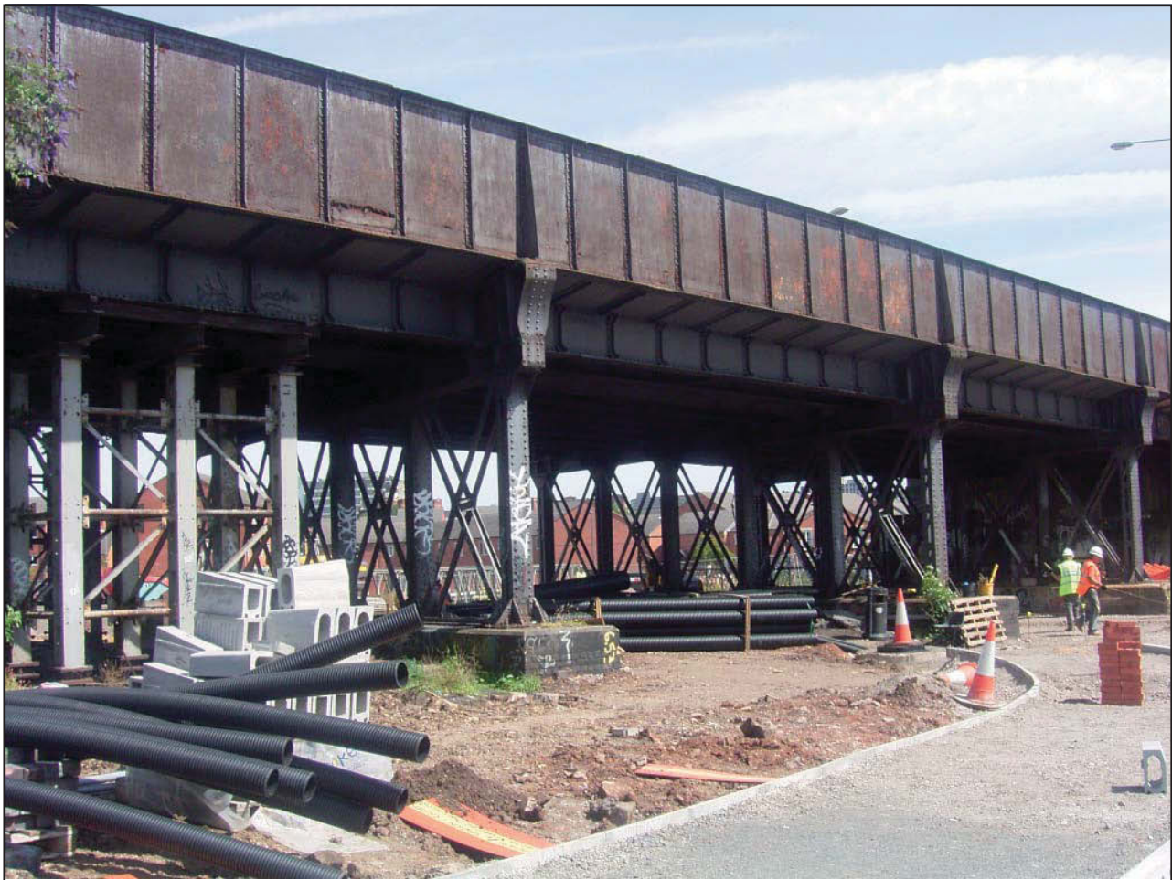
Plate 8 : Spans 4 to 7 View to North West
