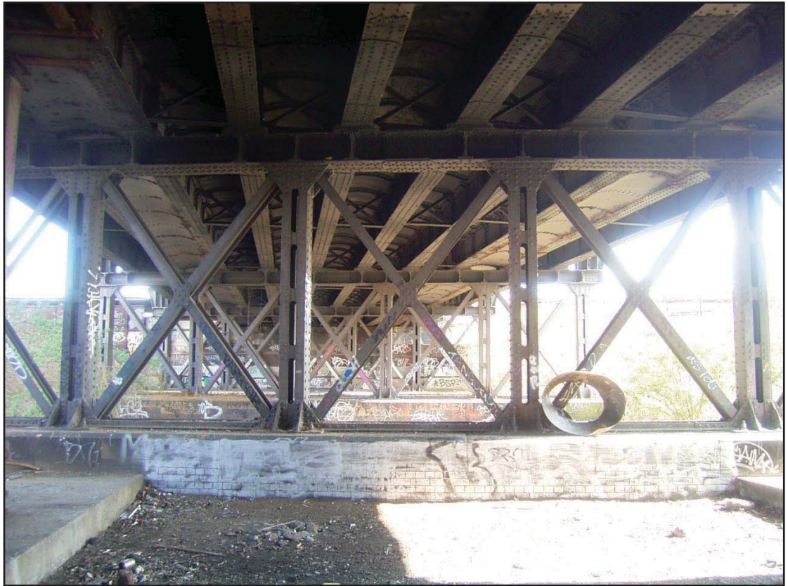
Plate 9 : Spans 4 to 7 Internal Structure
