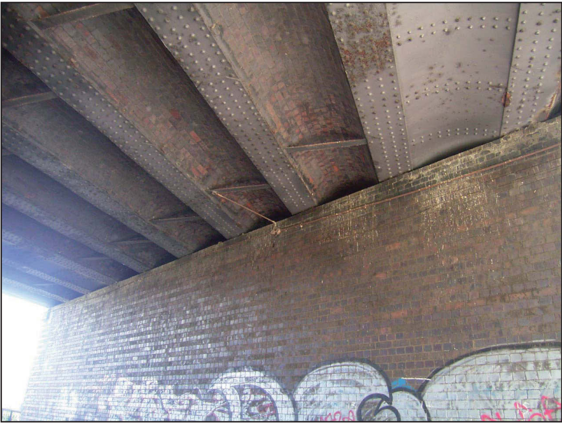
Plate 7 : Span 3 Showing Girders and Brick Jack Arches
