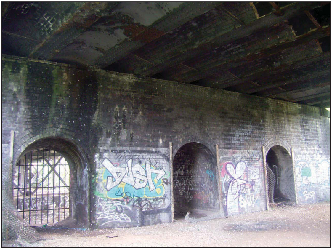
Plate 11 : Spans 8 & 9 Showing Safety Refuges
