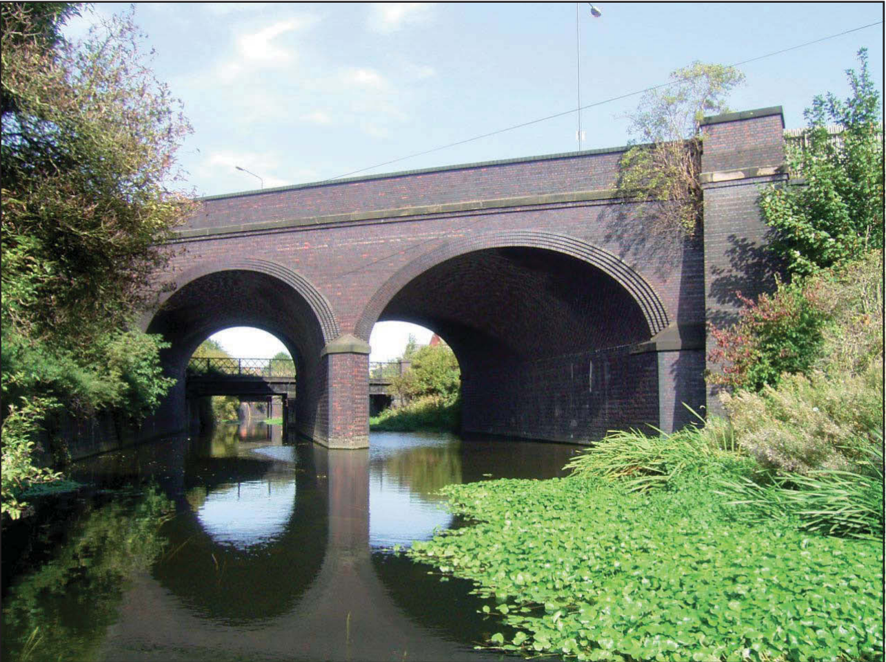
Plate 4 : Spans 1 & 2 View to North
