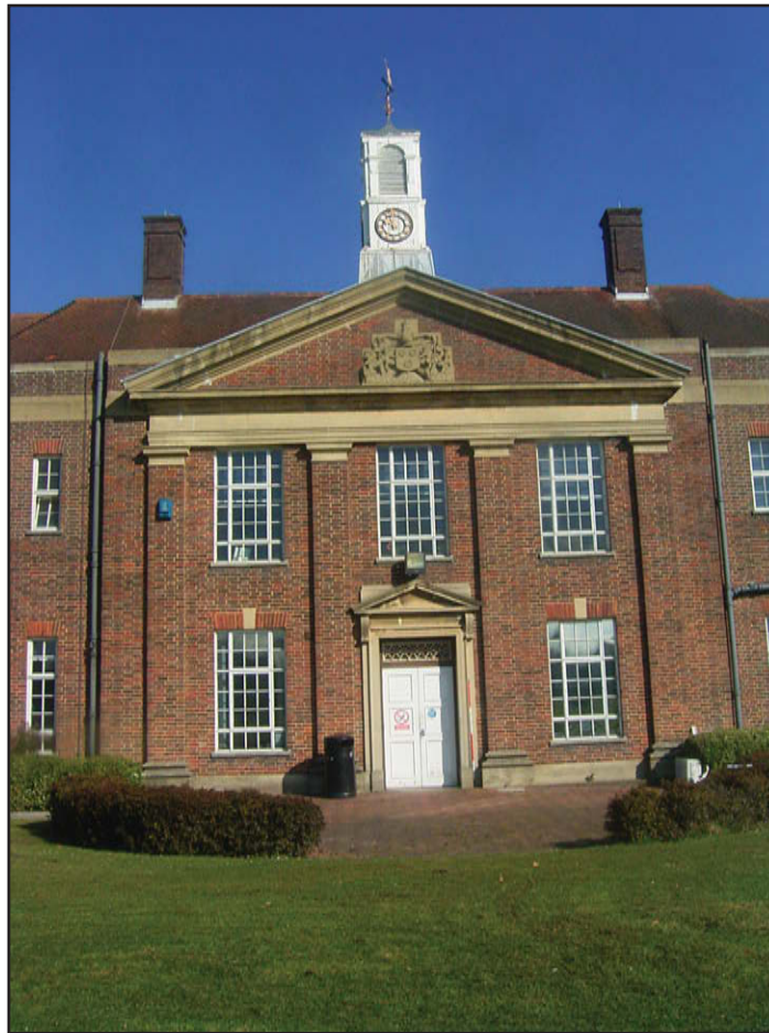
Plate 3: The central section of the south elevation
