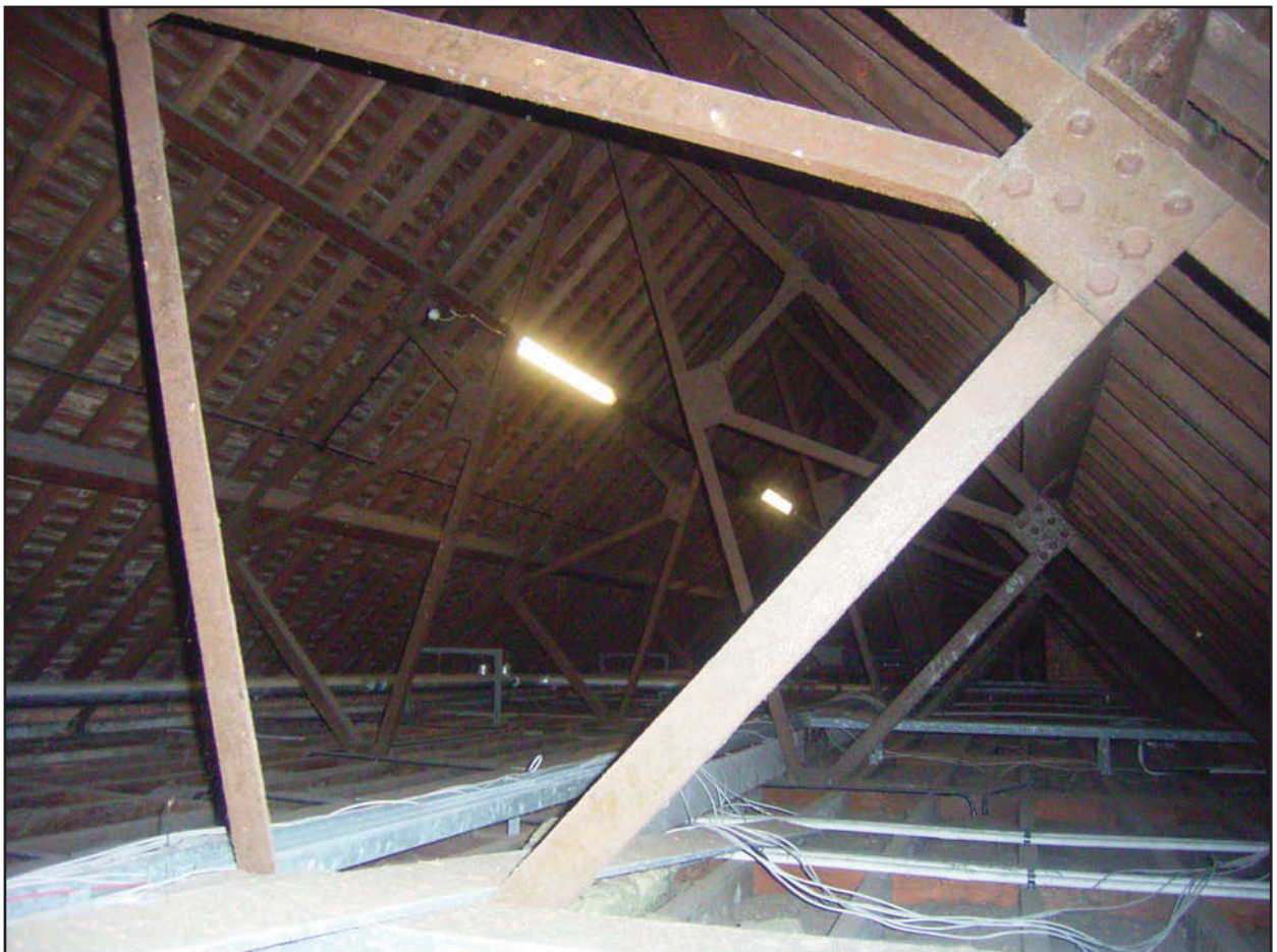
Plate 28: The 1936 south range roof trusses
