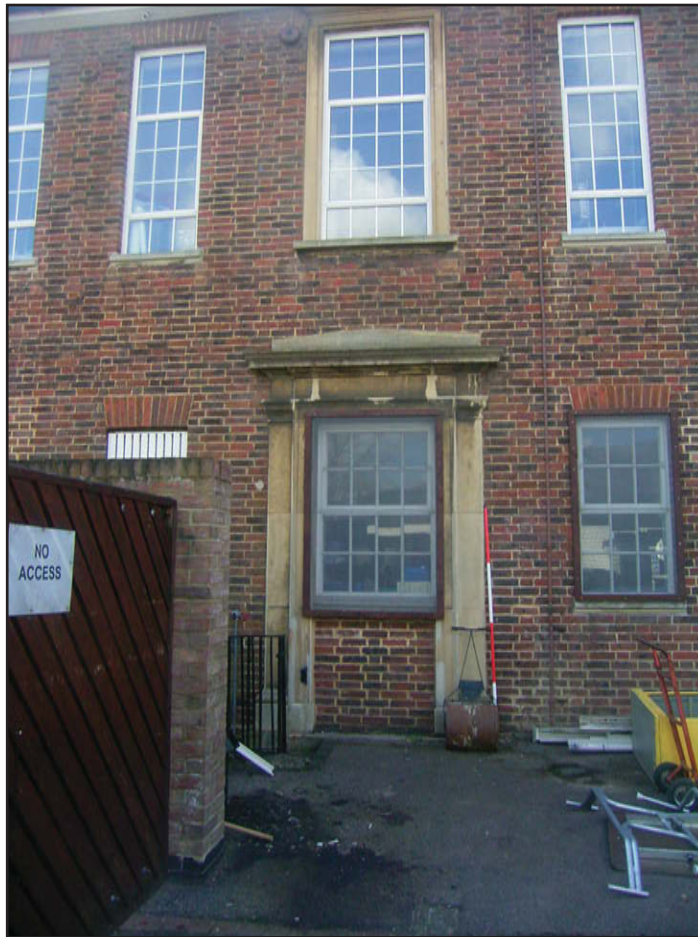
Plate 13: Blocked doorway in north elevation
