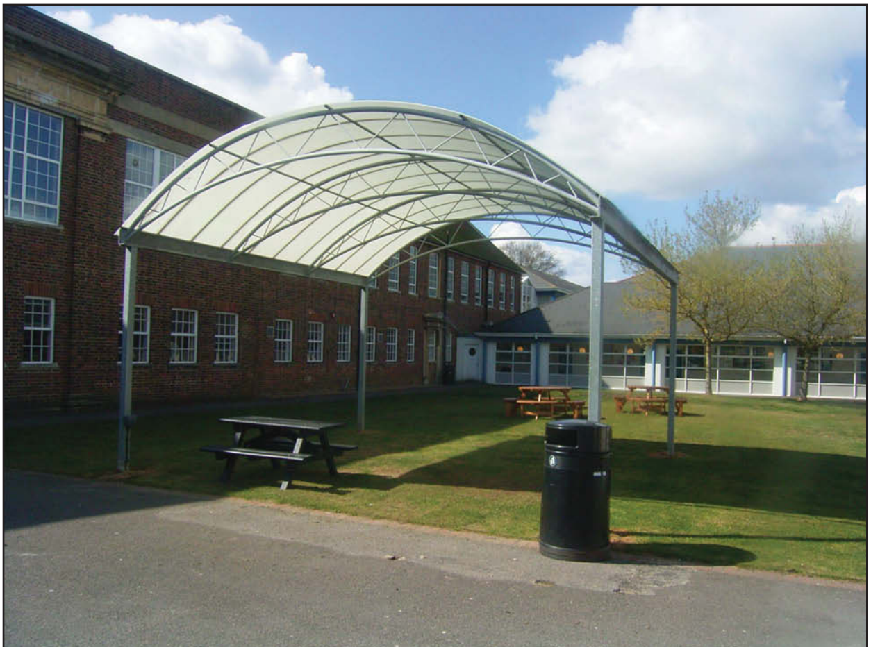
Plate 14: The north elevation
