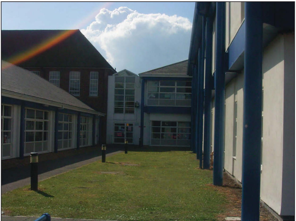
Plate 10: The corridor connecting the sports hall extension to the 1930s main building
