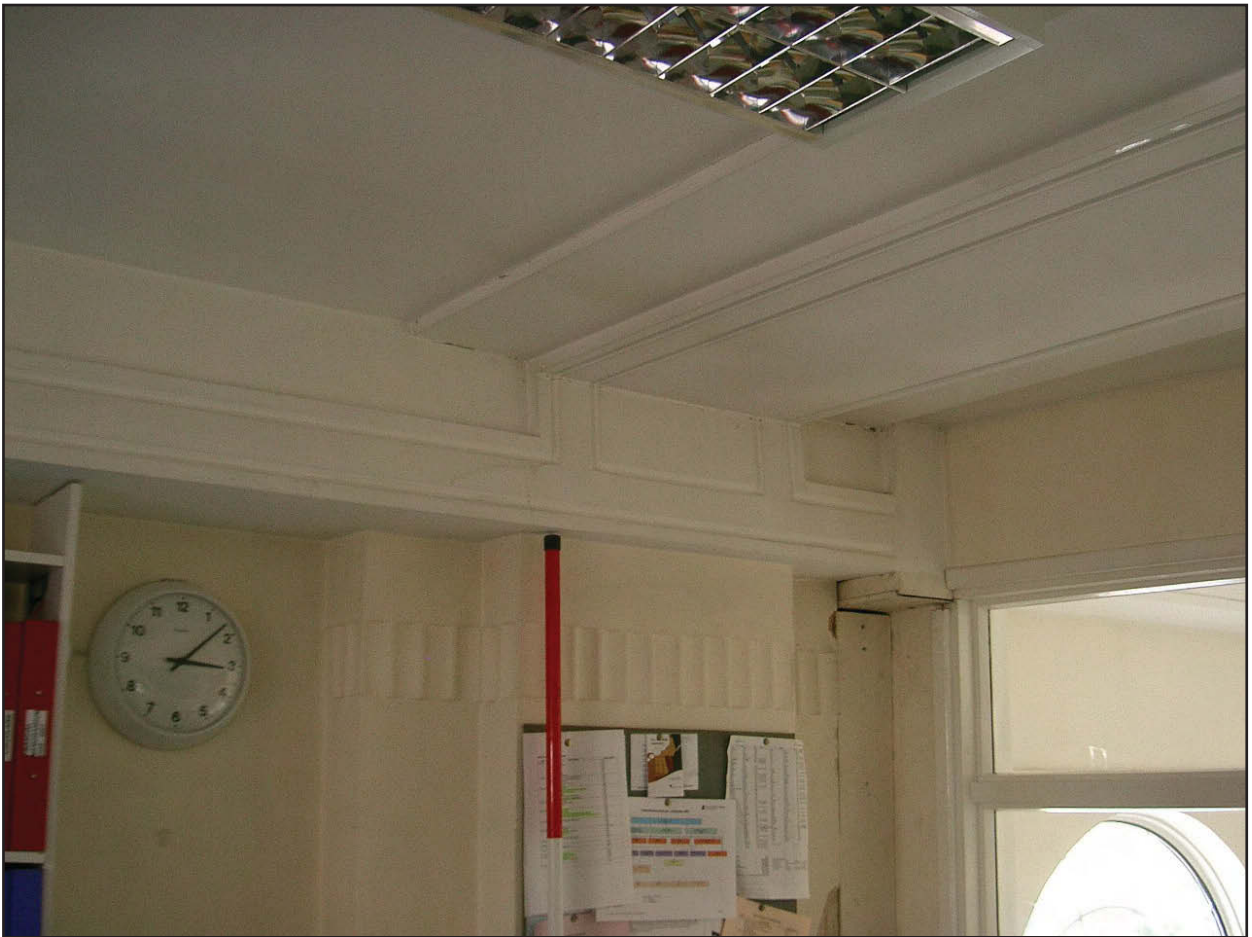
Plate 17: Detail from previous dining room as seen from within mezzanine offices
