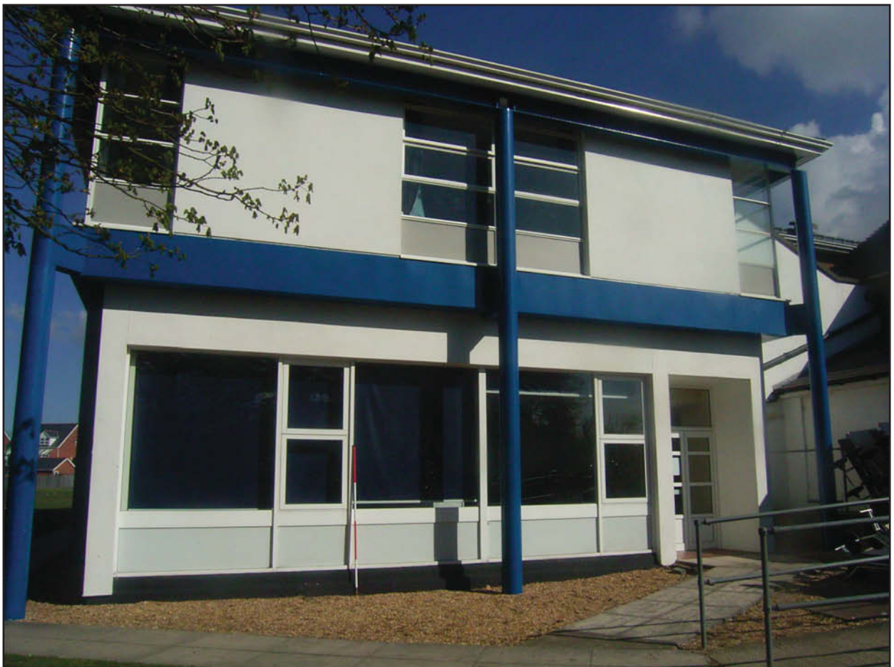
Plate 8: The 1991 sports hall extension east elevation
