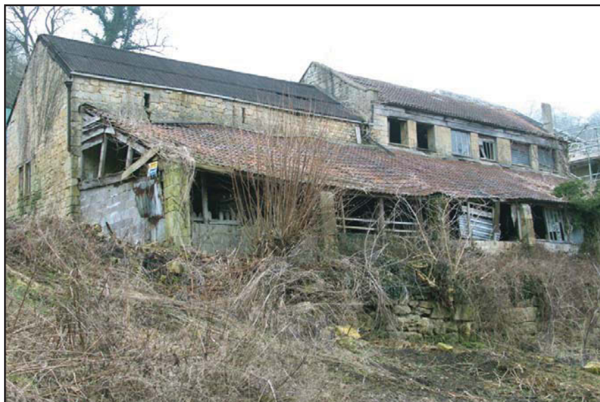
Plate 6: South elevation looking north-east.
