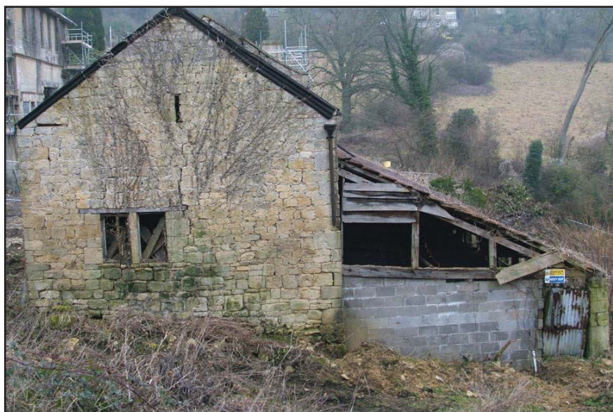
Plate 3: West end gable wall.
