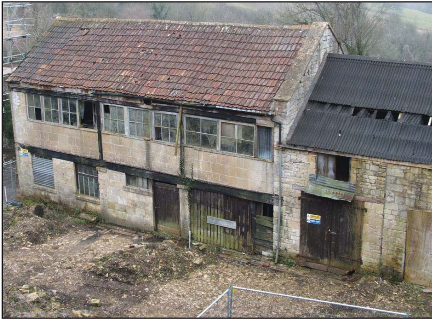
Plate 4: Phase 3 looking south east.
