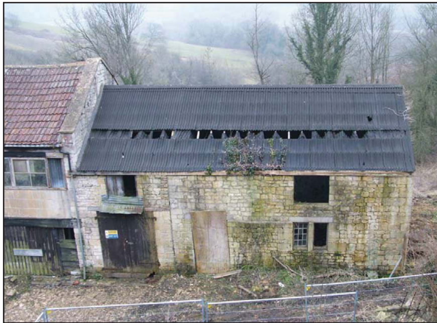
Plate 2: Phases 1 and 2 looking north, phase 1 on right.
