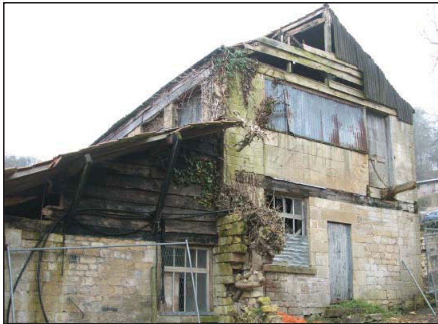
Plate 5: East end gable wall looking north-west.
