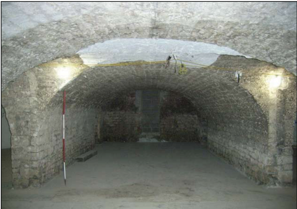
Plate 7: Octagon Vault Room 3 looking north-west
