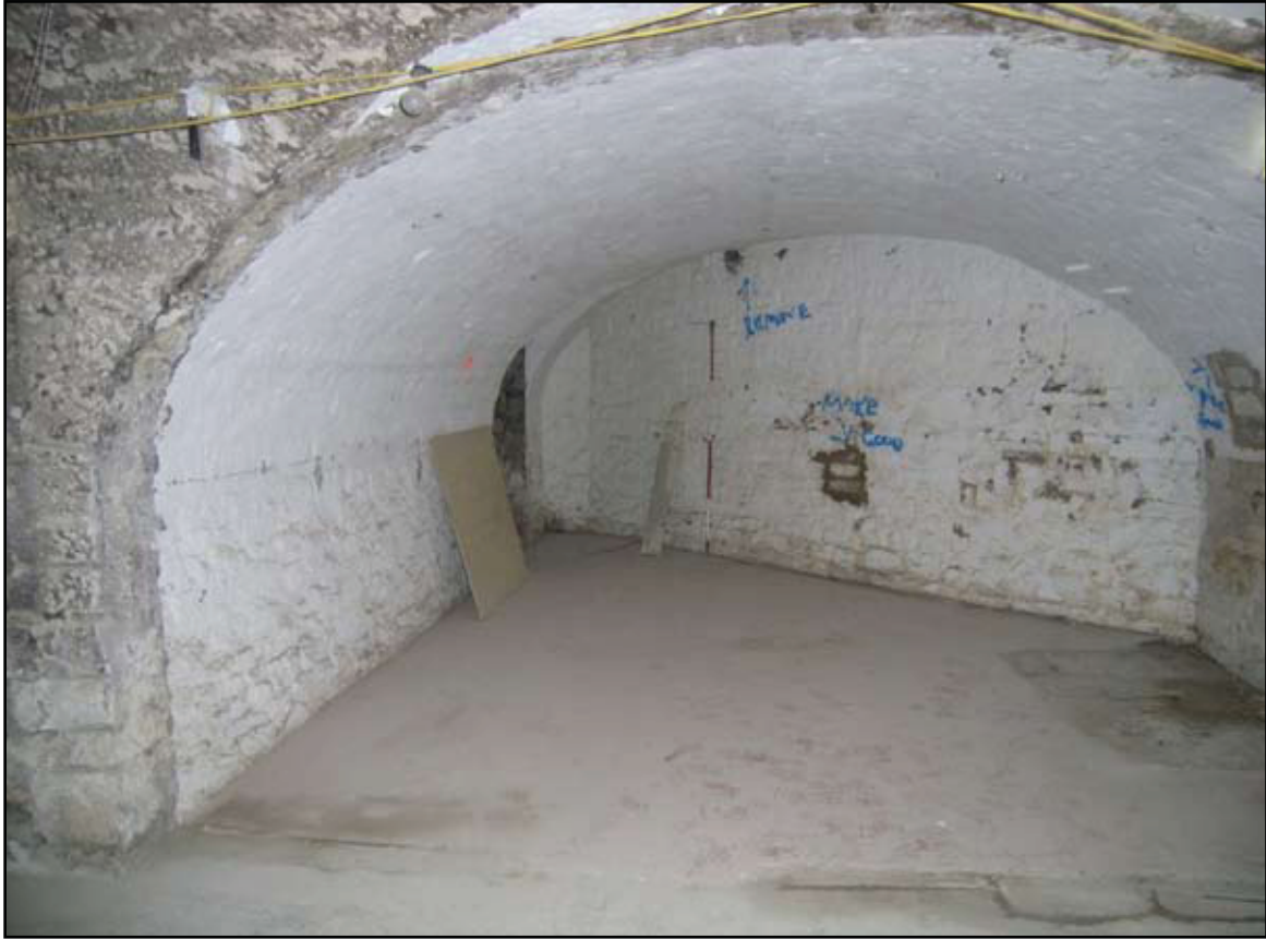
Plate 8: Octagon Vault Room 4 looking north-west
