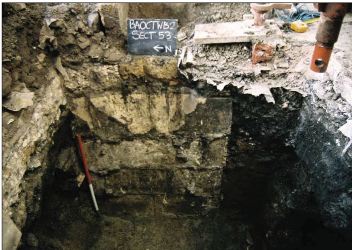
Plate 2: Trench 2 west facing Section 53 Wall (140)
