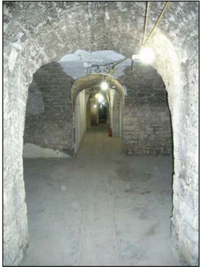
Plate 6: Octagon Vaults corridor and Tramway (123) looking towards Milsom Street
