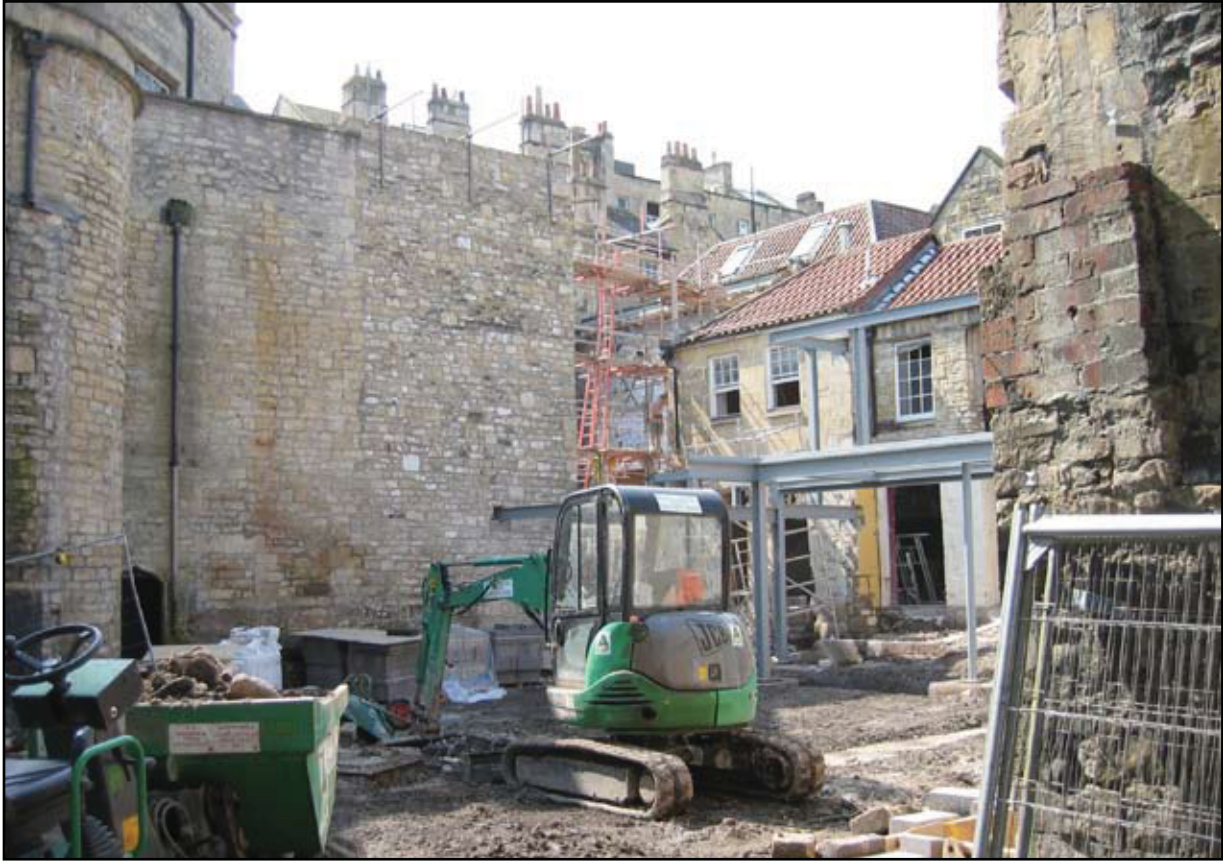
Plate 3: Western wall of Octagon Chapel and blocked Doorway (104) looking north-west
