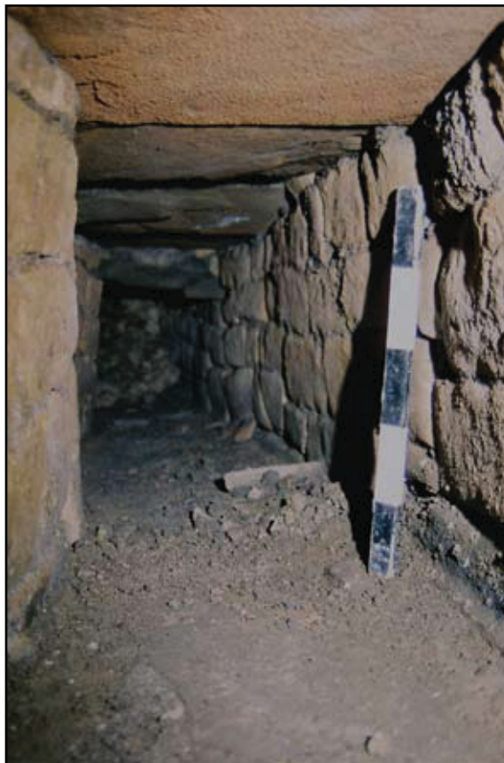
Plate 1: Trench 2 Culvert (151) looking south-east
