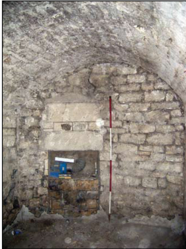
Plate 11: Octagon Vault Room 6 Blocked Fireplace (154)
