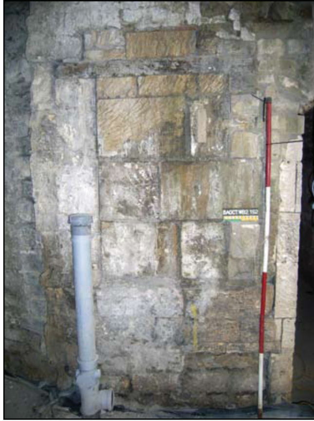
Plate 10: Octagon Vault Room 5 Blocked Window (152)
