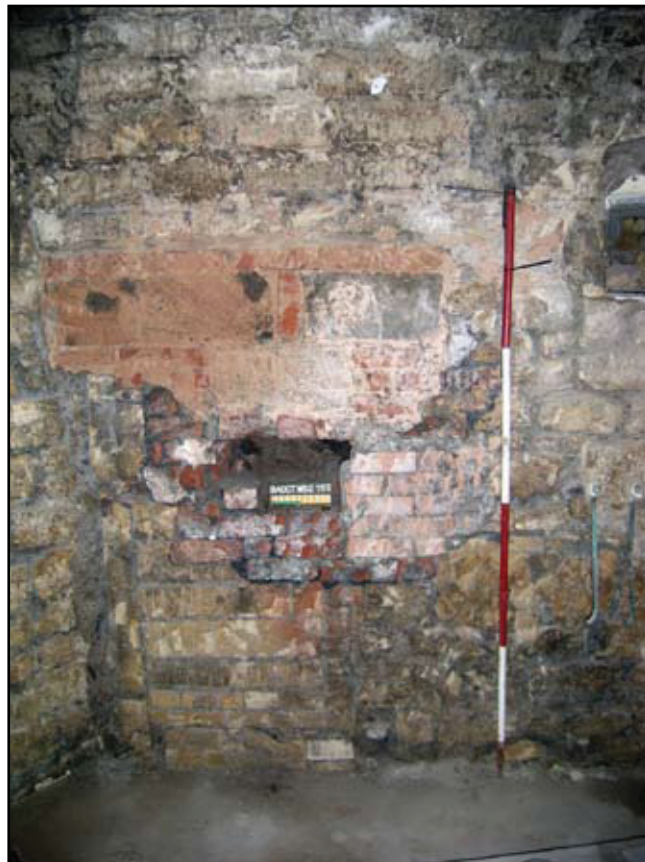
Plate 9: Octagon Vault Room 5 Blocked Fireplace (155)
