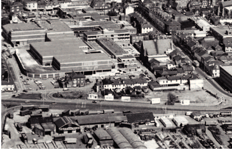
Plate 1: Aerial photograph of Godington Road and Hampstead Street (1975)
