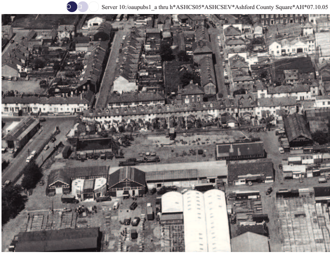
Plate 2: Aerial photograph of Godington Road and Hampstead Street (1963)
