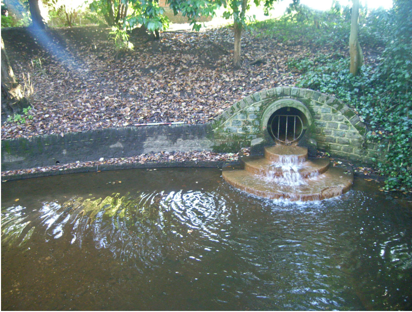
Plate 1: Southern lake inlet and wall
