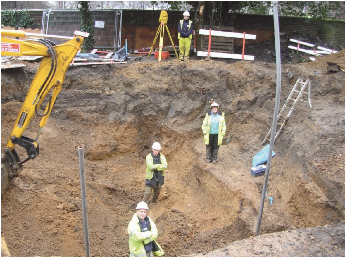
Plate 8: Trench showing depth of excavation
