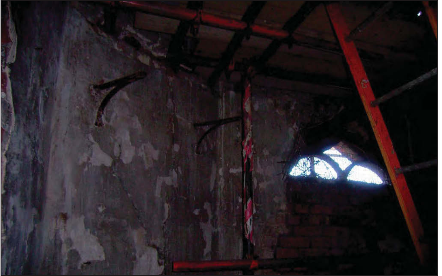
Plate 25: 1st floor of Dovecote
