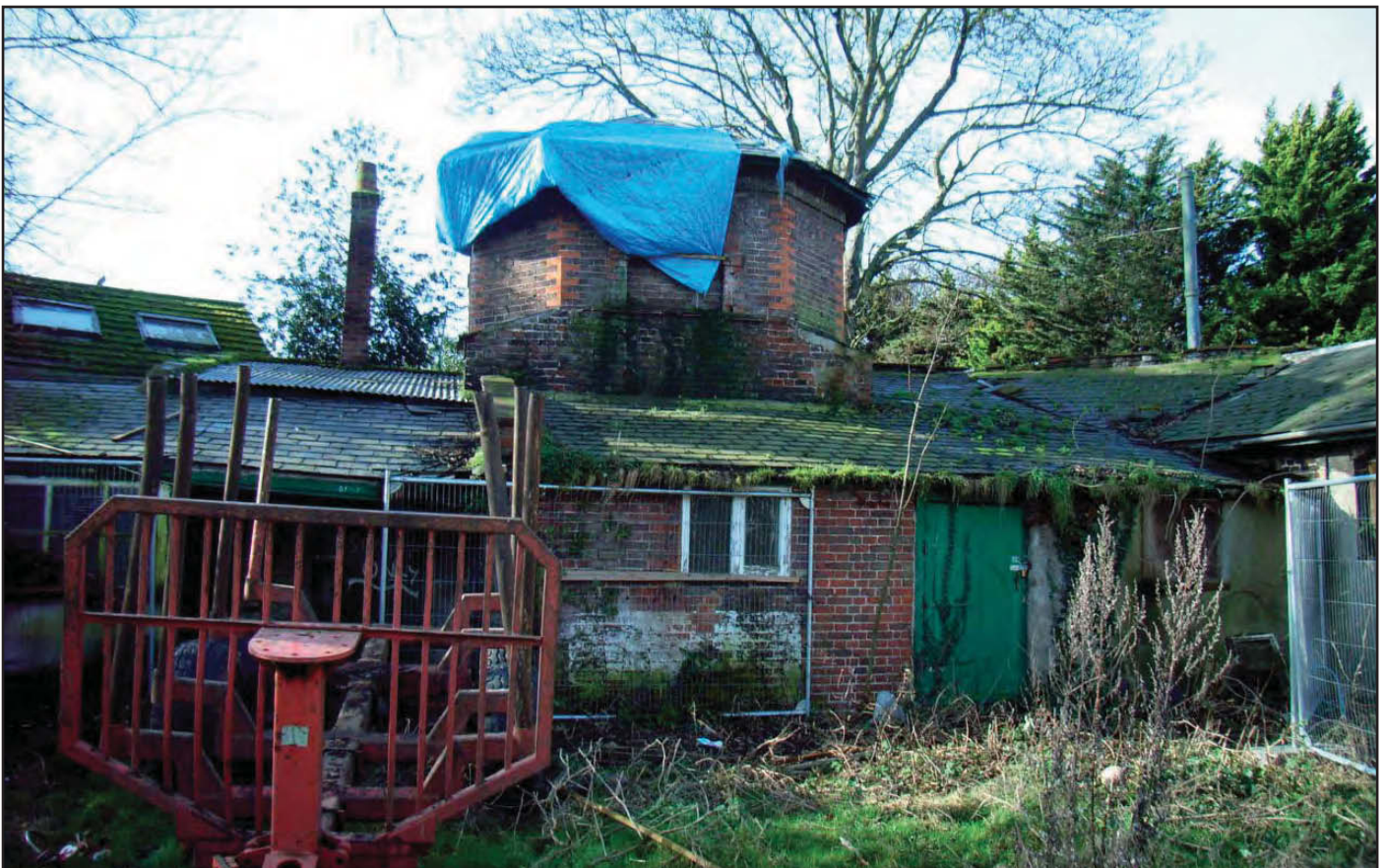
Plate 10: NE view of Dovecote before start of works
