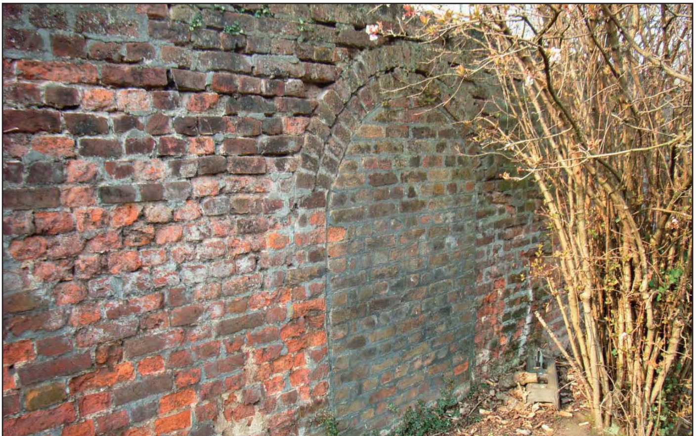
Plate 6: Infilled doorway in Wall 4
