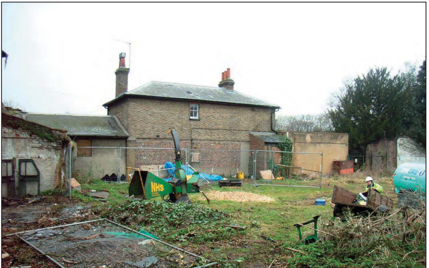
Plate 32: General view towards cottage before start of works
