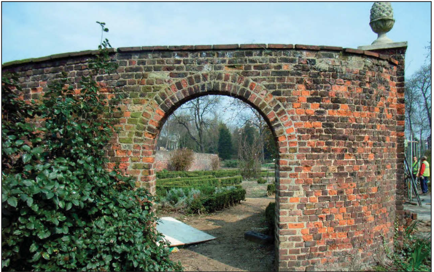
Plate 7: Secondary (early 20th century) doorway at corner between Walls 4 and 5
