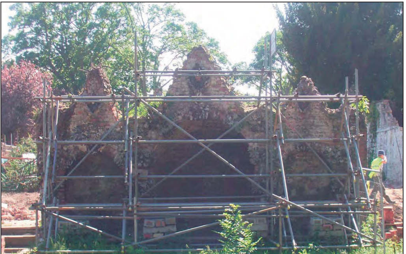
Plate 40: Alcove Seat from NE before start of works
