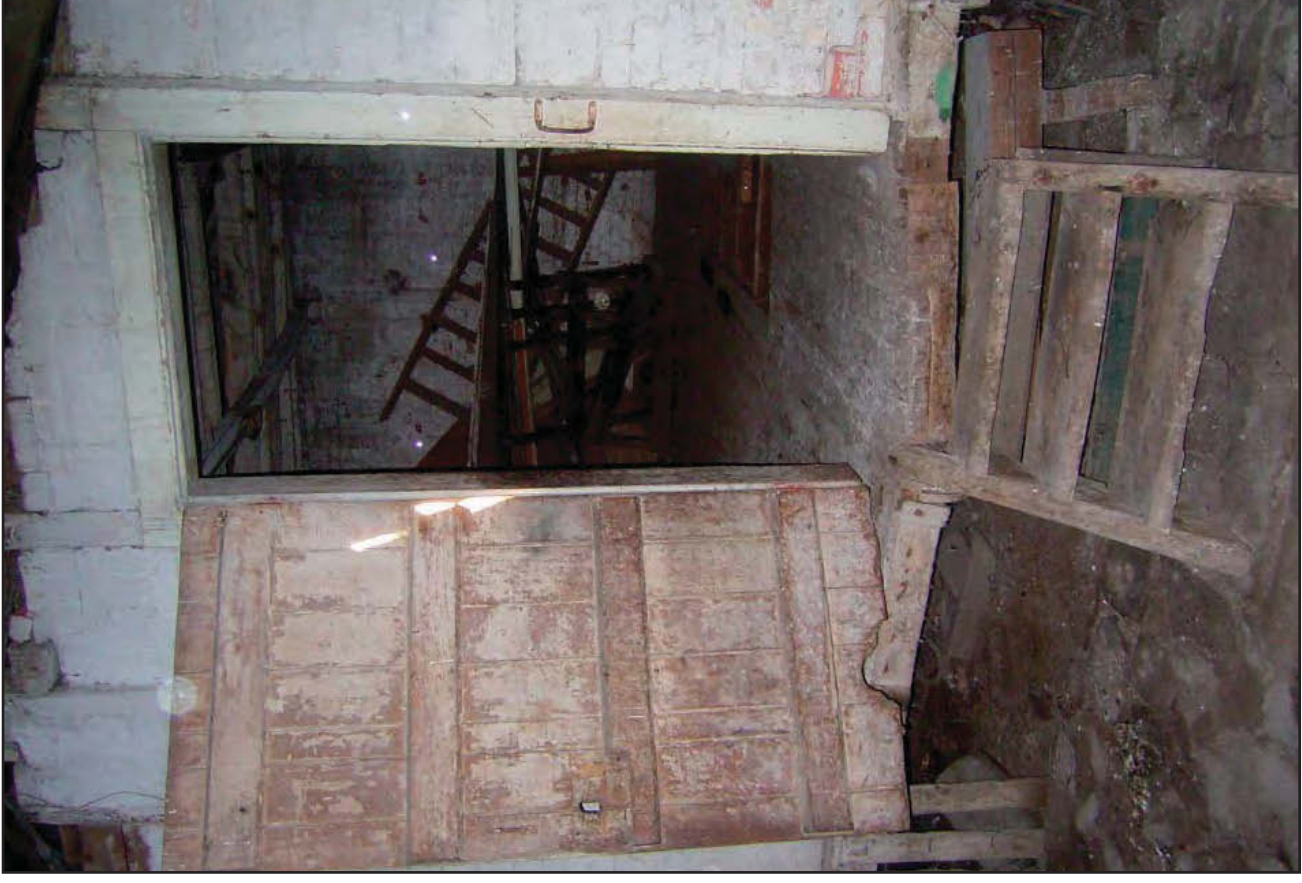
Plate 36: Access door to Granary
