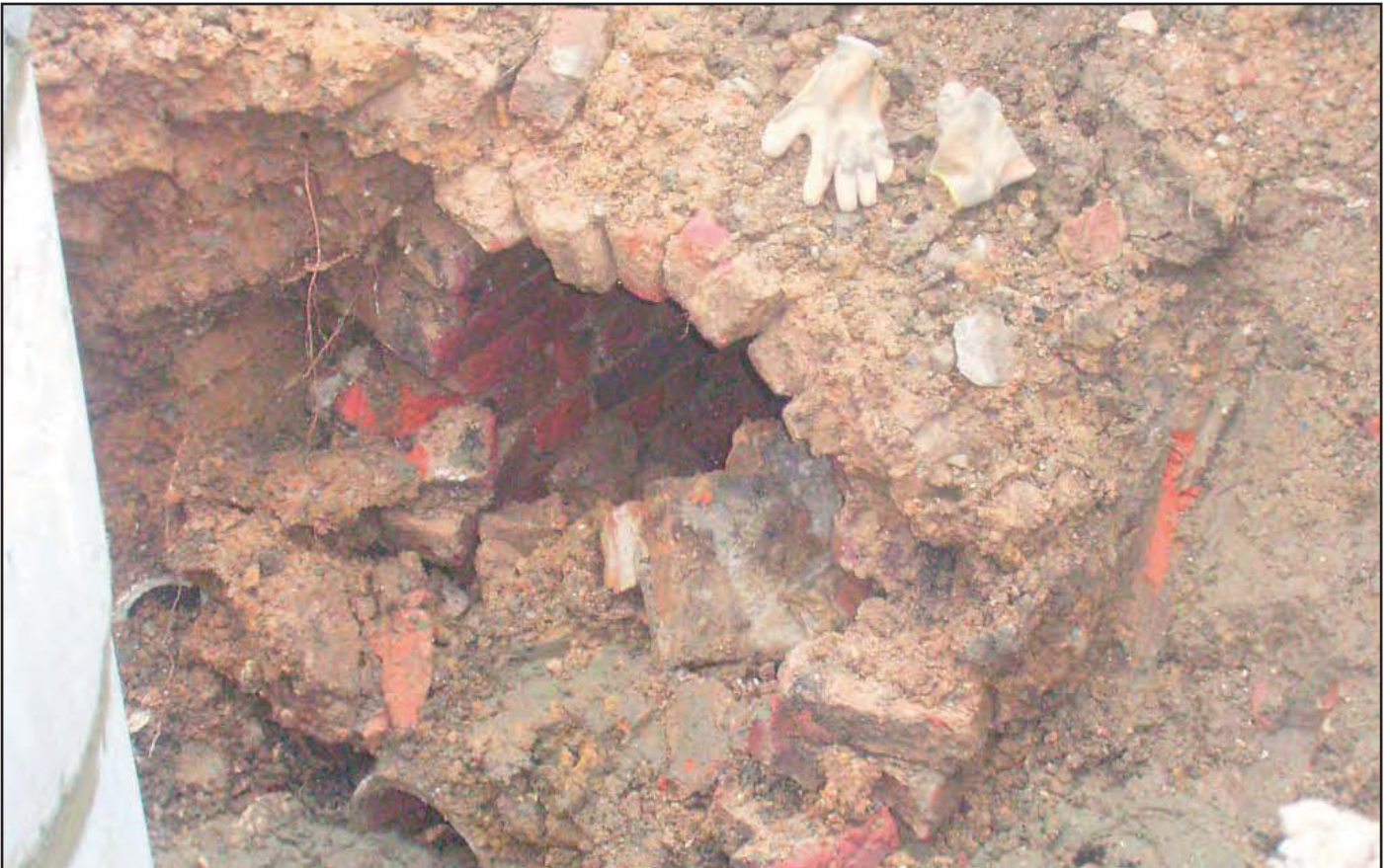
Plate 52: Culvert (5035) in Trench 33 adjacent to house
