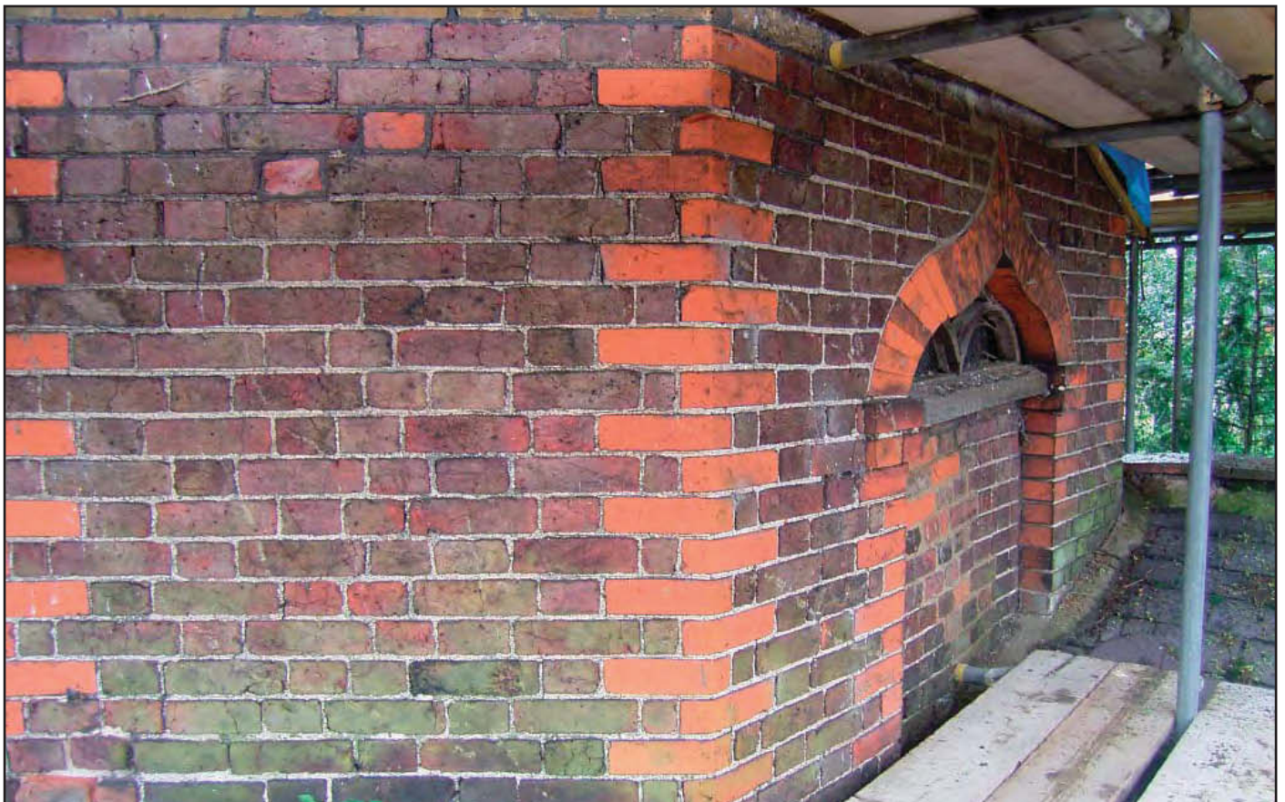
Plate 16: 1st floor of Dovecote
