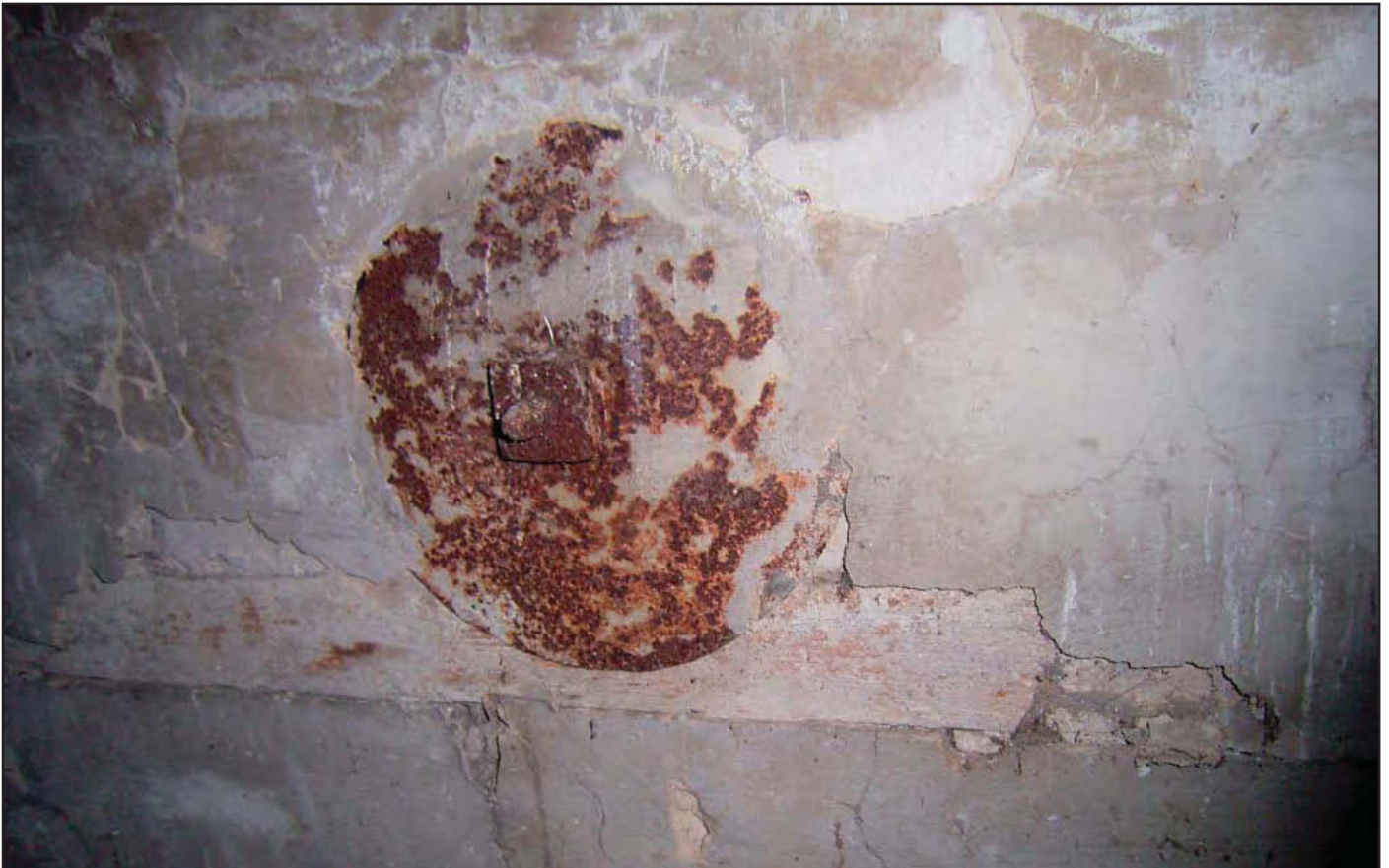
Plate 22: Tie bar plate in Dovecote
