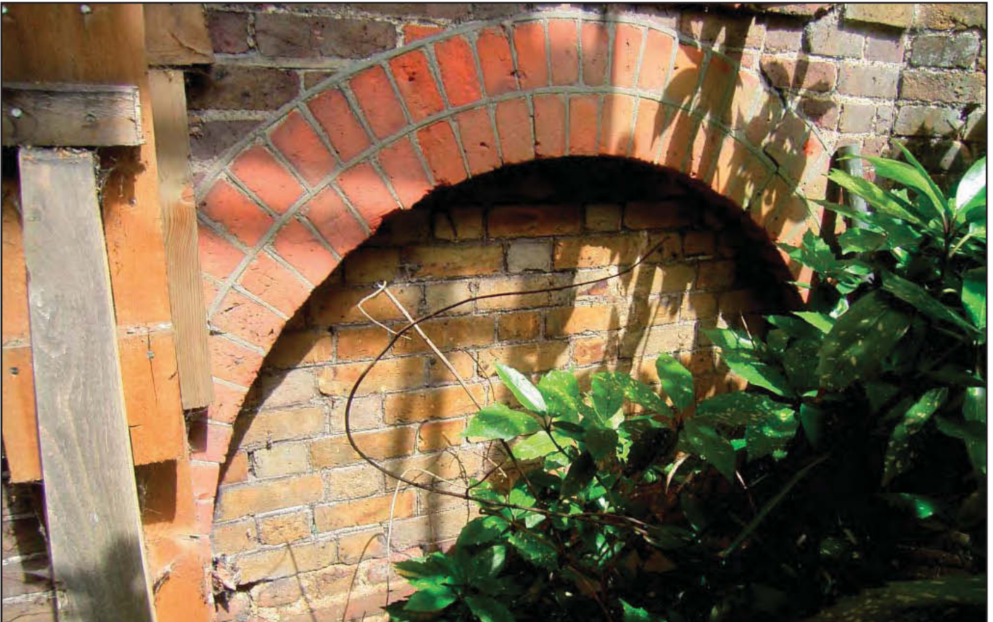
Plate 14: Blocked arch in SW elevation of Dovecote
