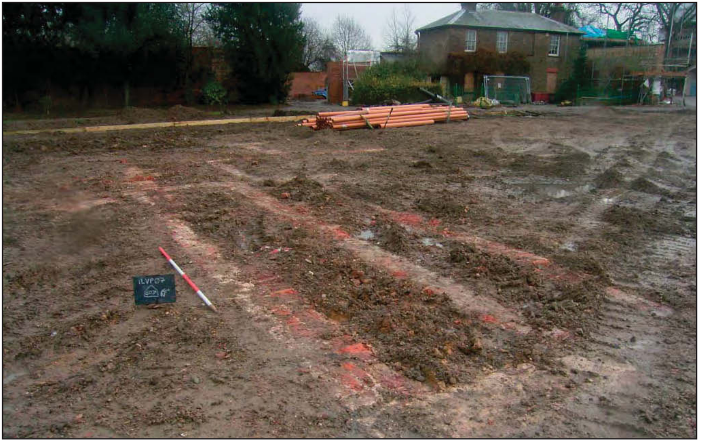
Plate 53: Footings (5034) exposed in Tennis Court Area viewed from north
