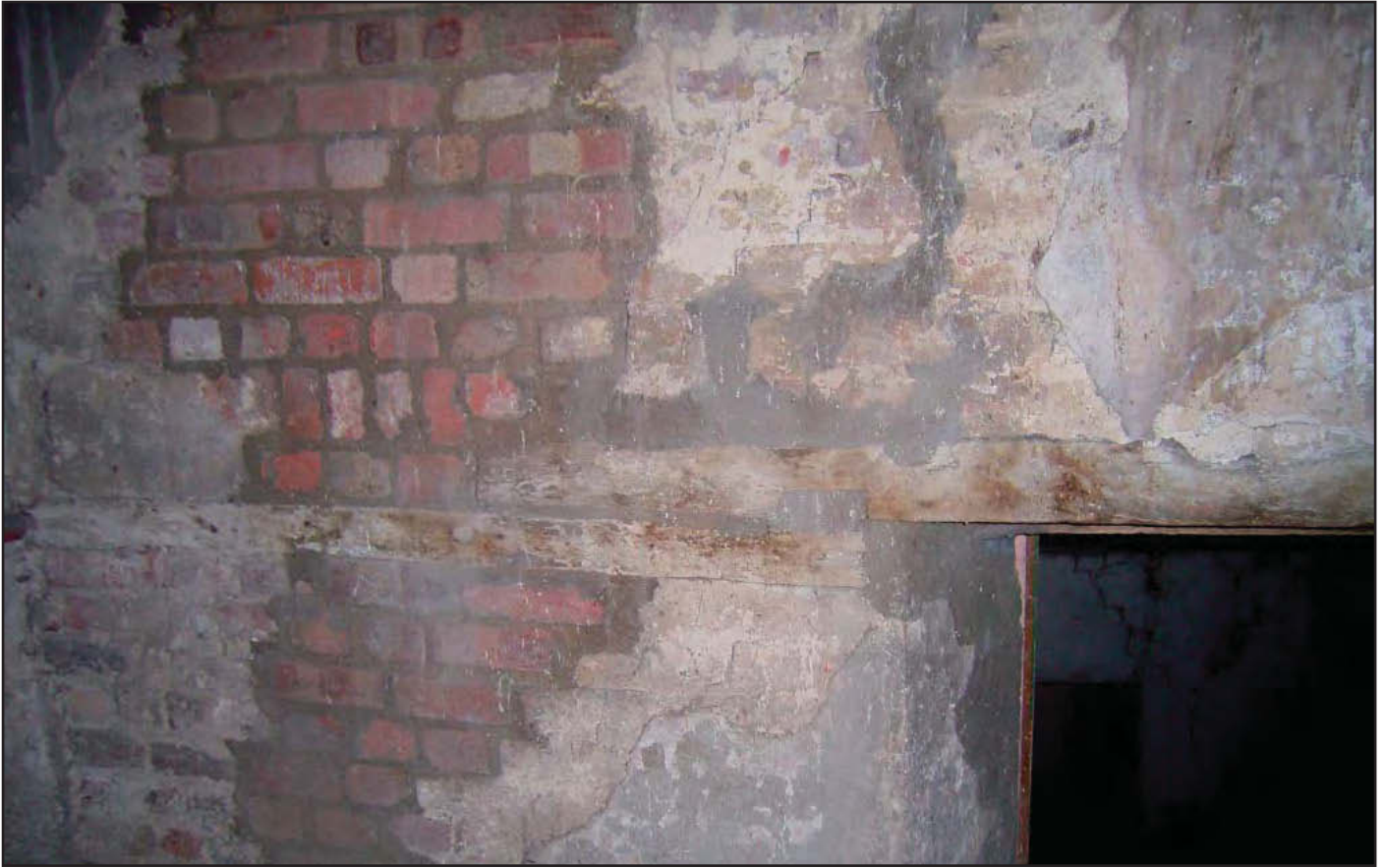
Plate 29: Repairs in internal walls of Dovecote
