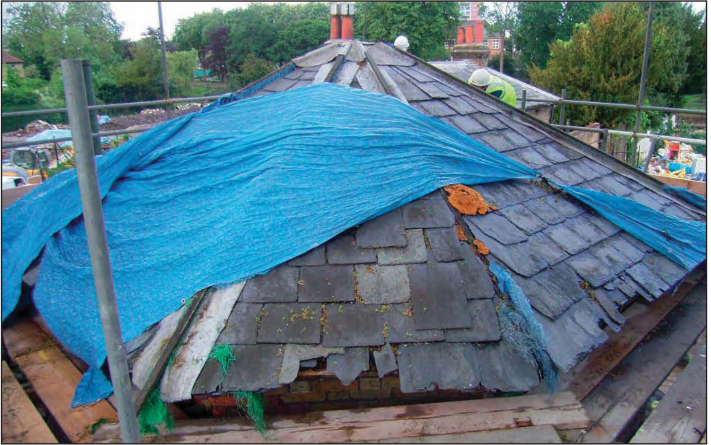
Plate 17: Roof of Dovecote
