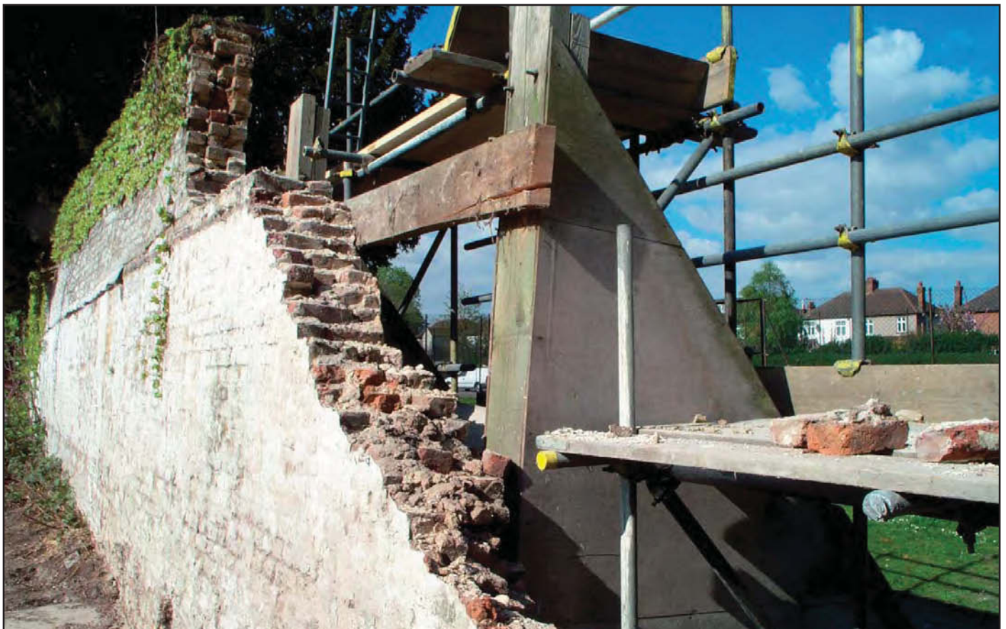
Plate 8: Wall 1 (NE end) during reconstruction
