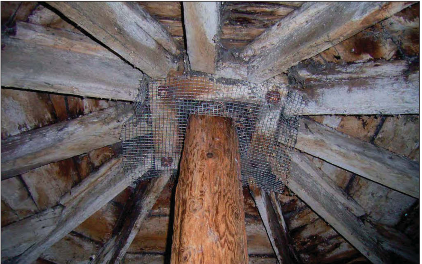
Plate 28: Apex of roof in Dovecote
