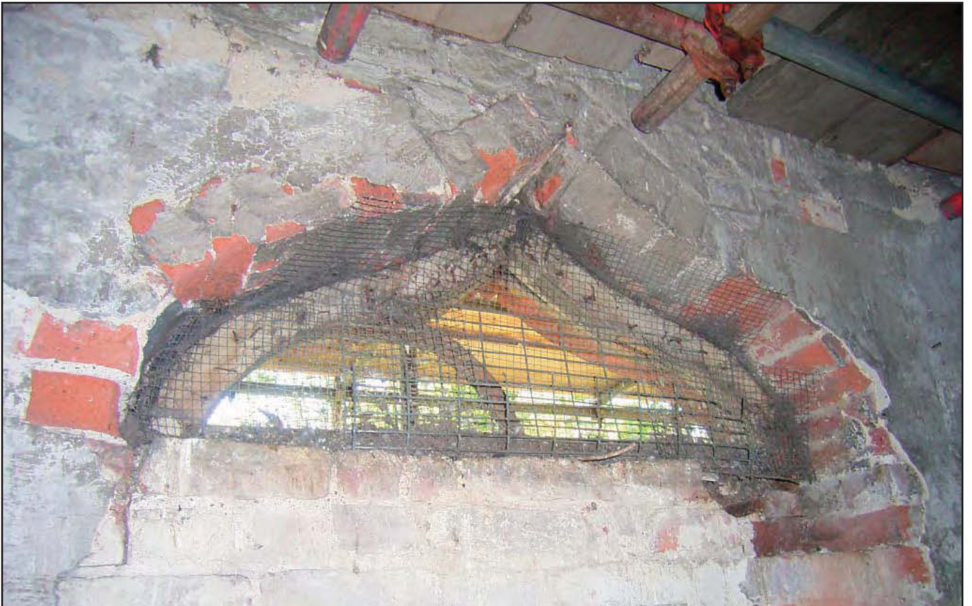
Plate 26: Window arch in Dovecote
