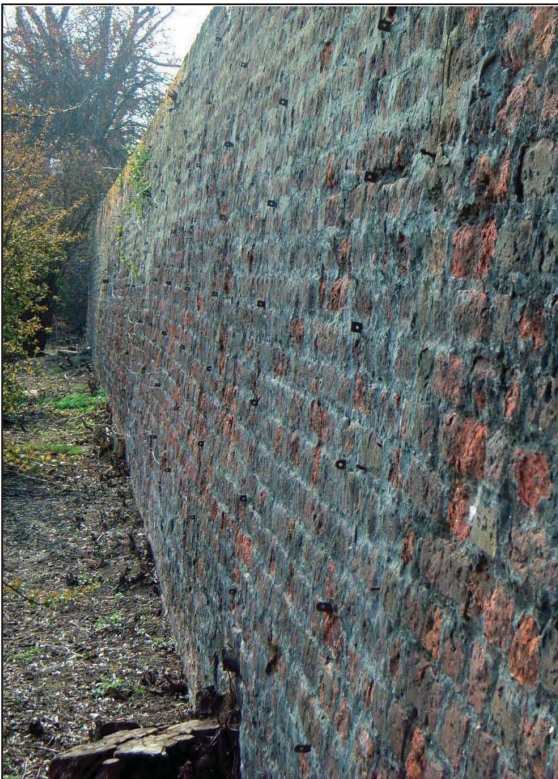
Plate 4: SE side of Wall 2 showing ash-rich repointing
