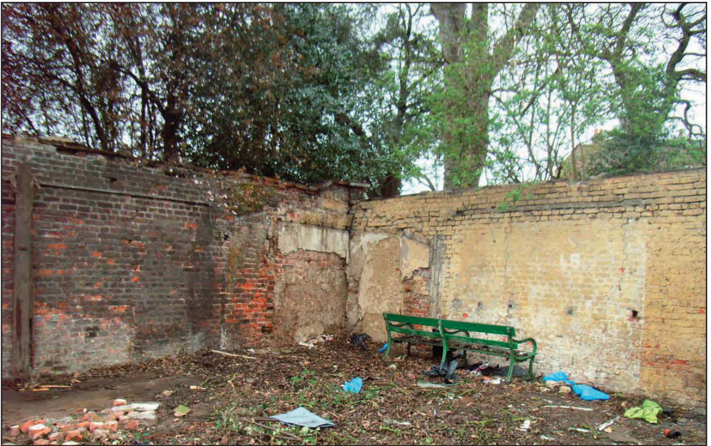
Plate 3: South corner between Walls 2a and 3
