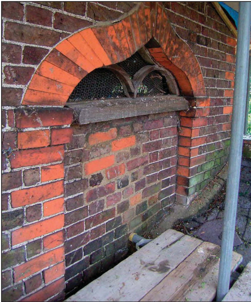
Plate 15: 1st floor blind window in Dovecote with 1864 inscribed on brick
