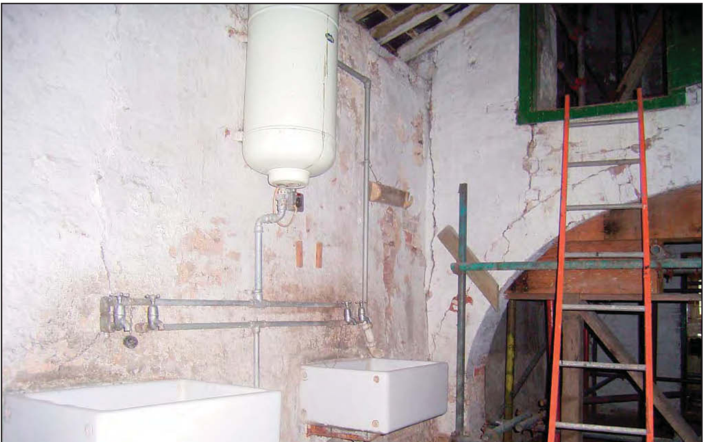
Plate 24: NW ground floor room in Dovecote
