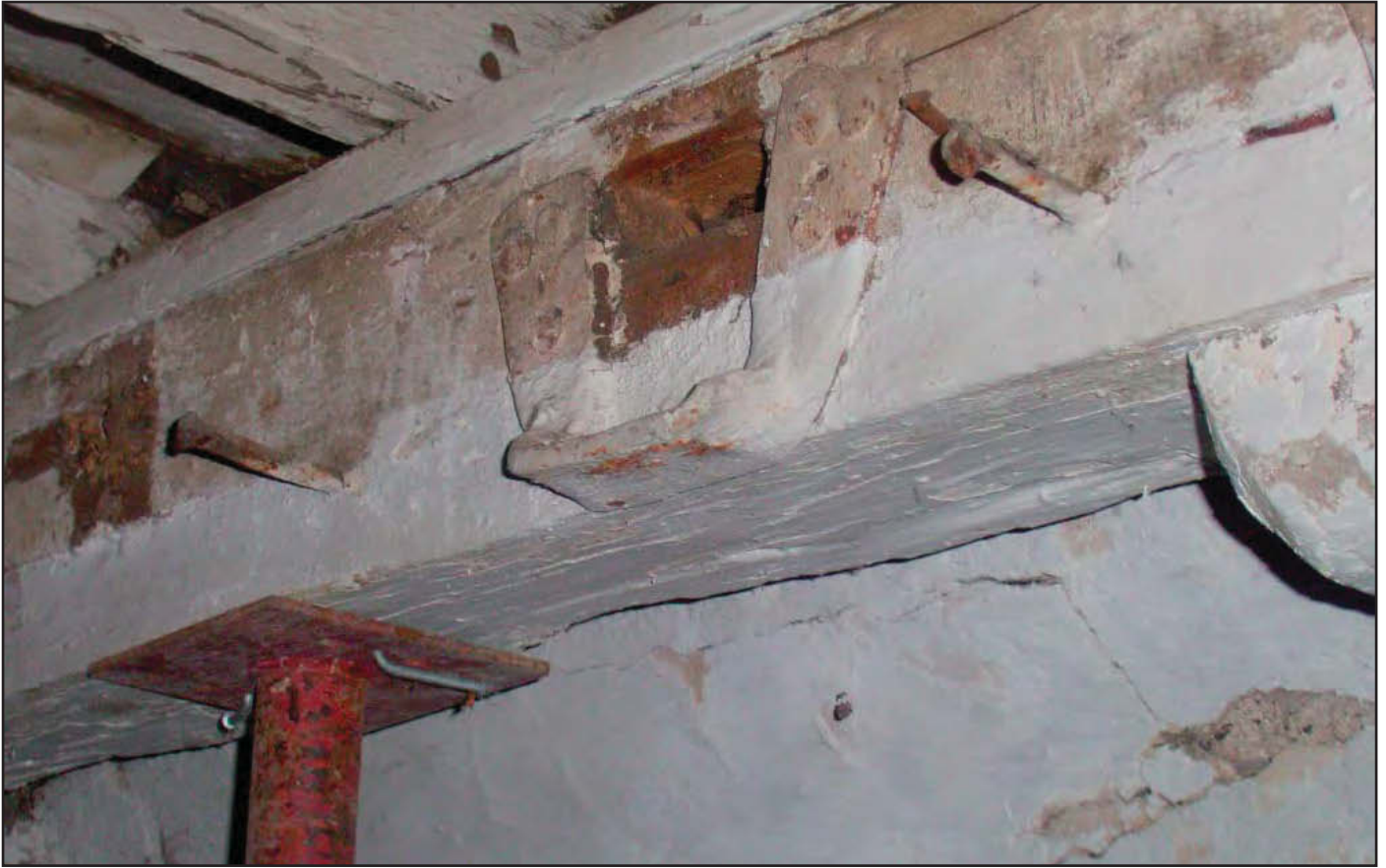
Plate 21: Sockets in principal joist of Dovecote central room
