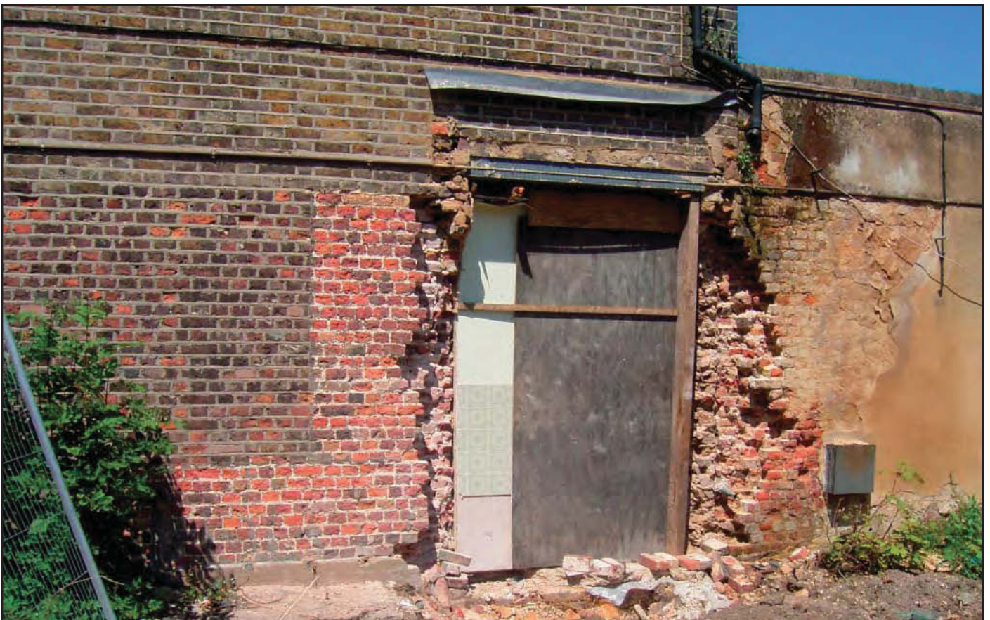
Plate 34: SE wall of Cottage after removal of WC lean-to
