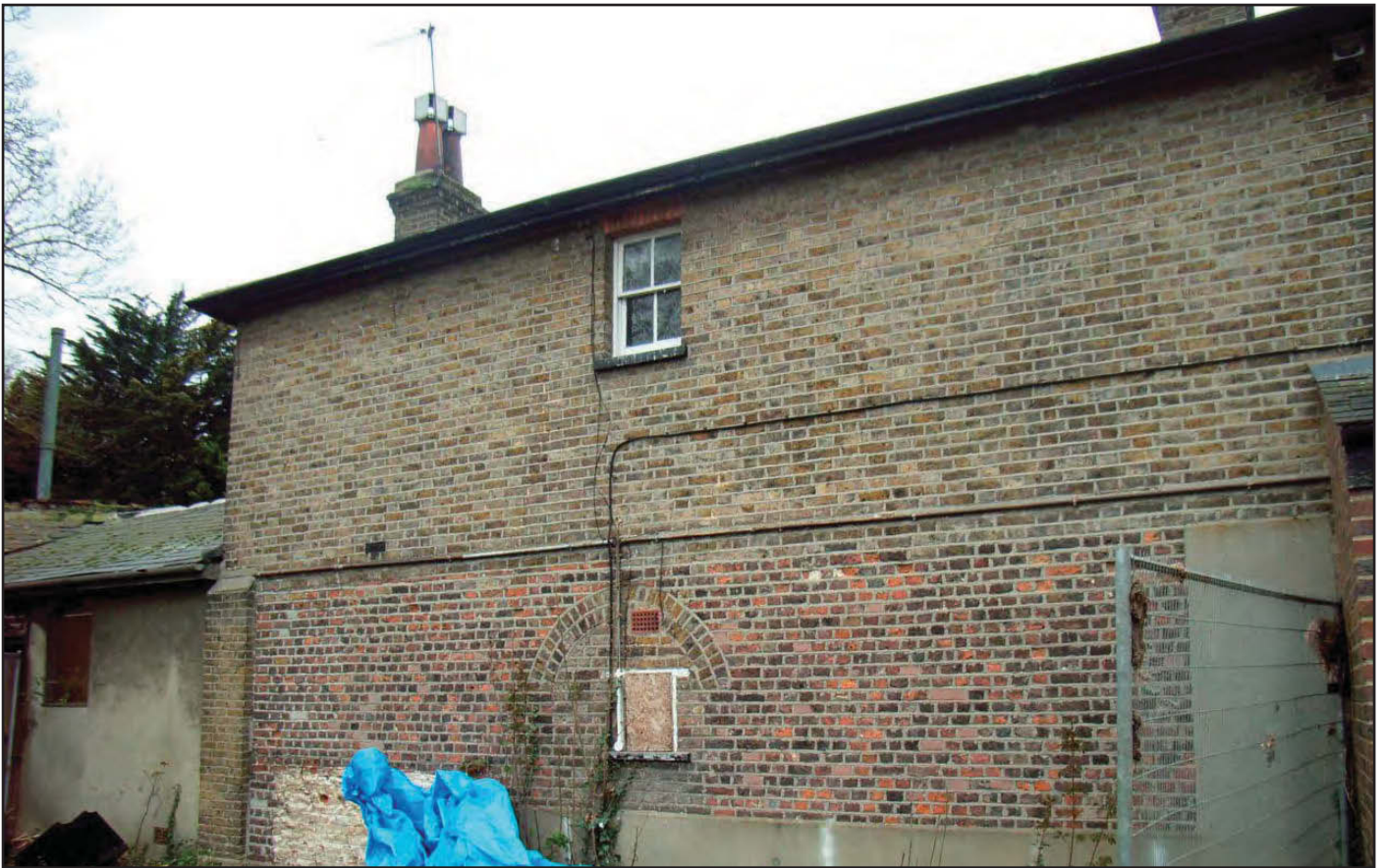
Plate 33: SE wall of Cottage showing 18th-century brick below 19th-century
