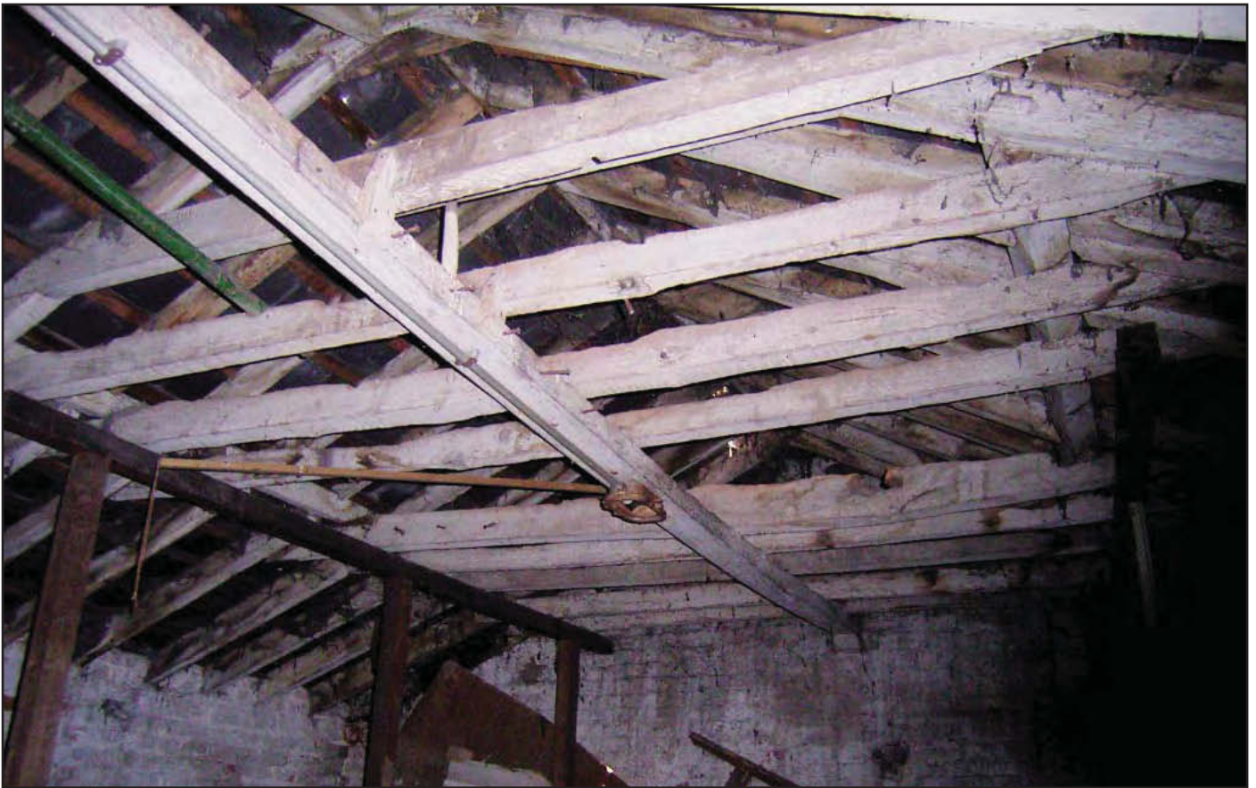
Plate 39: Roof in Granary
