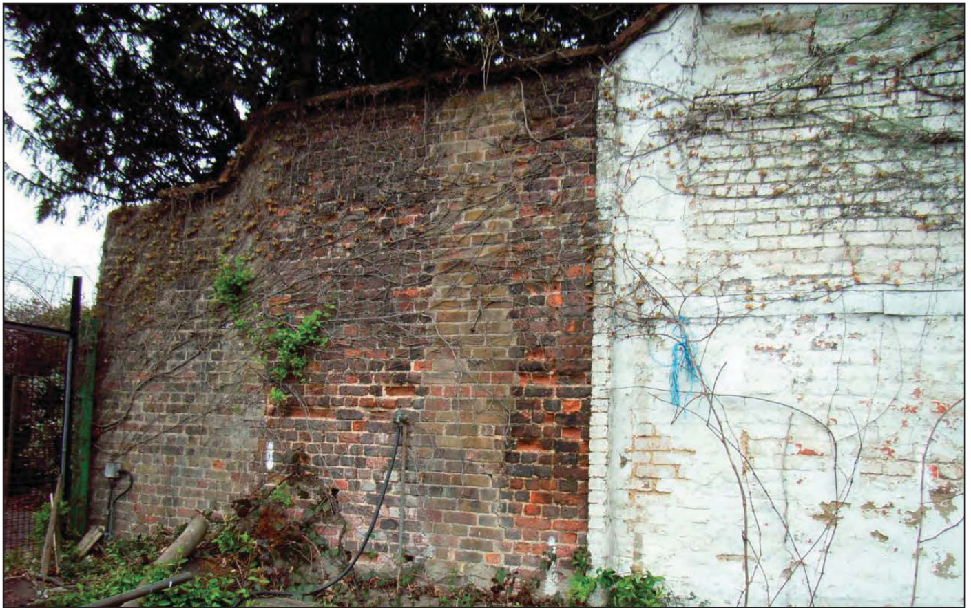
Plate 5: Pier of rebuilt brick towards centre of Wall 1 (Flue 1)
