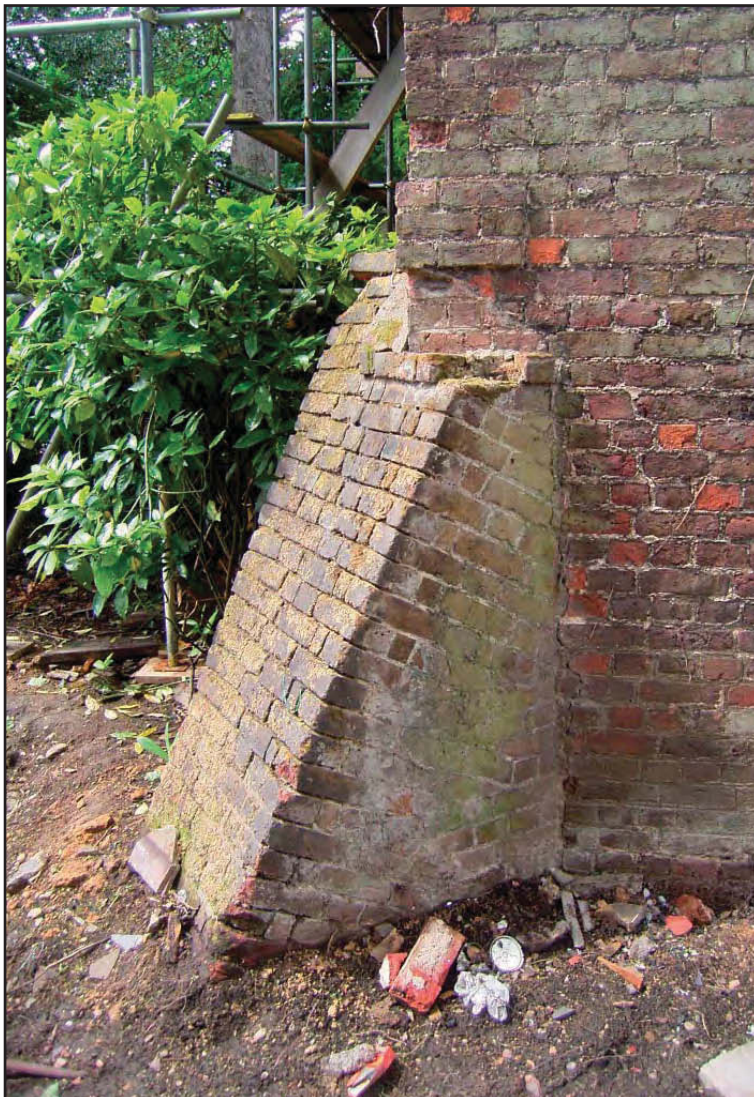
Plate 12: Later 19th-century buttress at south corner of Dovecote
