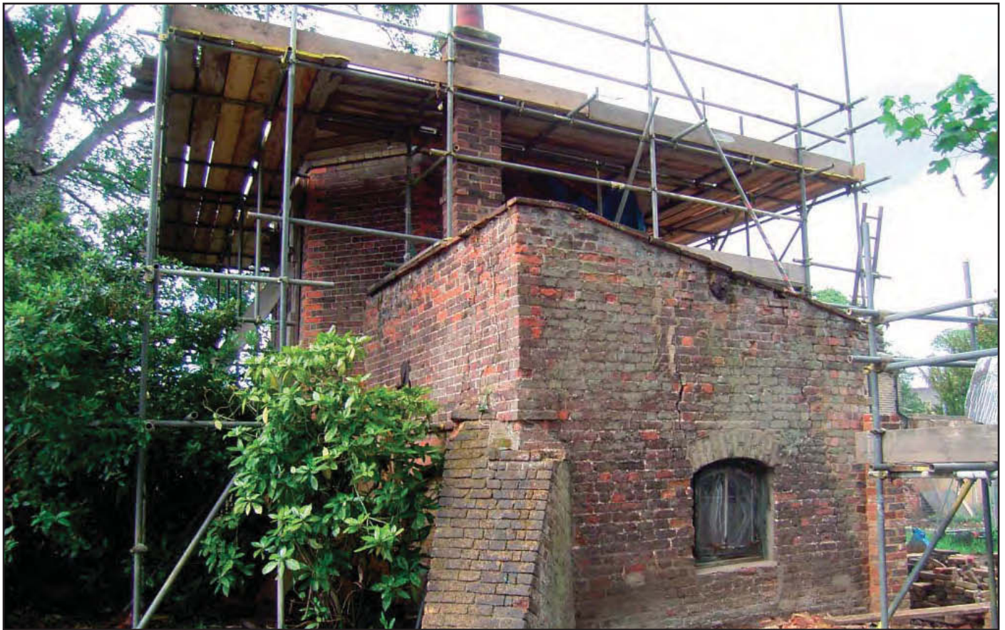
Plate 11: SE elevation of Dovecote with 18th-century brickwork at ground floor
