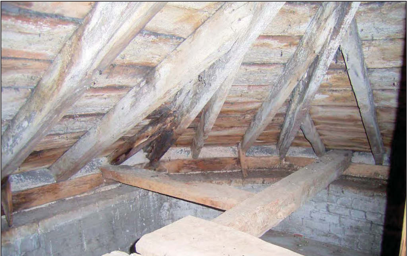
Plate 30: Roof detail in Dovecote
