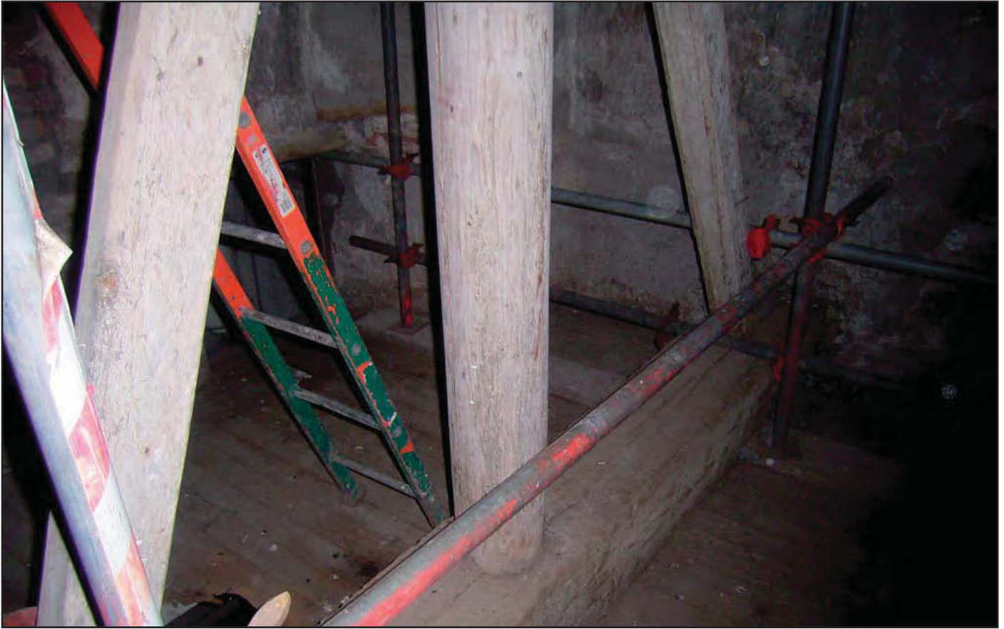
Plate 27: Bearer across floor in Dovecote supporting central post
