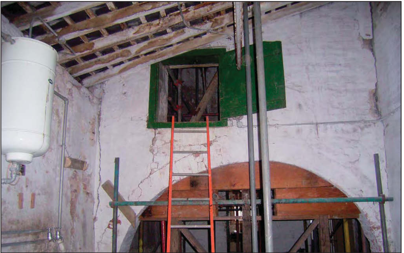
Plate 23: NW ground floor room in Dovecote
