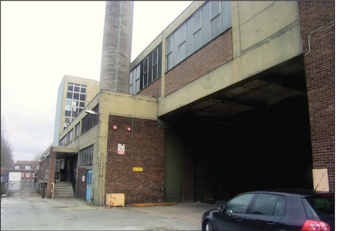
Plate 5: West elevation showing opening beneath Block B
