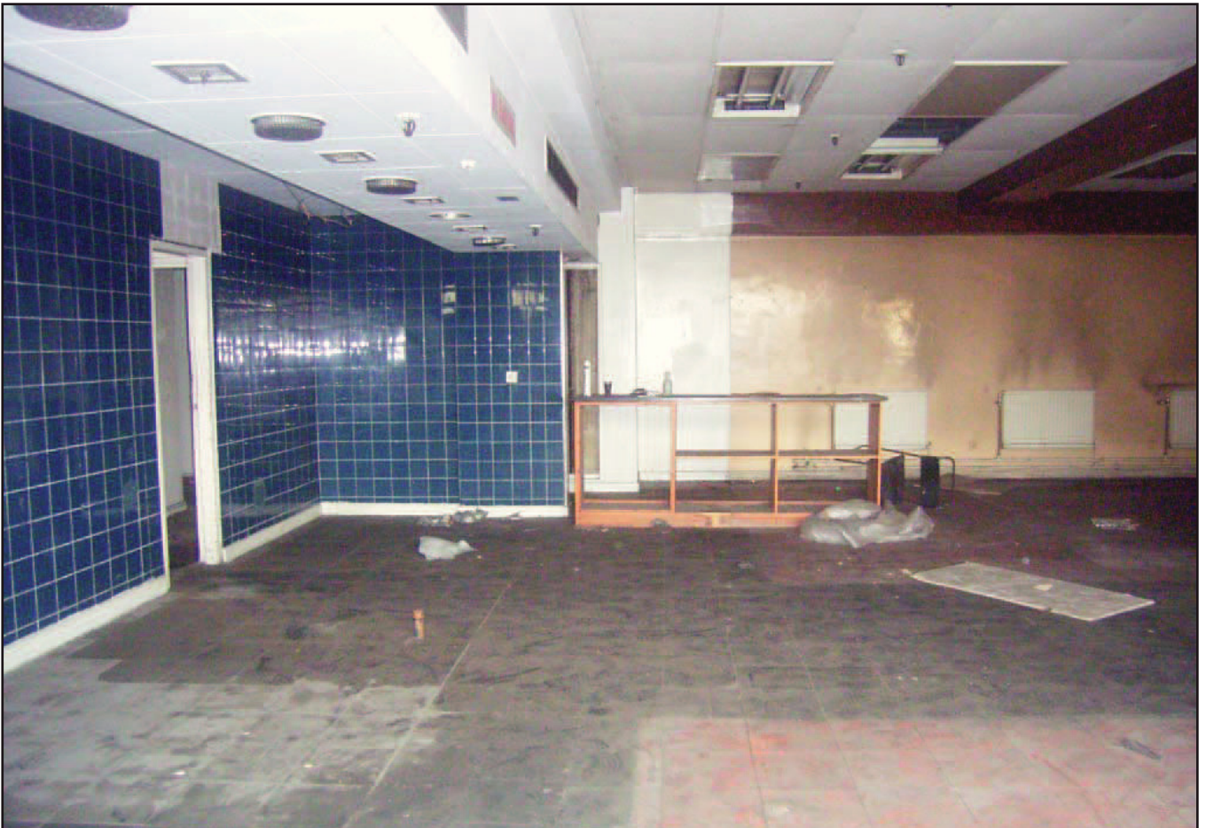
Plate 32: Canteen (Block A mezzanine between ground and first floor)
