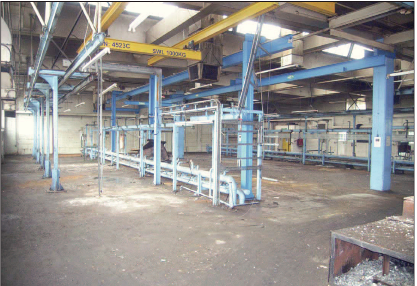
Plate 26: Foundry (1st floor Block C)
