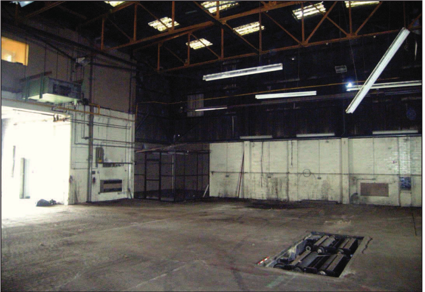
Plate 13: Block D (Eastway Zinc) interior
