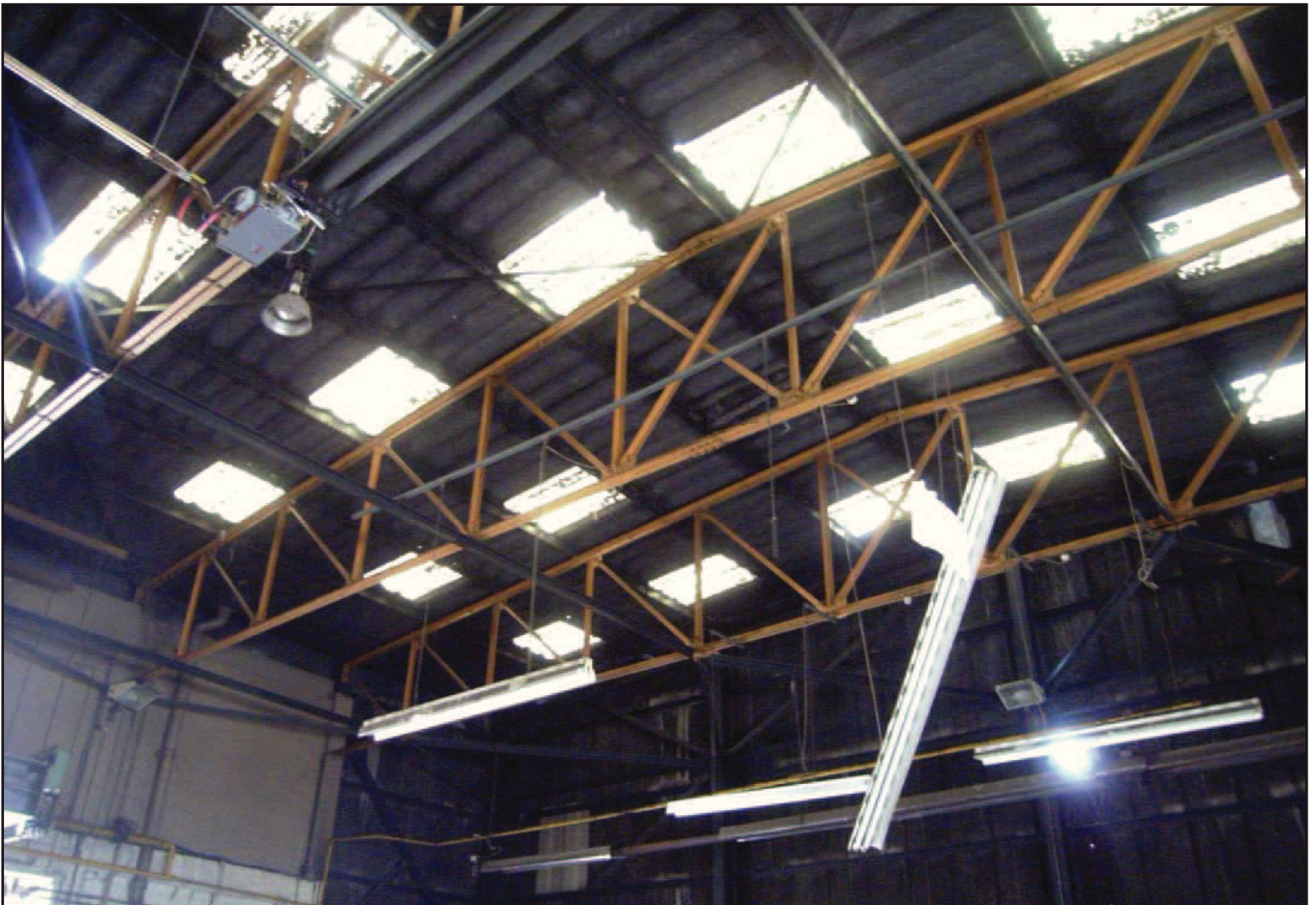
Plate 14: Roof in Block D (Eastway Zinc)
