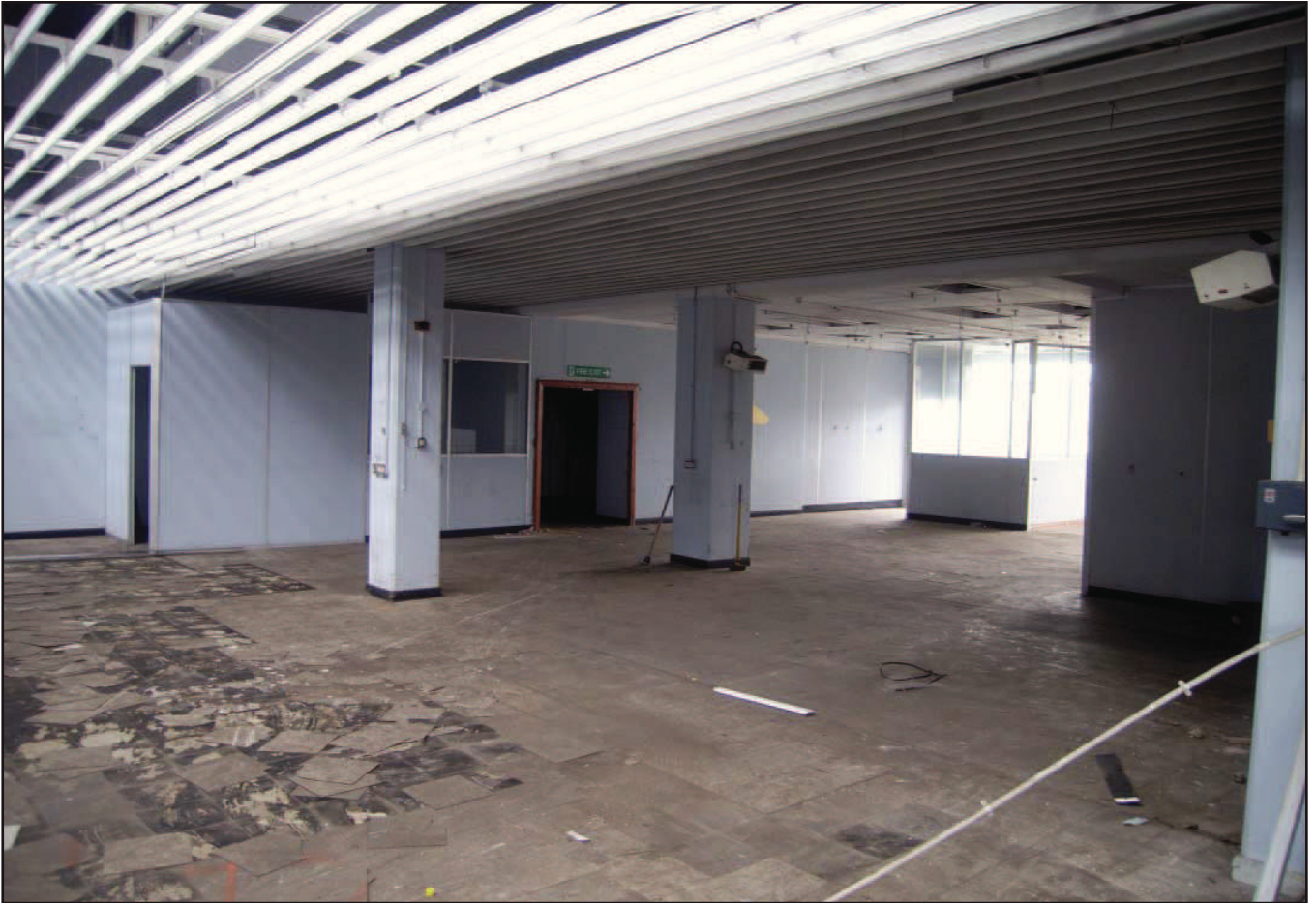
Plate 29: Second floor Block B
