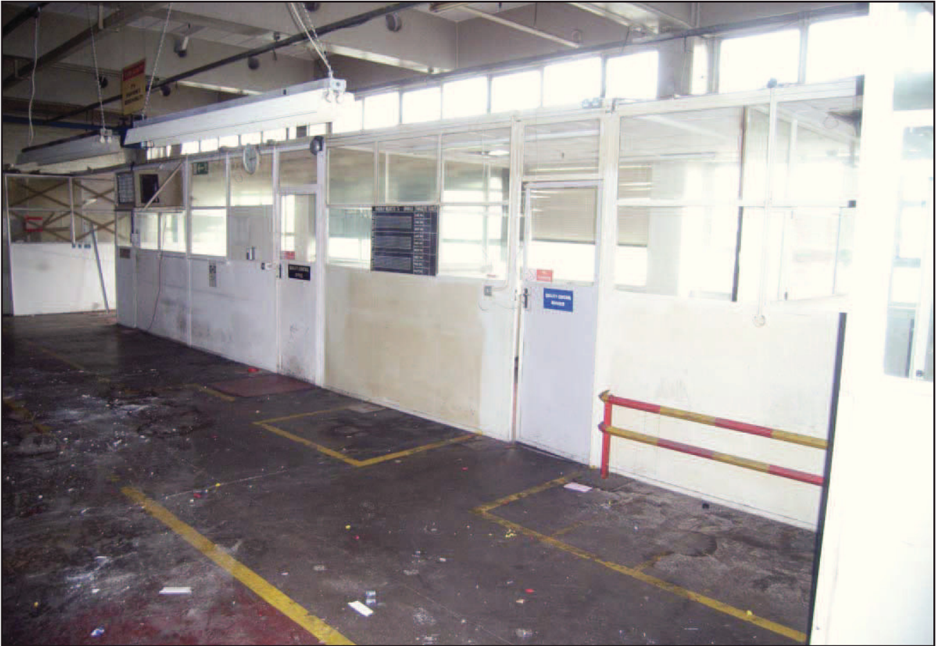
Plate 23: Offices at south end of Machining Dept (1st floor Block A)
