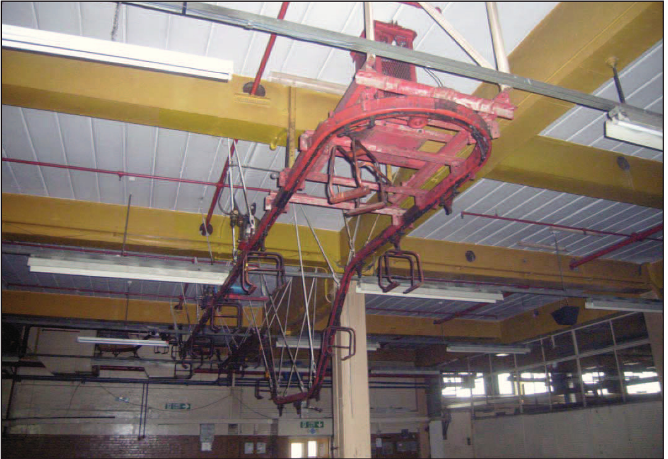
Plate 9: Overhead conveyor track in ground floor despatch area (Block B)
