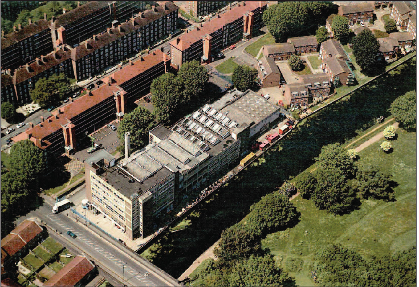
Plate 33: Aerial view of factory. Provided by Telford Homes
