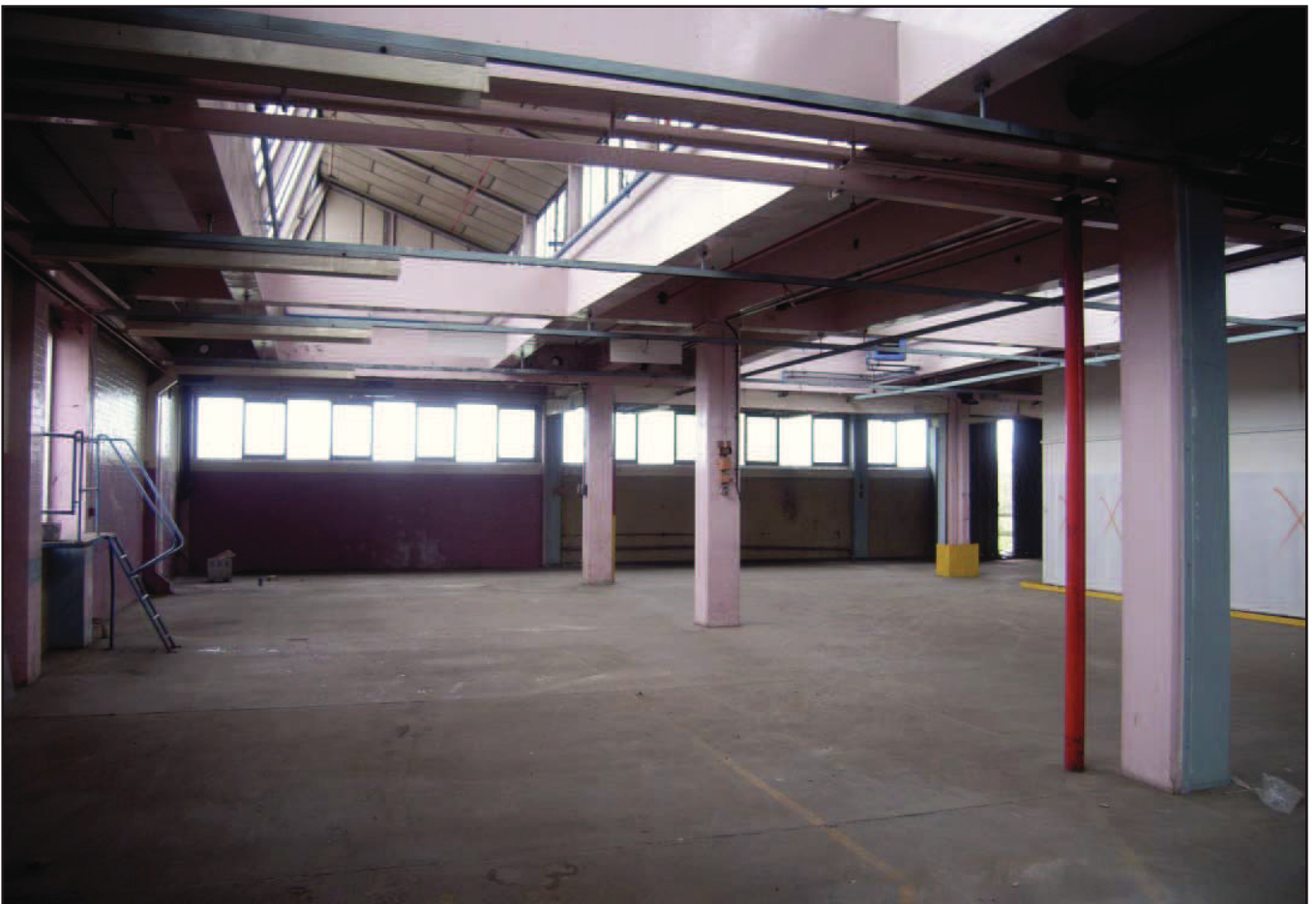
Plate 28: Storage area (2nd floor Block B)
