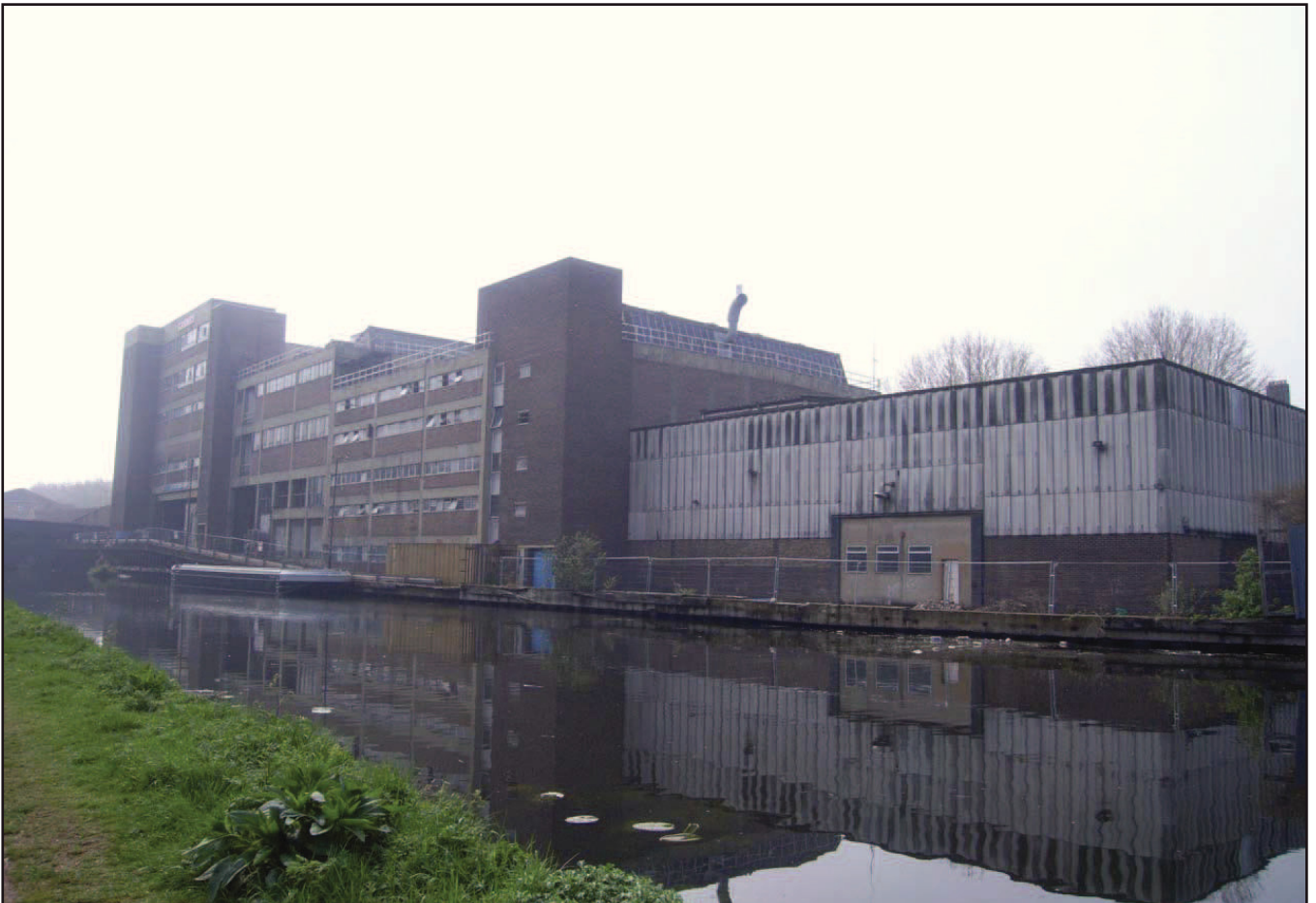
Plate 4: View of whole complex from north-east
