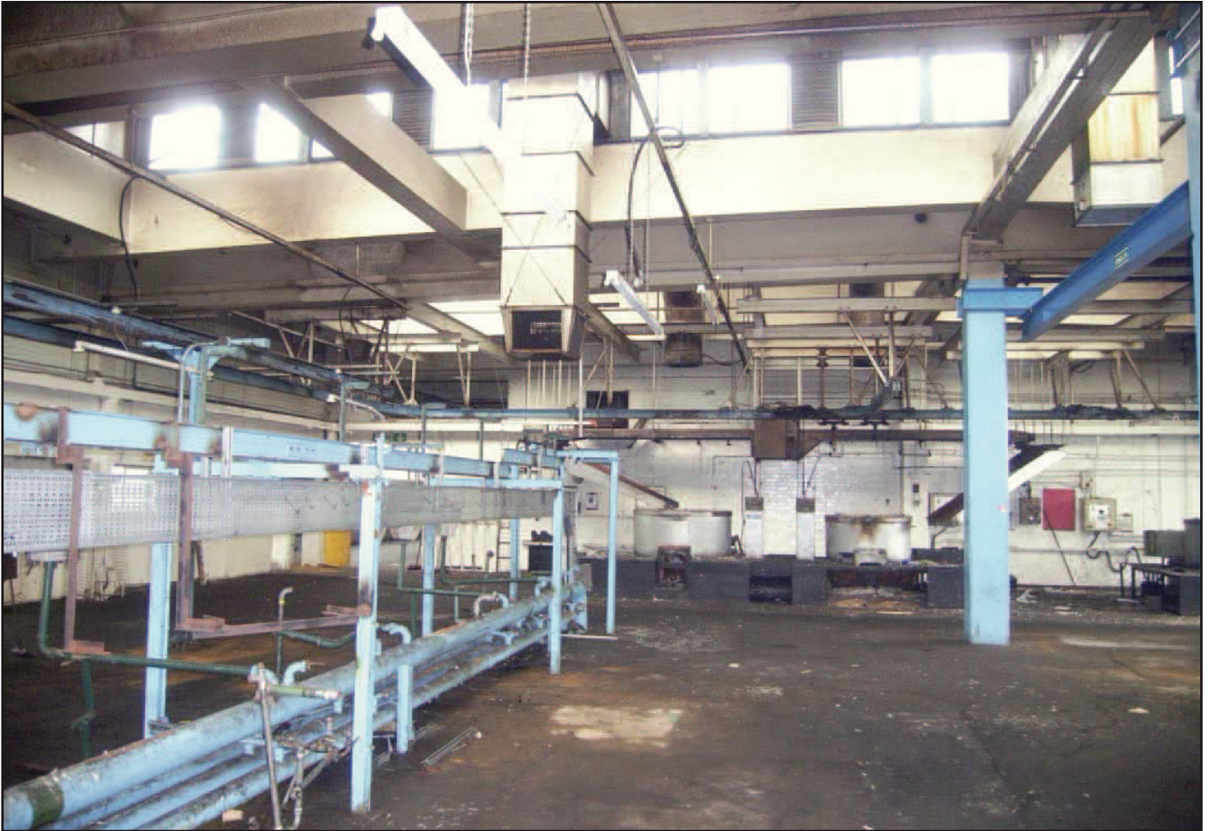
Plate 27: Foundry (1st floor Block C)
