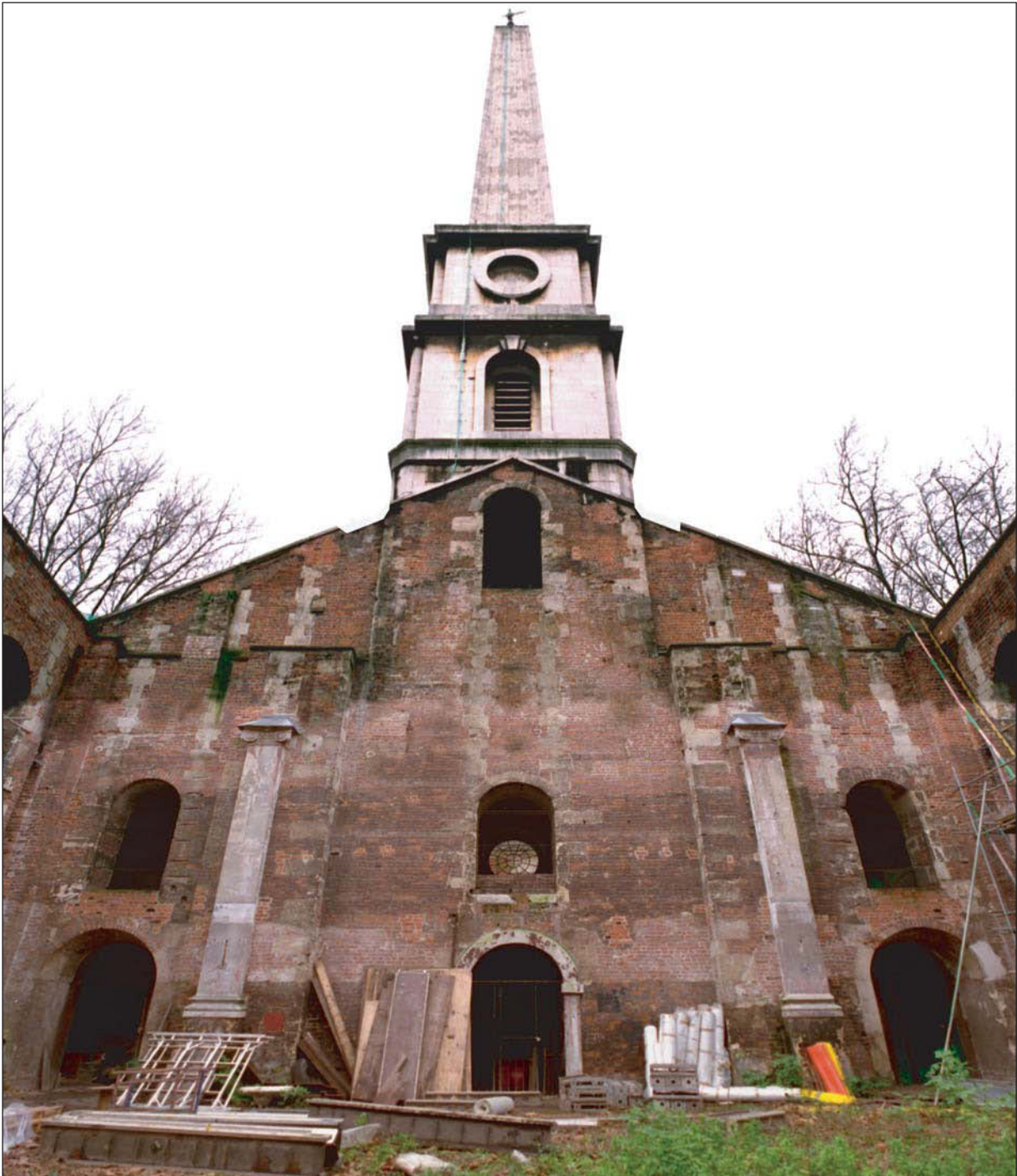
Plate 1.1: View of the tower from the interior of the church
