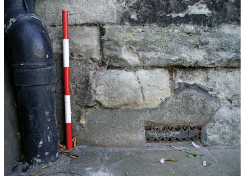
Plate 4: All Saints Vestry, Kingston: East elevation - repair at base of pipe
