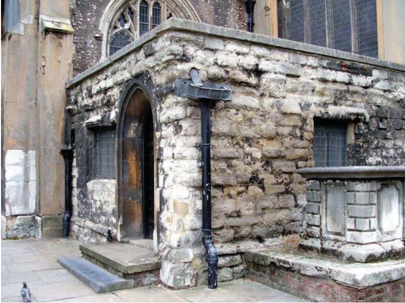
Plate 9: All Saints Vestry, Kingston: North Elevation - repairs to corner and discolouration of stonework caused by damp
