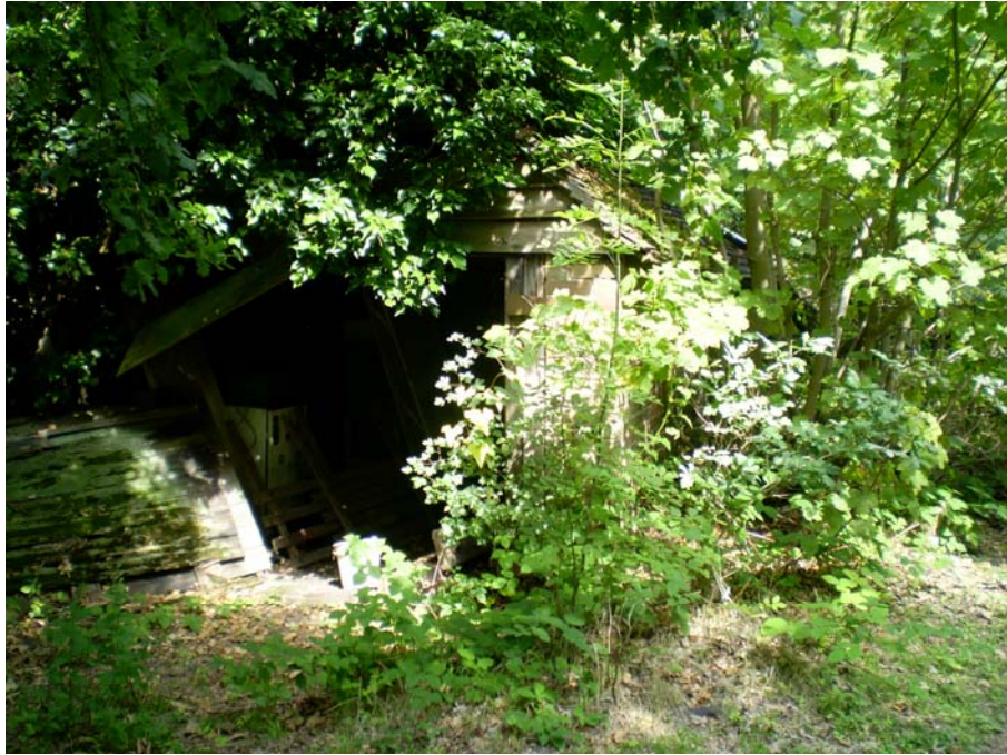
Photo: Feature E2 brick and tile shed
