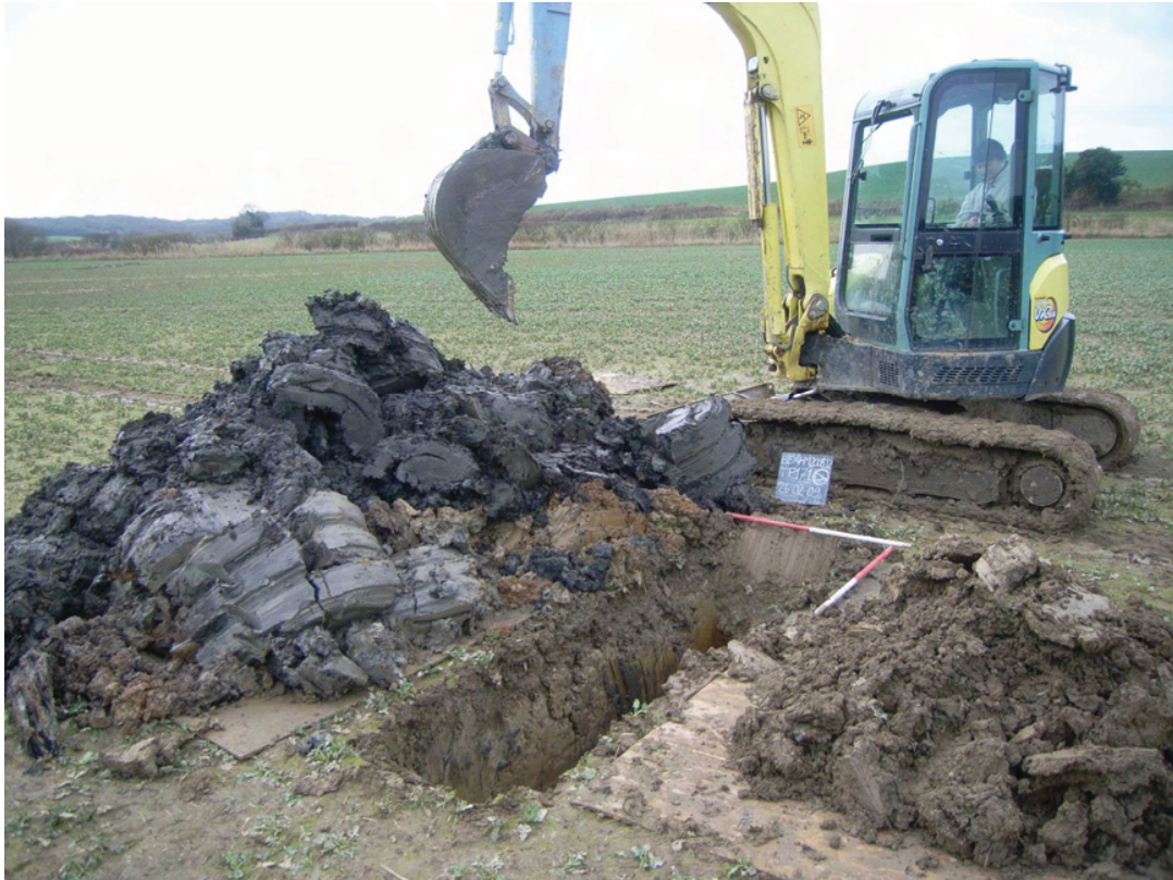
Plate 1: Photo of Test Pit 171 being excavated with a mini Digger
