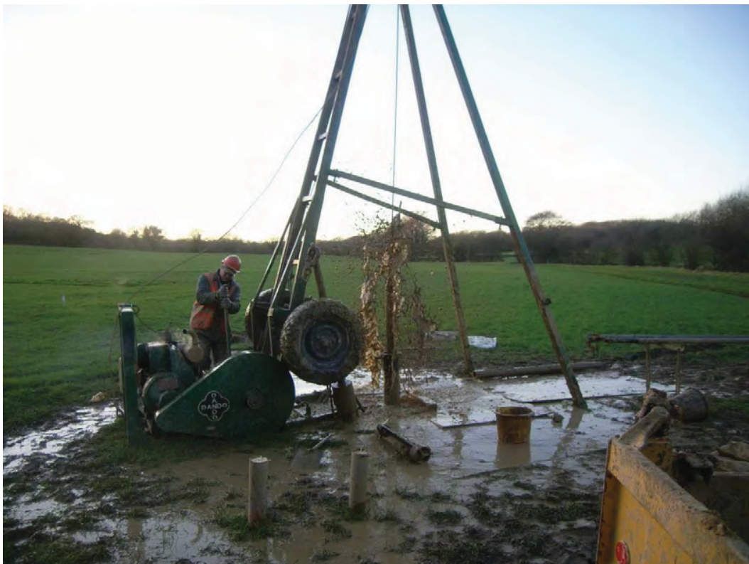
Plate 2: Photo of Borehole drilling using a cable percussion rig
