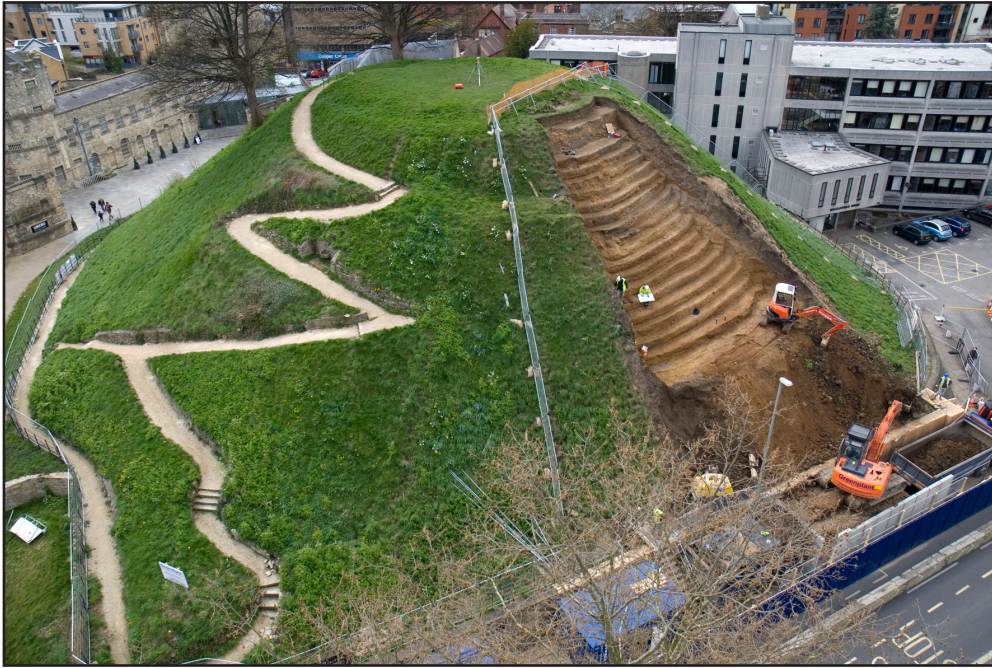
Plate 3: Working view removing slumped material of mound
