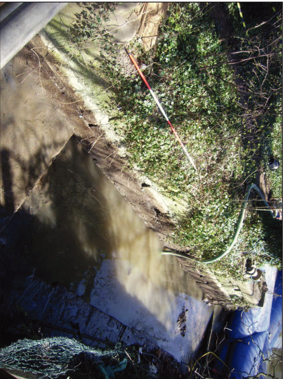
Plate 1 : Mill race, drained prior to deposition of concrete
