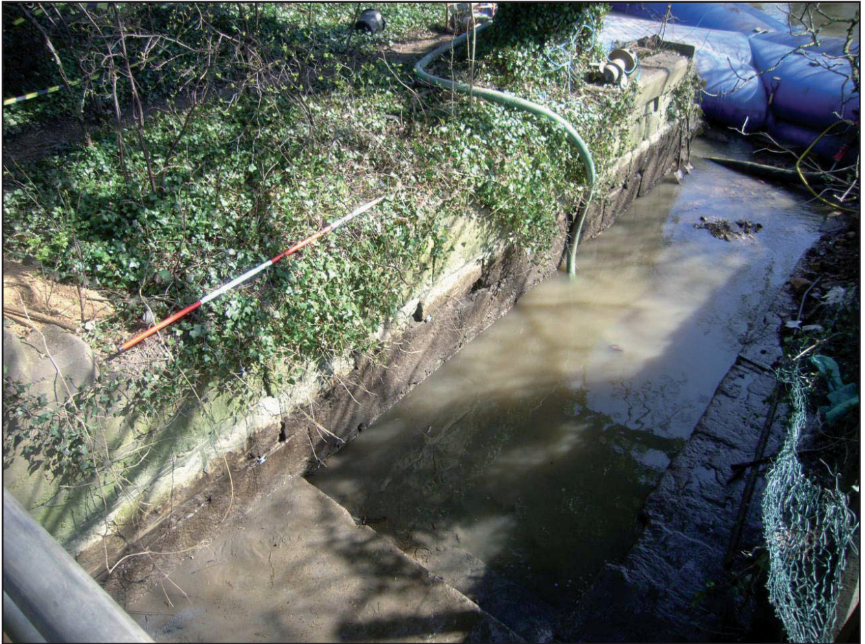
Plate 1: Mill race, drained prior to deposition of concrete
