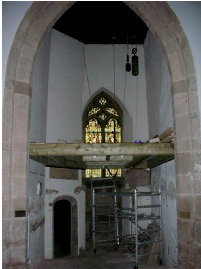
Plate 22: Tower (looking west), with mezzanine floor partially inserted
