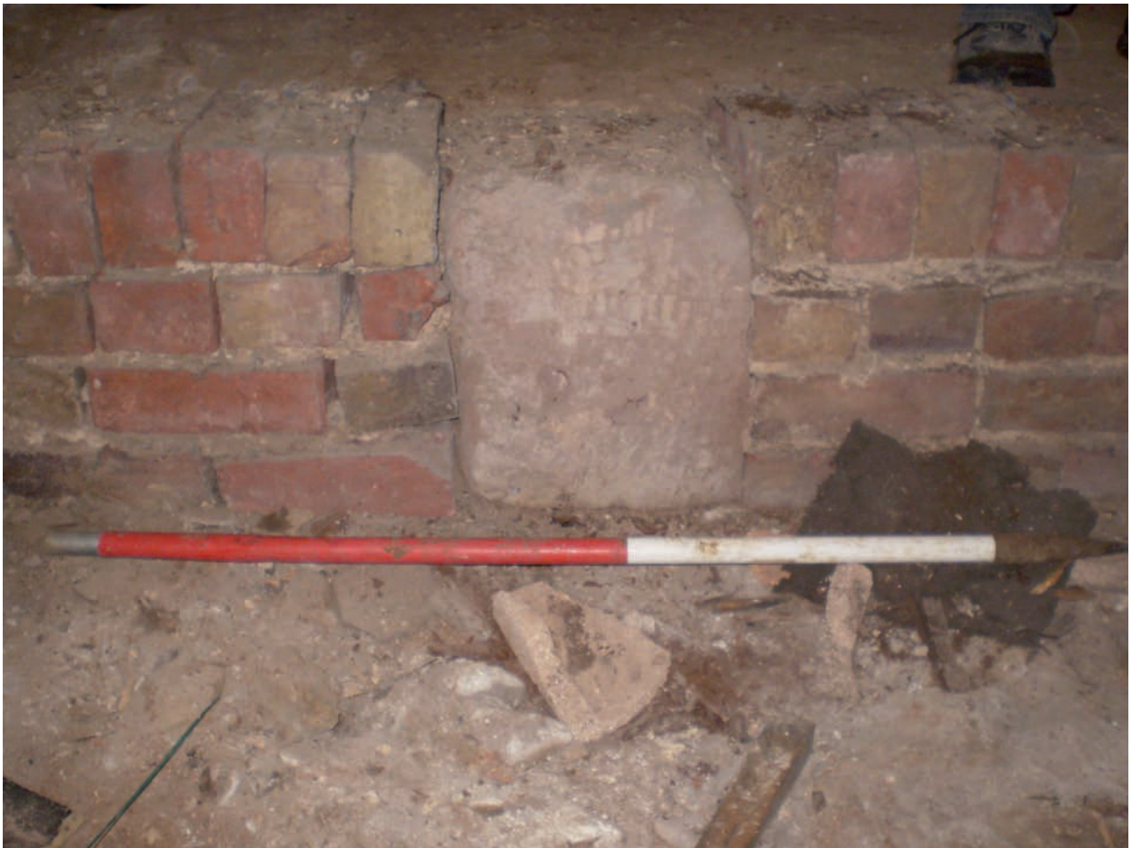
Plate 12: Brick floor support wall 117. Note the dressed masonry built into it (looking north)
