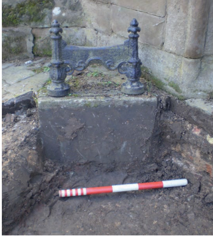
Plate 31: Boot scraper on east side of north porch door (looking south-east). Note the stone footing
