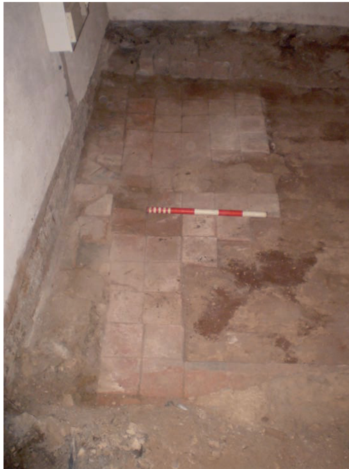
Plate 16: Part of tiled floor surface 106 (looking south). Note the broken tiles and stone used to fill the gap along the eastern edge
