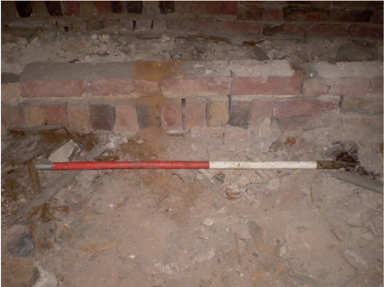
Plate 11: A brick floor support wall (100)
