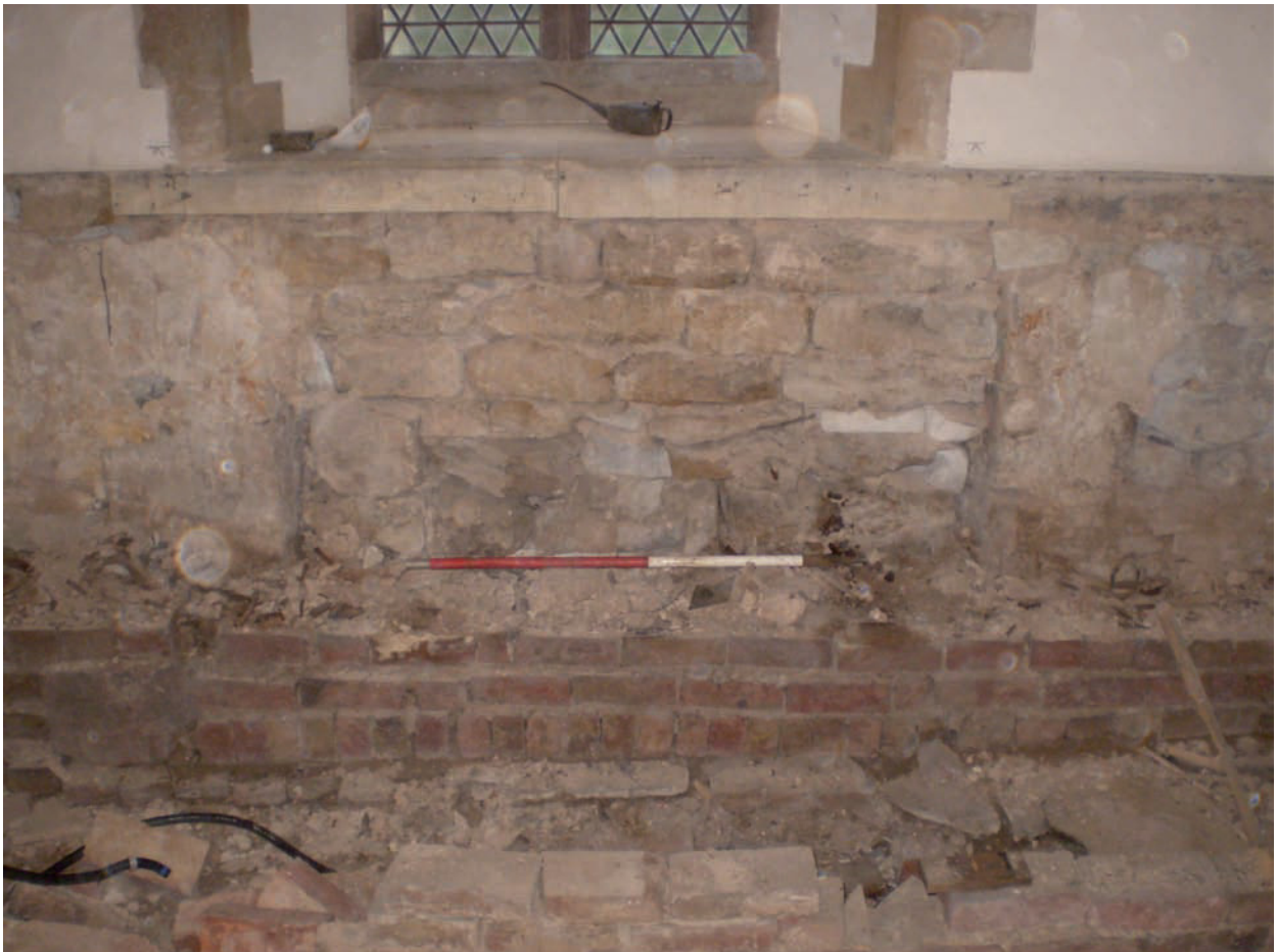
Plate 18: Blocked doorway 104 in south wall of south aisle (looking south)
