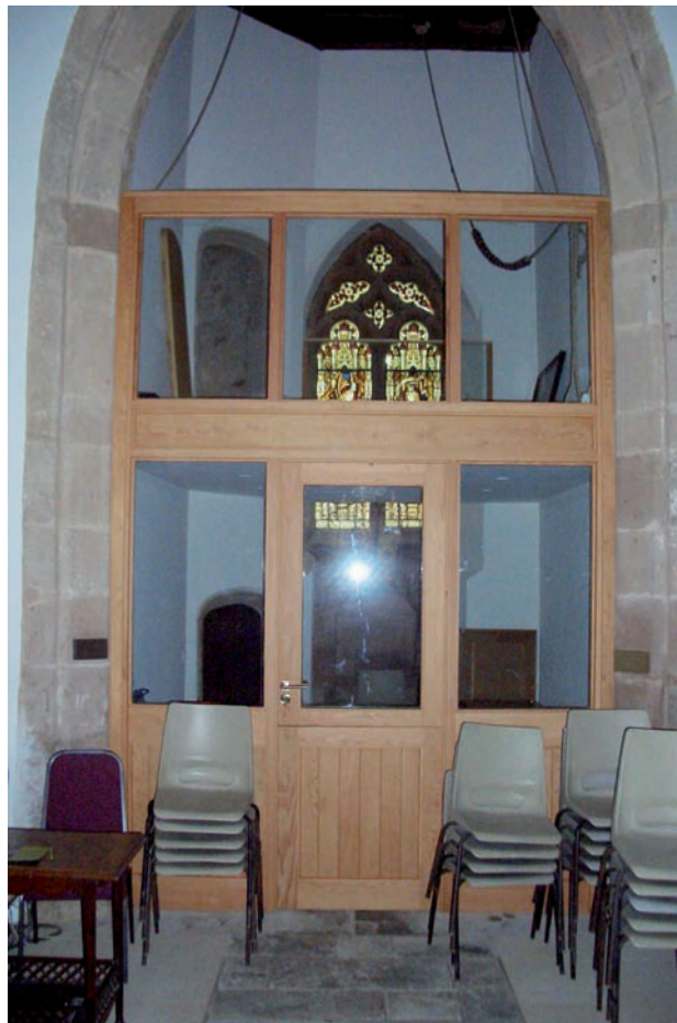
Plate 24: Tower (looking west), after completion of mezzanine floor and new access door
