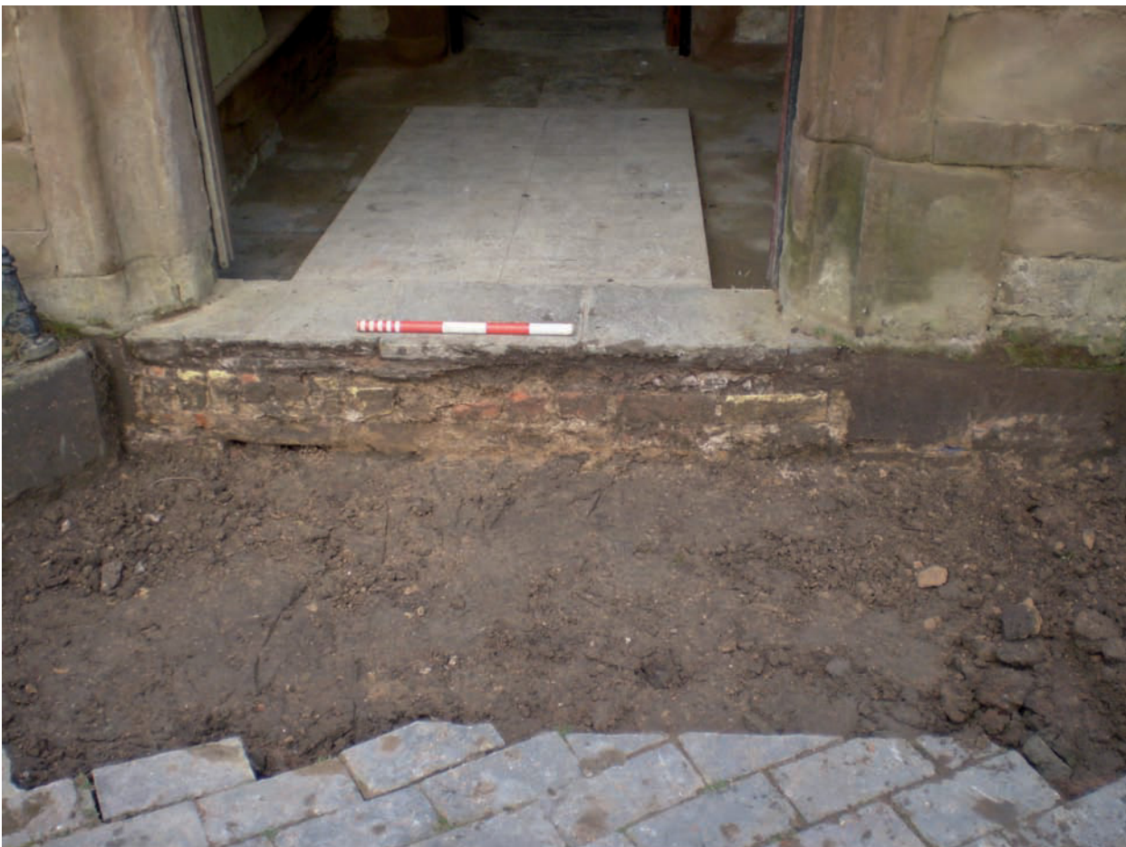
Plate 30: Footing of porch step 303 (looking south)
