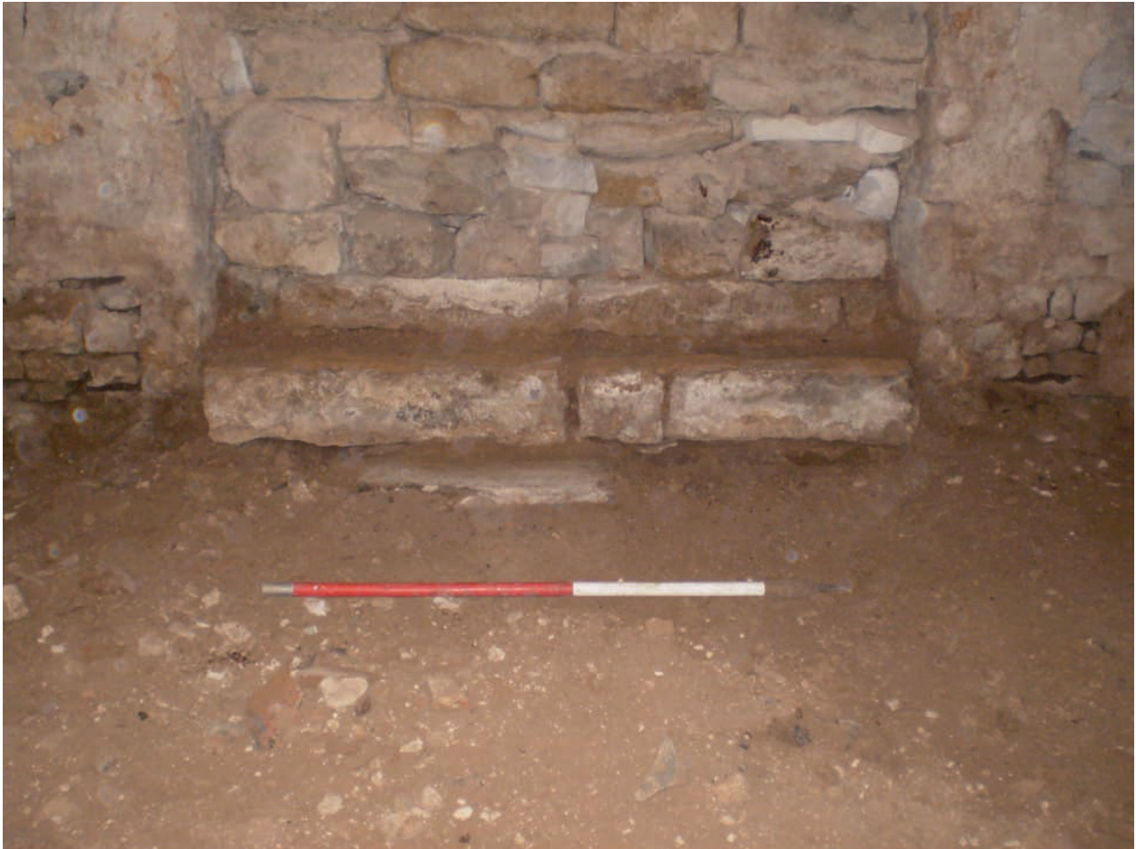
Plate 19: Steps of blocked doorway 104 (looking south)
