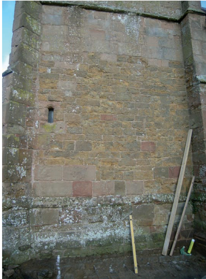
Plate 5: South wall of west tower (9) (looking north)
