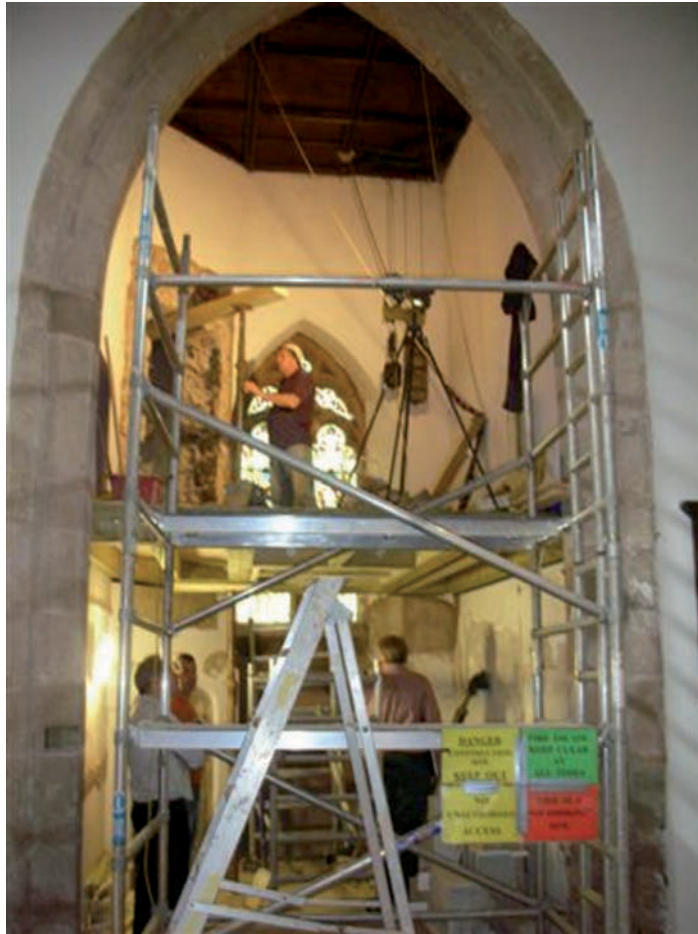
Plate 23: Tower (looking west), new access door to mezzanine floor partially opened
