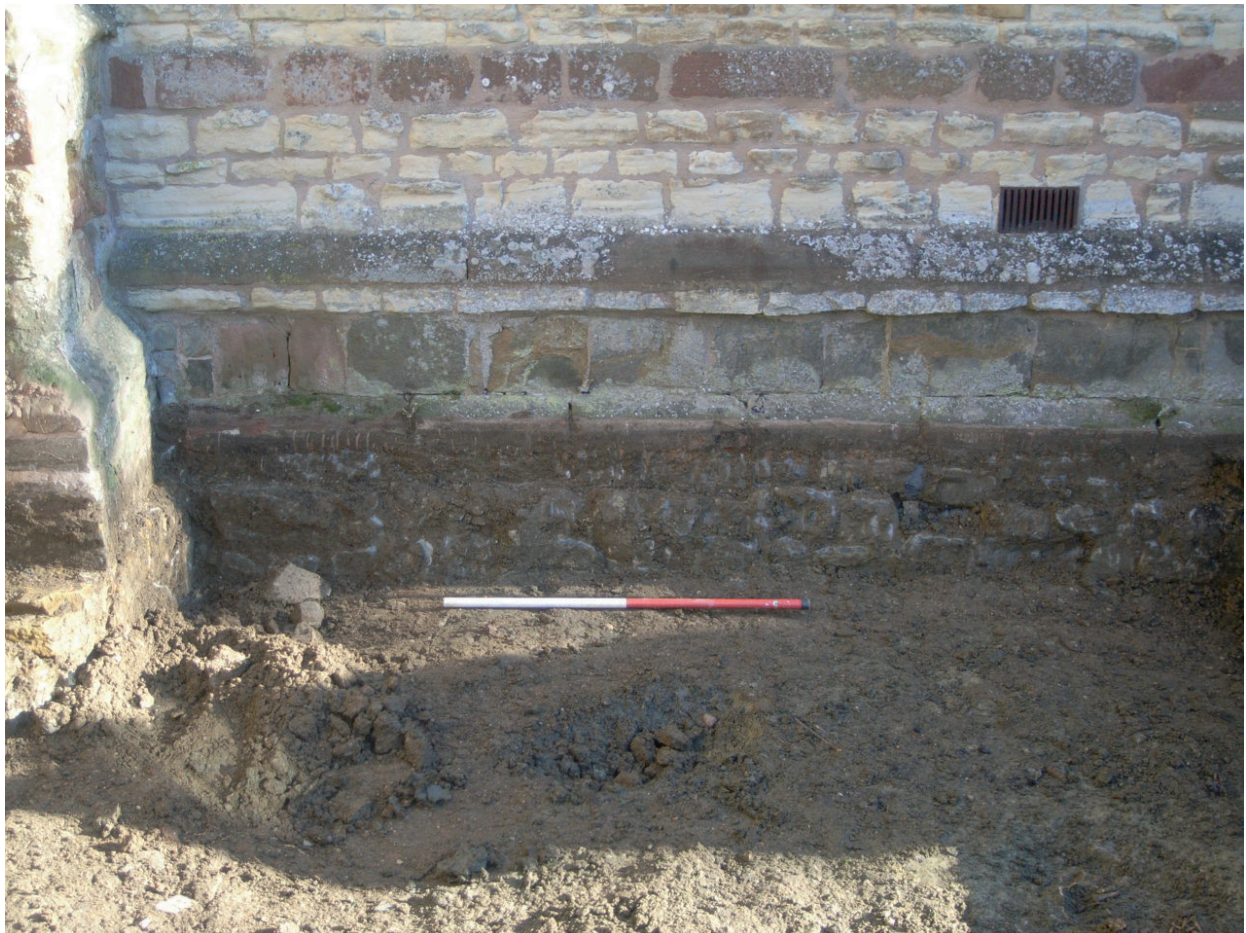
Plate 10: Foundation 12, for wall 13 (looking east)
