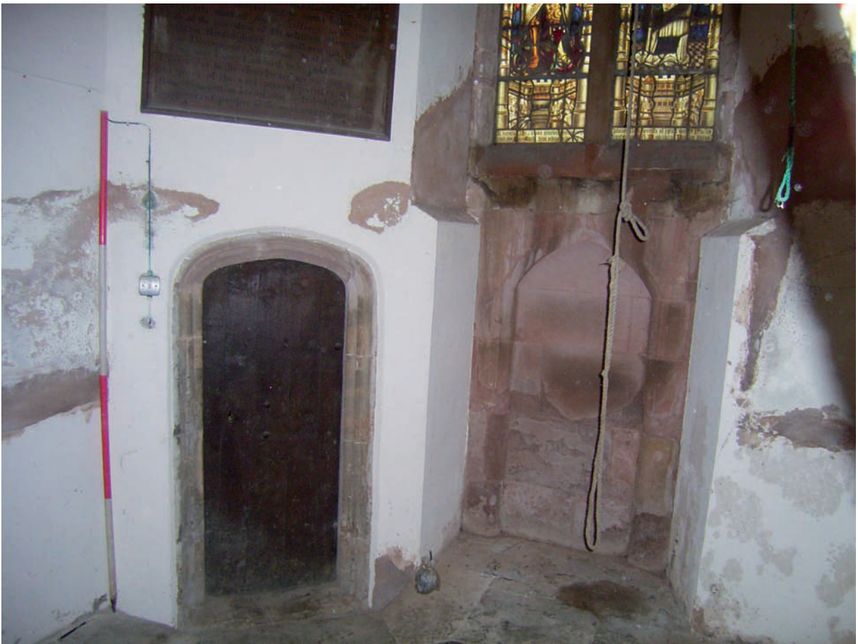
Plate 1: West tower, looking south-west. Note the blocked doorway below the stained glass window
