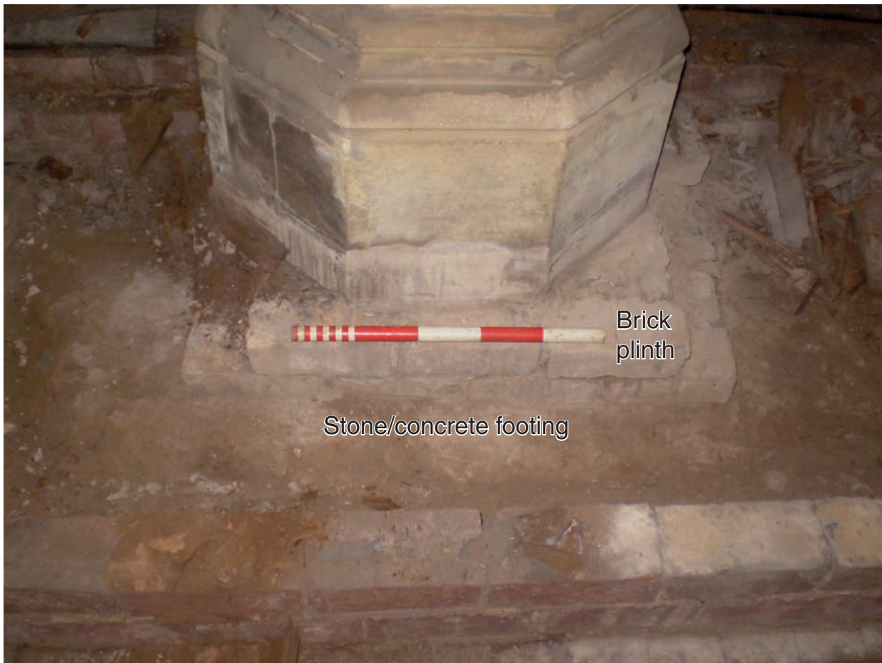
Plate 14: 19th century column base. Note the brick plinth and stone/concrete footing
