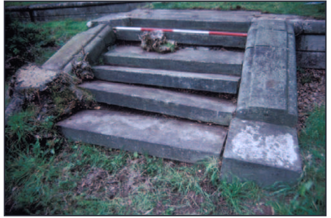
Plate 56 - Trench 103, shows current surviving state of steps S9. Looking west.
