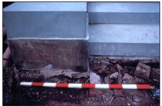
Plate 46 - Trench 3, reinstated stonework on steps S3. Looking north.
