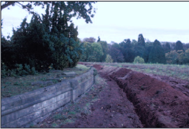
Plate 67 - Service trench excavated along east side of eastern balustrade of gardens for new pumphouse. Looking north.
