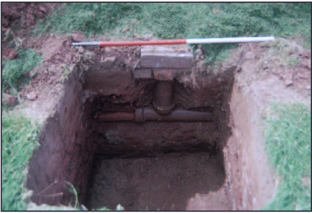
Plate 27 - Trench 11, trial pit excavated by garden contractor to examine drainage. Looking south west.
