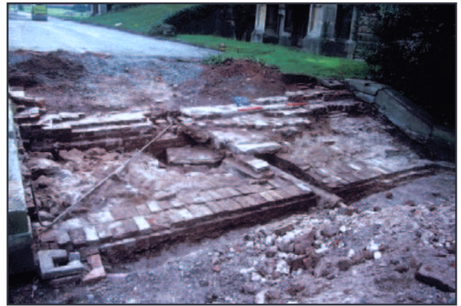
Plate 52 - Trench 100, excavation of step foundations S16 in East Parterre garden. Looking south west.
