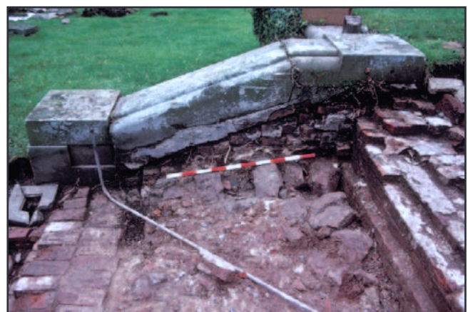
Plate 54 - Trench 100, detail of surviving stringer of steps S16. Looking east.
