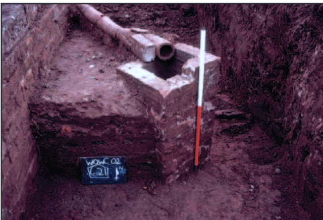
Plate 45 - Trench 20, detail of drainage recorded in area of new pumphouse. Looking north.
