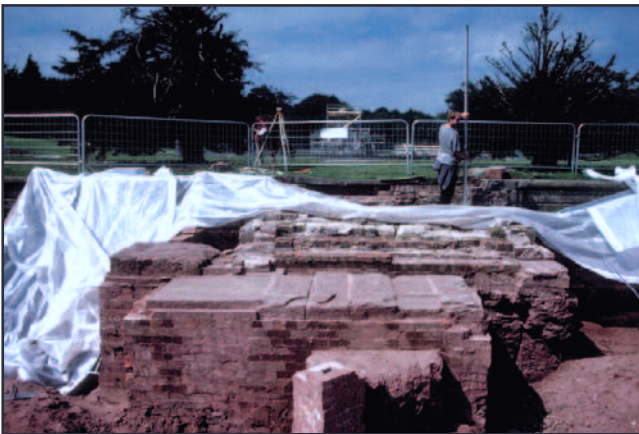
Plate 63 - Trench 20, fountain tunnel entrance exposed. Looking west.
