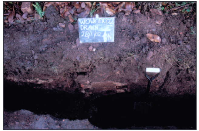
Plate 70 - Drain recorded during monitoring works carried out along service trench excavated to the north of the house. Looking north.
