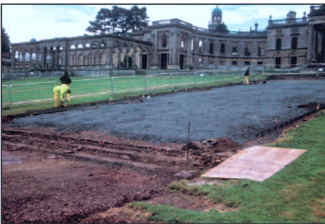
Plate 29 - Trench 6, surviving step foundations S5 with central path being prepared for re-surfacing. Looking north west.
