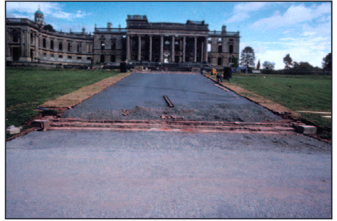
Plate 50 - Preparation of paths for re-surfacing with steps S5 in foreground. Looking north.
