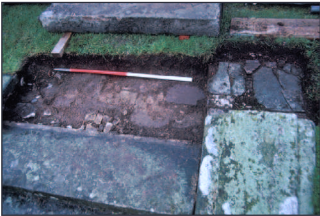
Plate 9 - monitoring works carried out during removal of step stonework, steps S2. Looking north.
