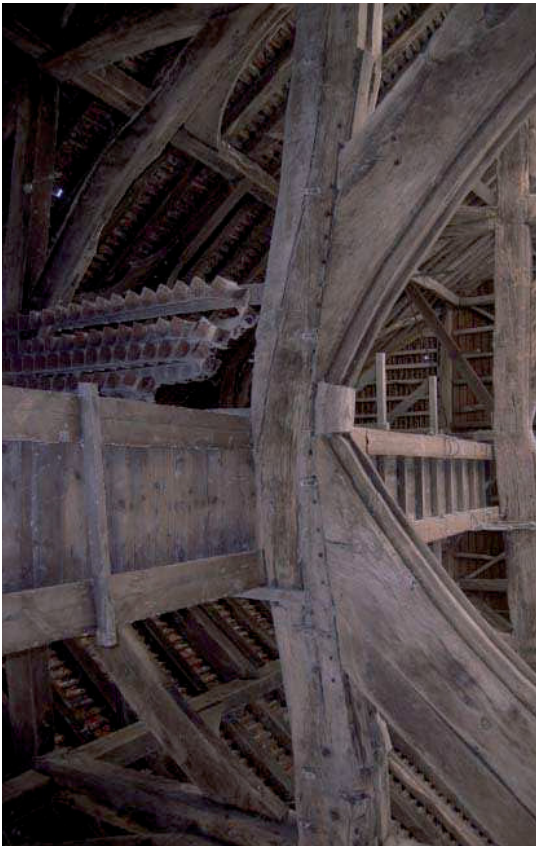
Plate 9: Detail of Frame 2 and 20th-century gantry
