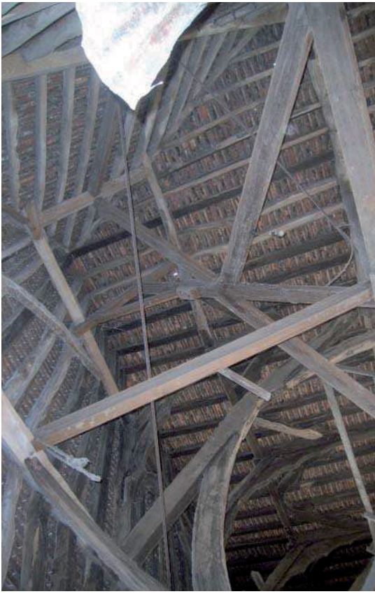
Plate 17: Secondary west end of barn
