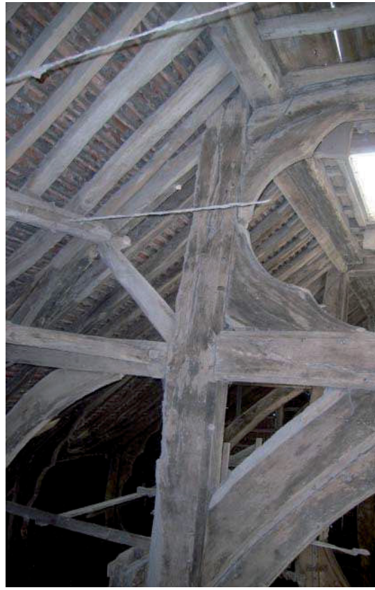
Plate 11: Detail of framing in Frame 3
