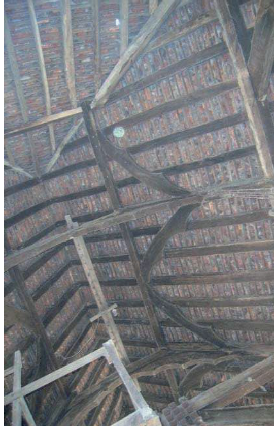
Plate 10: View of roof at east end of barn
