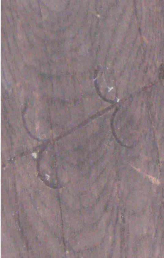
Plate 20: Carpenters mark on Frame 3 (W central)
