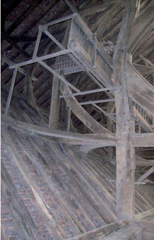
Plate 8: Roof in east half of barn
