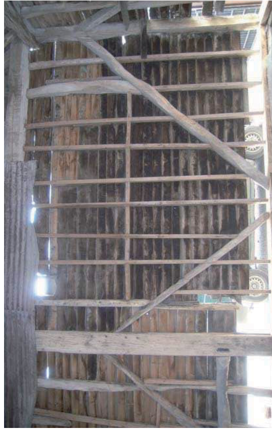
Plate 15: Secondary frame at W end of barn
