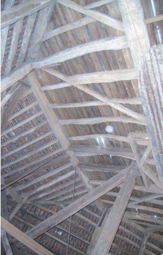
Plate 16: Secondary west end of barn
