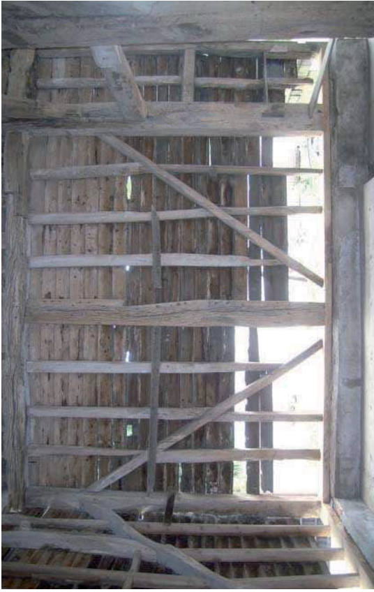
Plate 13: Secondary framing and possibly reused tie at W end of N wall
