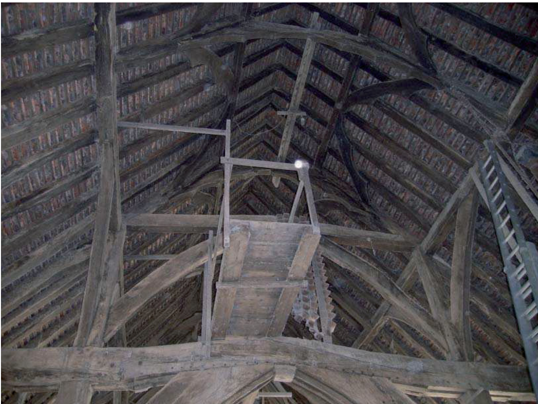
Plate 7: Roof in east half of barn
