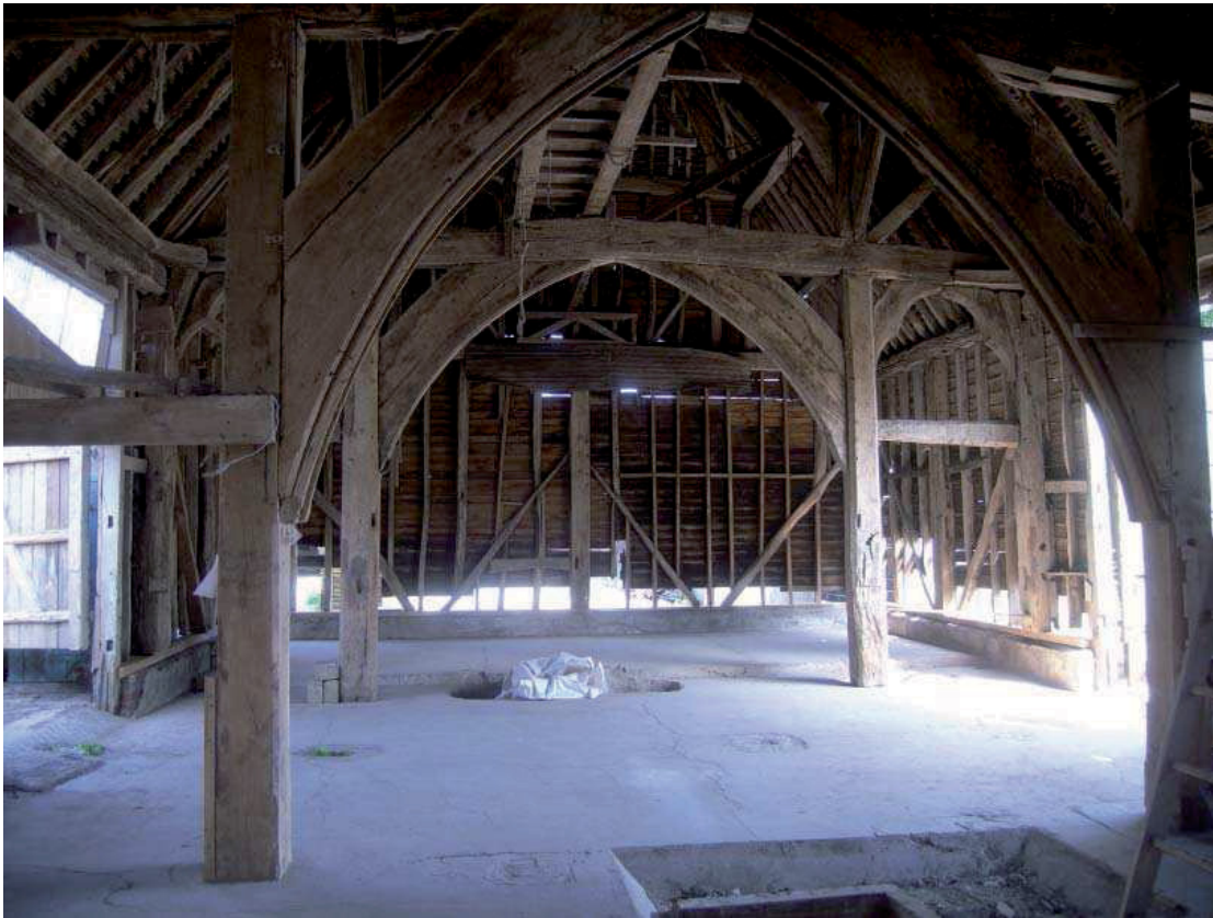
Plate 6: General internal view of barn from east
