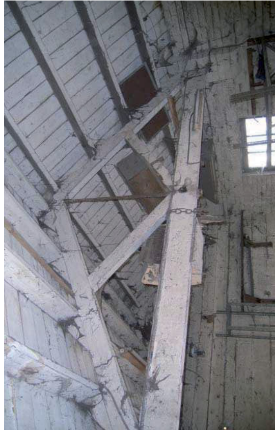
Plate 27: Interior of north room of stable range
