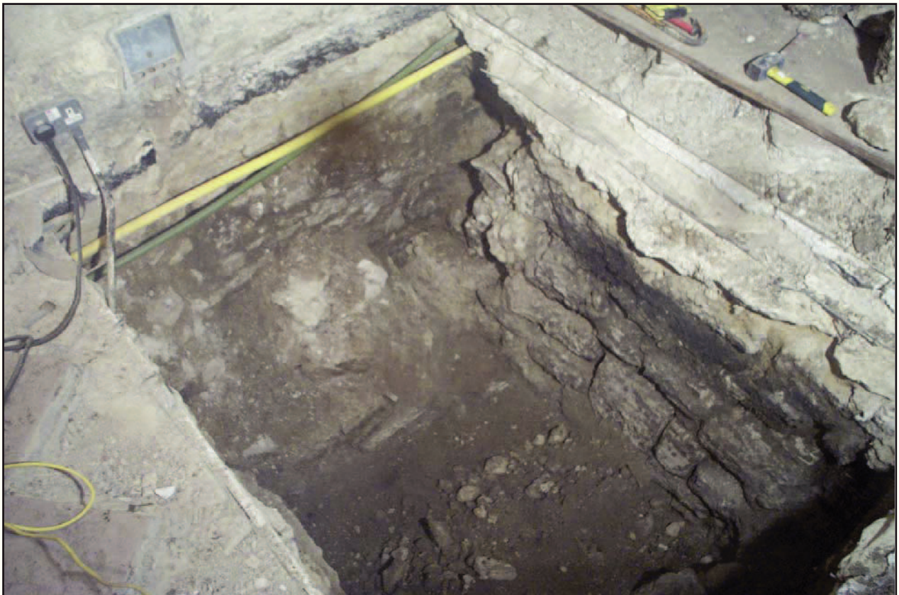
Plate 6: Trench 3 Footing 313 following partial dismantling of wall 305
