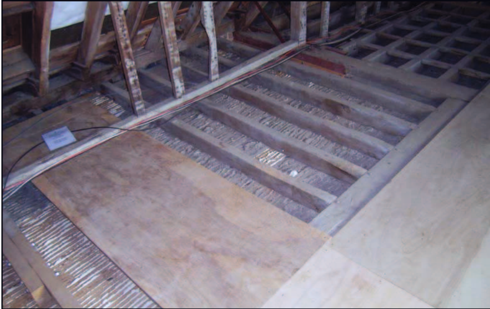
Plate 30: Central bay (6th) where a staircase might have been placed
