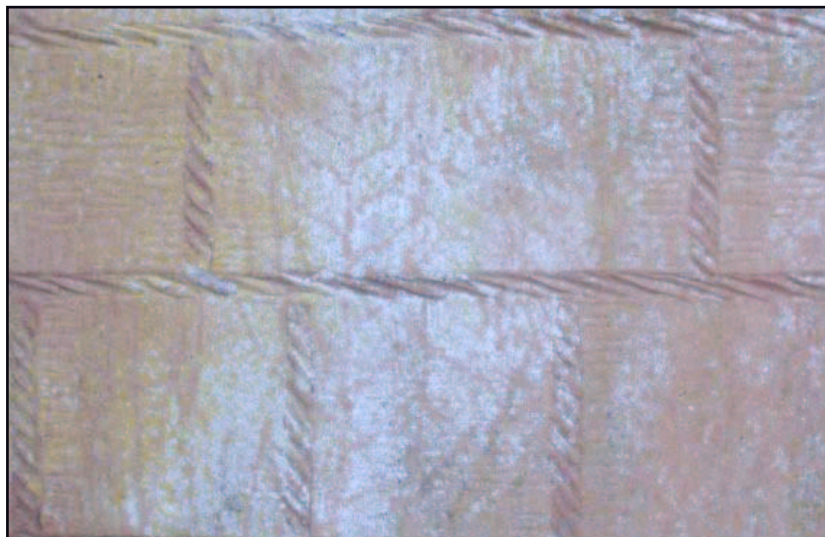
Plate 13: Main fabric. South facade
