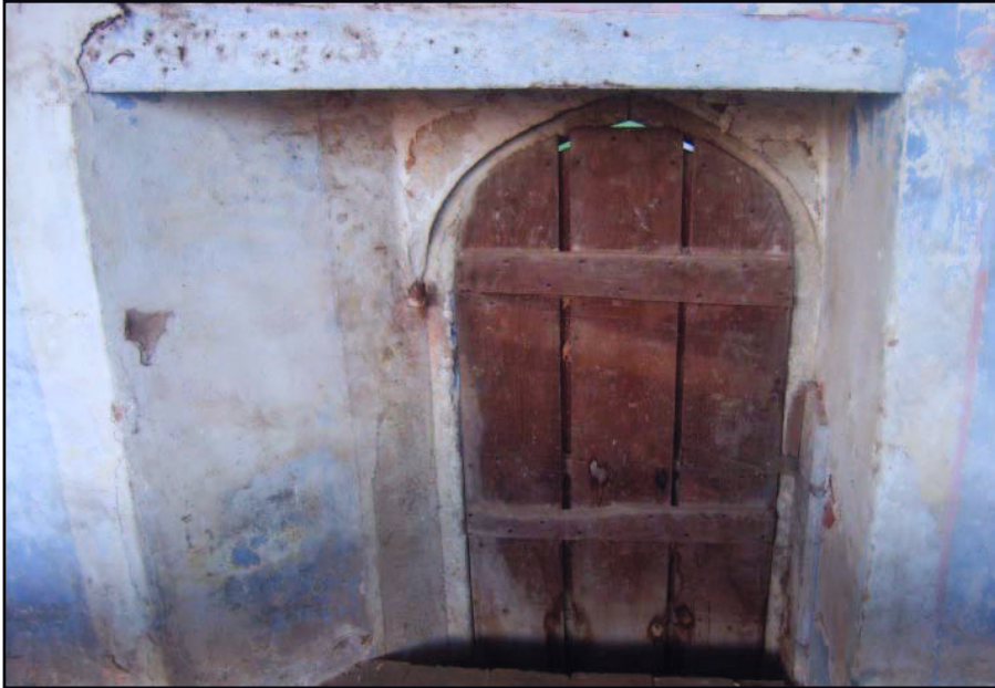
Plate 18: Central doorway in the north wall, inside
