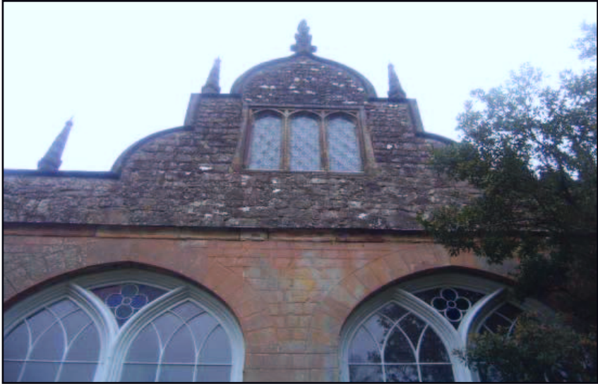
Plate 14: Gable, south facade
