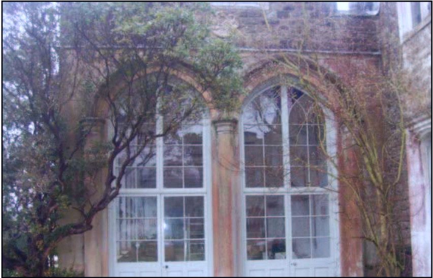
Plate 16: Doors, east facade
