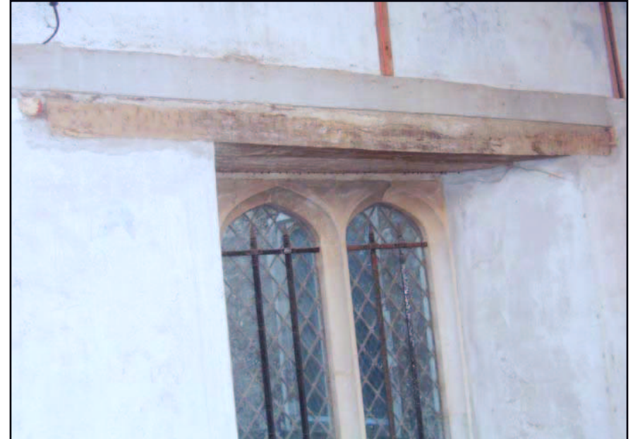
Plate 19: Lintel of a window on the ground floor north wall
