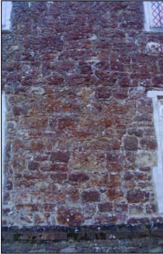
Plate 10: Phasing in north facade from insertion of windows
