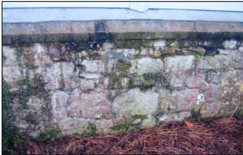
Plate 12: Base of the south facade with partially coursed stone
