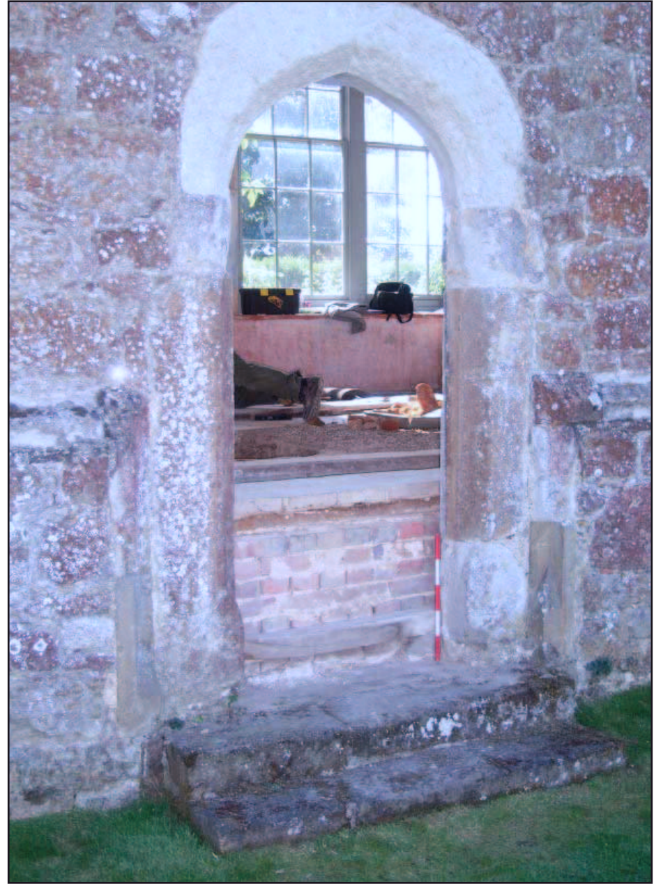
Plate 42: Former doorway in north wall showing raised floor level
