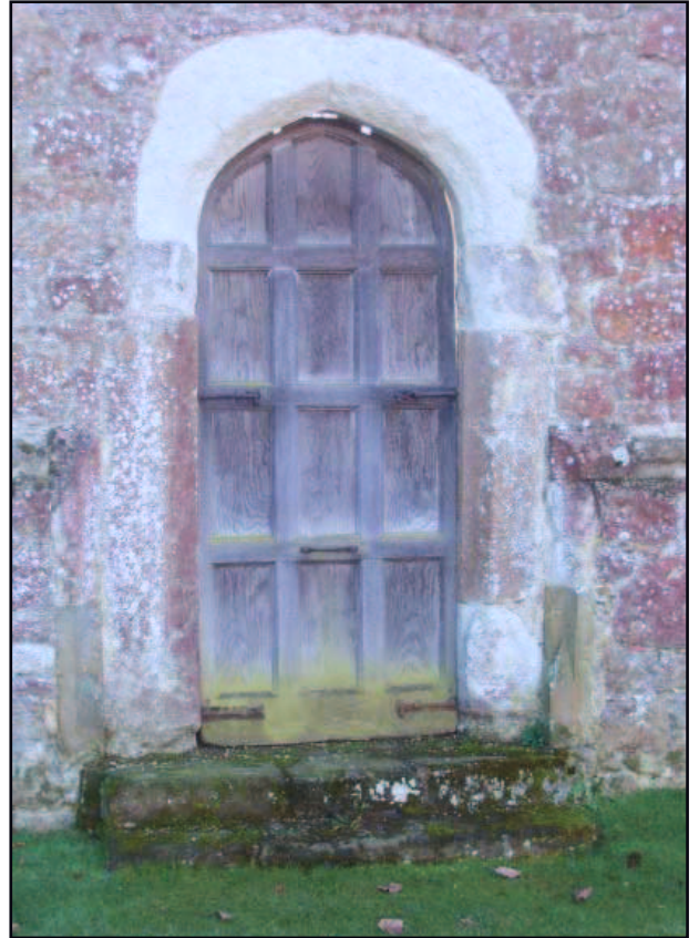
Plate 11: Current central doorway in the north facade
