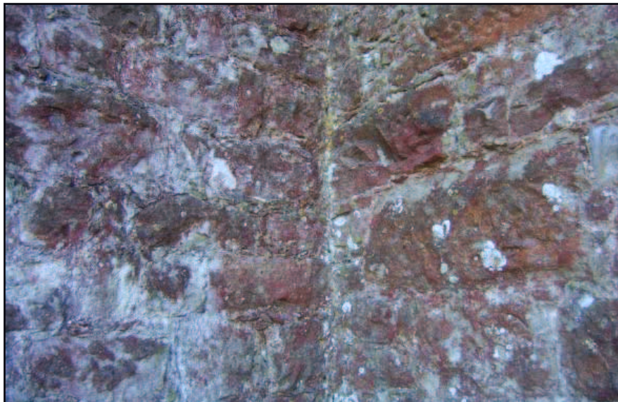
Plate 7: The southern end of the east range
