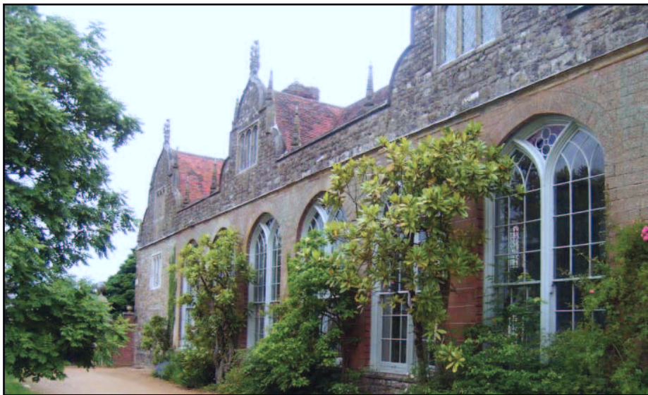
Plate 2: General view of the south facade
