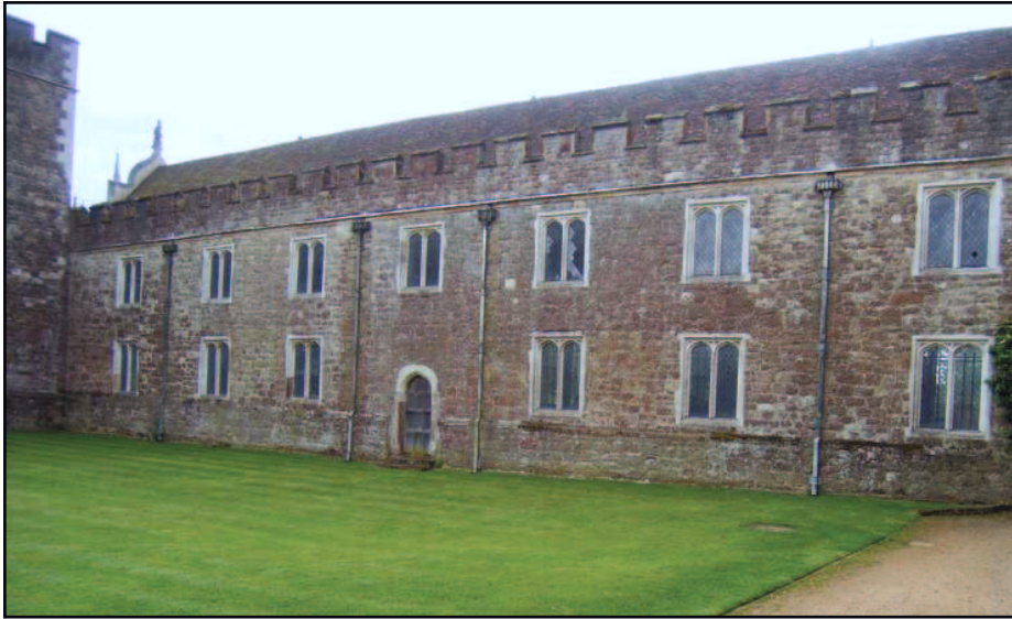
Plate 1: General view of the north facade
