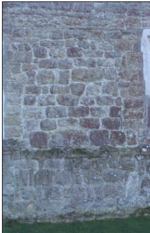
Plate 9: Blocked doorway in the north facade (west)
