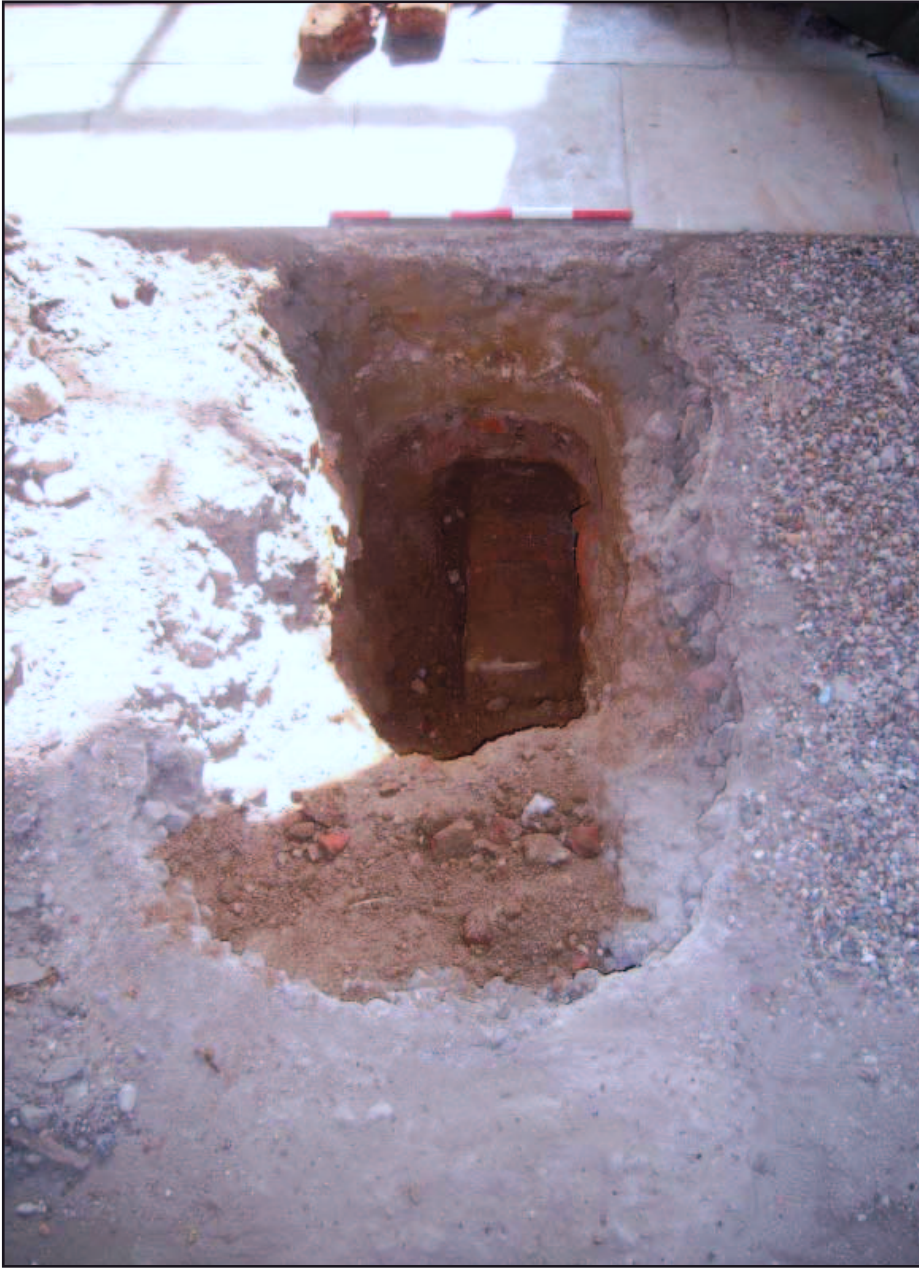
Plate 39: Trench 3 within Orangery showing surviving footings from former partition
