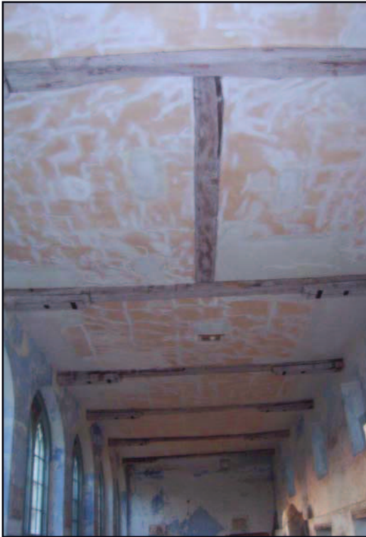
Figure 26: Western half of the current ceiling
