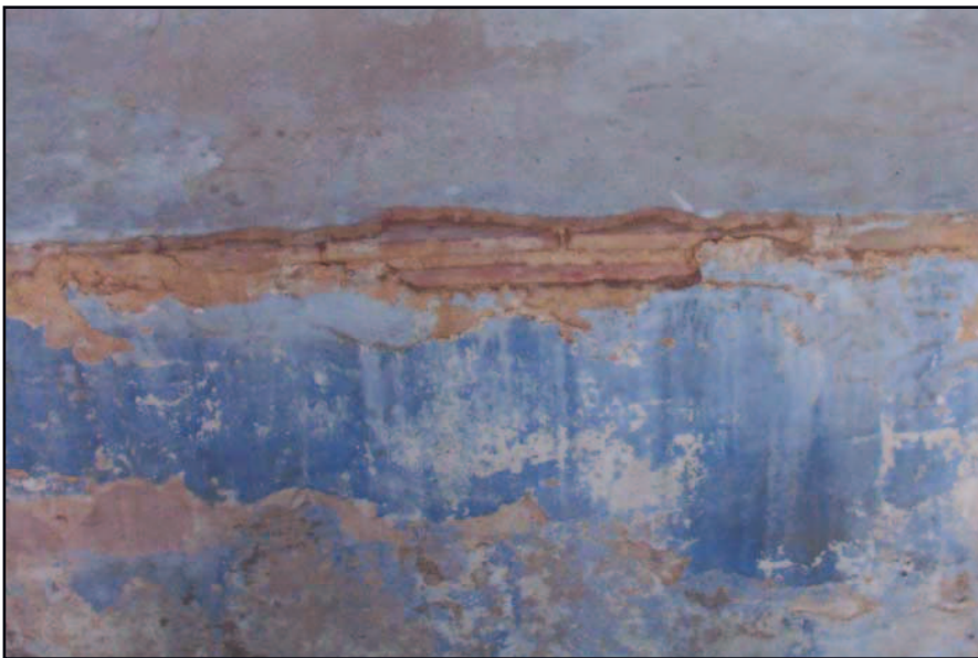
Plate 20: Sill of a window on the ground floor, north wall
