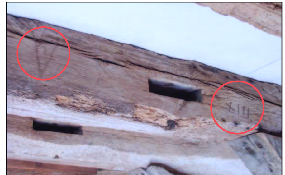
Figure 29: Roman numerals and carpenters marks
