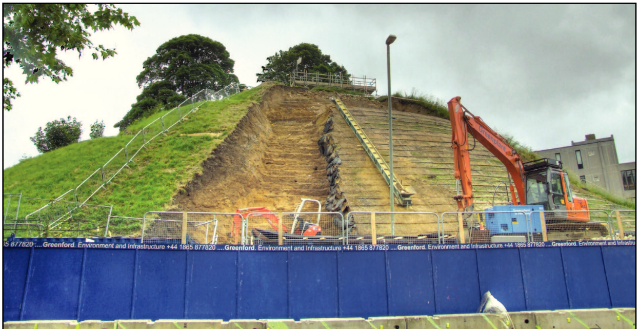
Plate 6: View of Gabions in place and their construction, wall visible at the top
