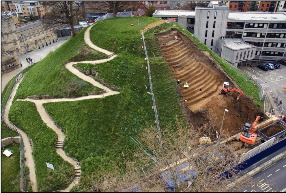
Plate 3: Working view removing slumped material of mound
