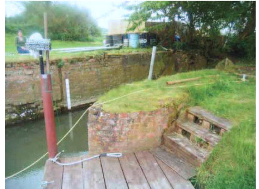
Plate 2: View of east end of central pier between wheel pits
