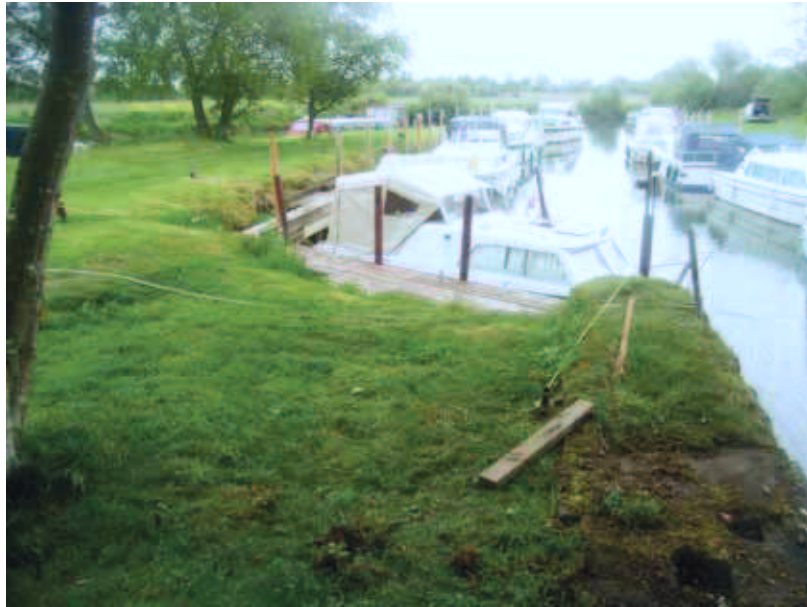
Plate 1: General view of infilled north wheel pit and tail race beyond
