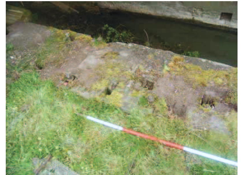
Plate 8: Holding-down bolts in upper face of stone bearing in south wall
