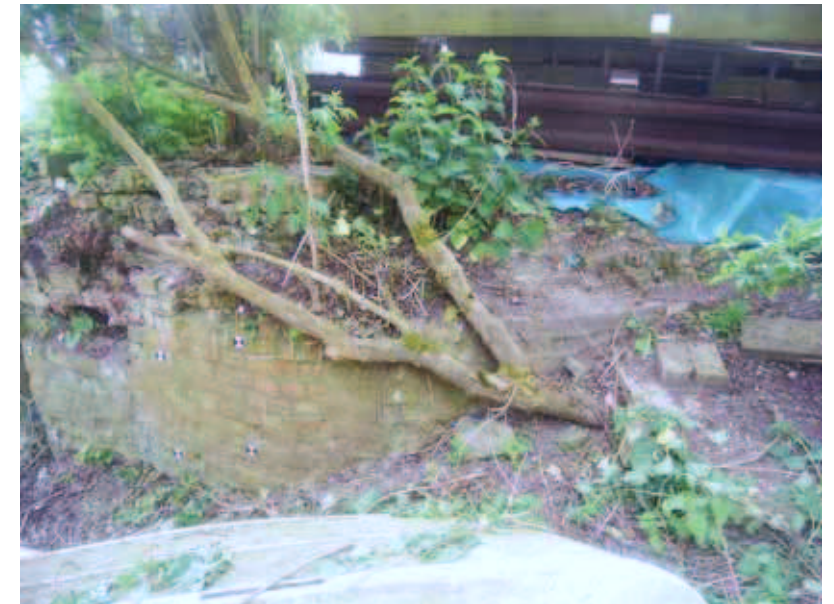
Plate 4: Curved west end of south wall
