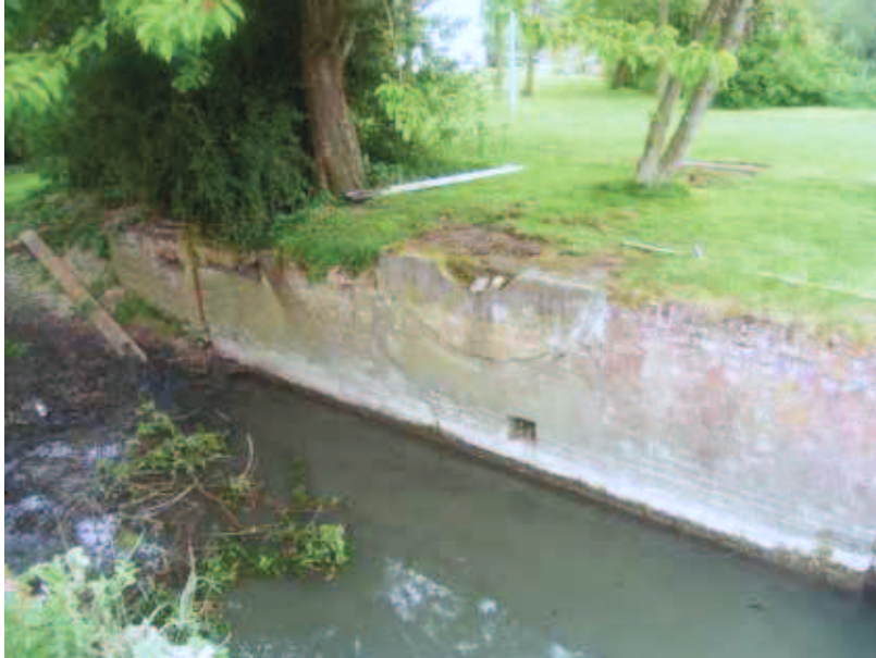
Plate 5: General view of north wall and infilled pit behind
