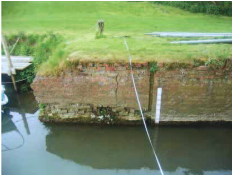
Plate 3: East end of south wall
