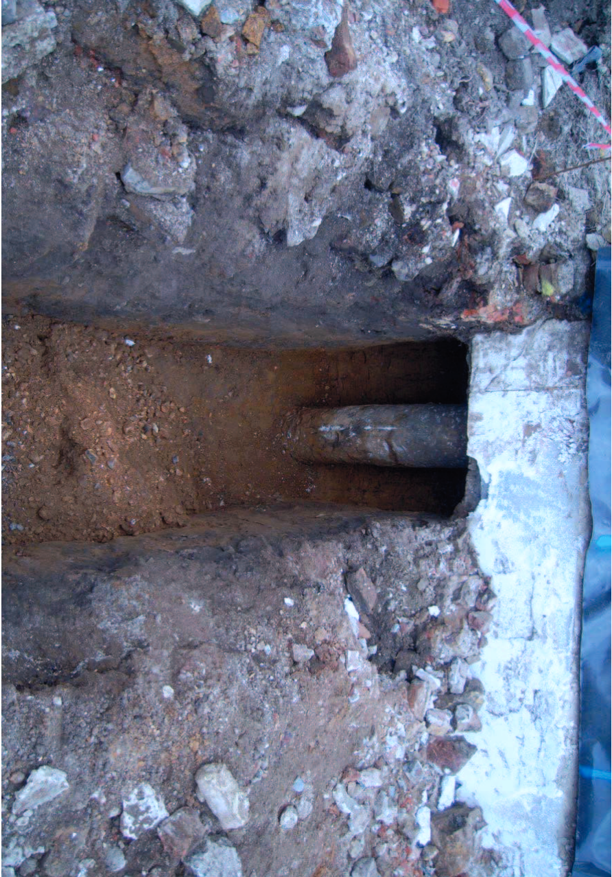
Plate 5: Underpinning trench, showing pile foundation
