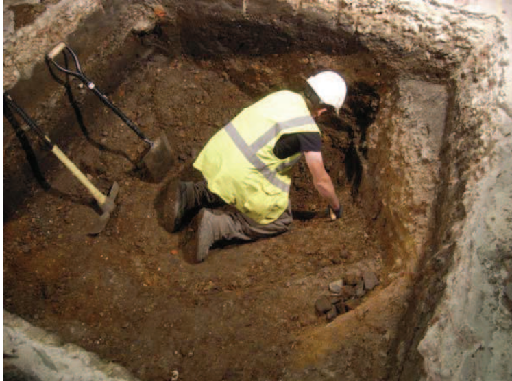
Plate 3: Test Pit 3 - Quarrying cut under excavation
