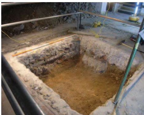
Plate 1: Test Pit 1 - Looking north west
