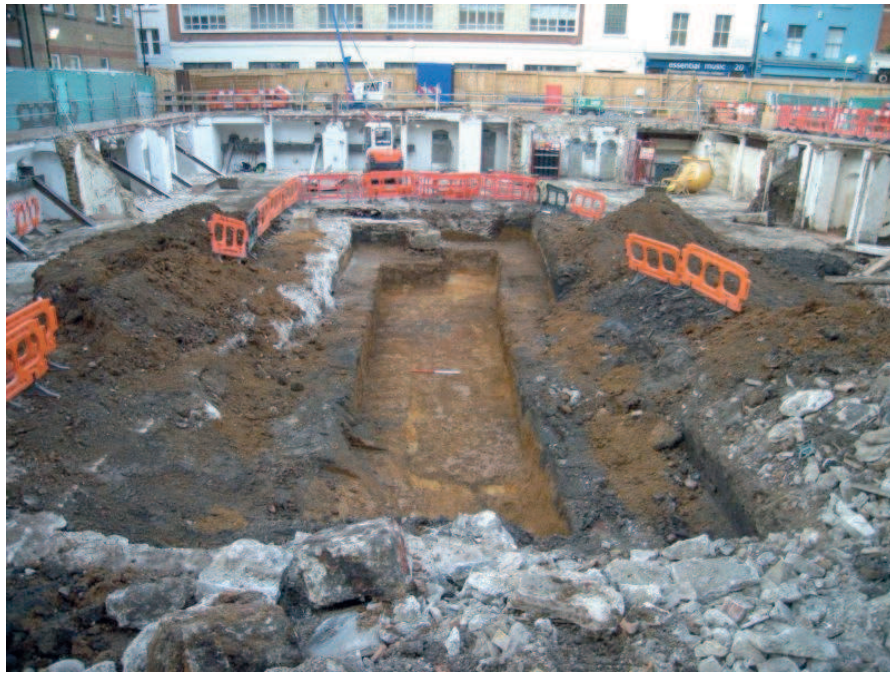
Plate 1: Uneven nature of the quarrying, looking west
