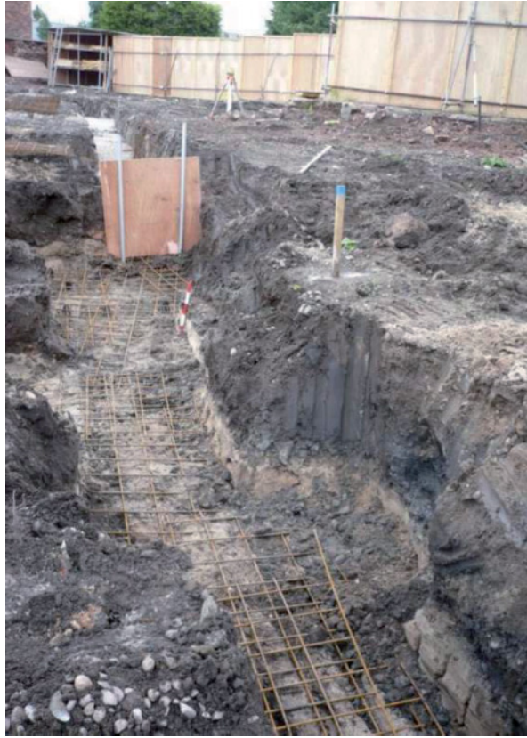
Plate 1: Roman road 119 in north-facing section with construction work ongoing
