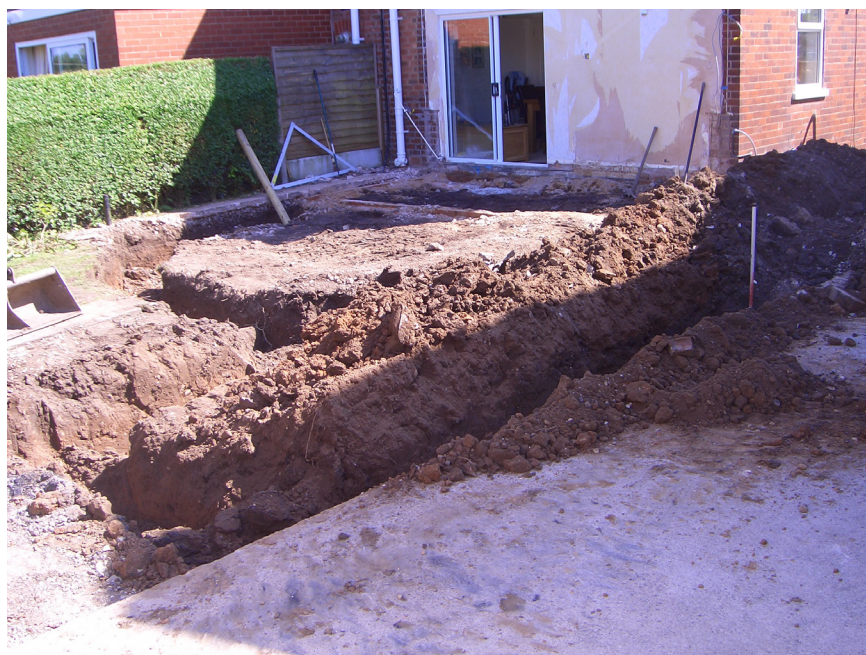
Plate 2: the rear of 53 Dowbridge following the excavation of the foundation trench
