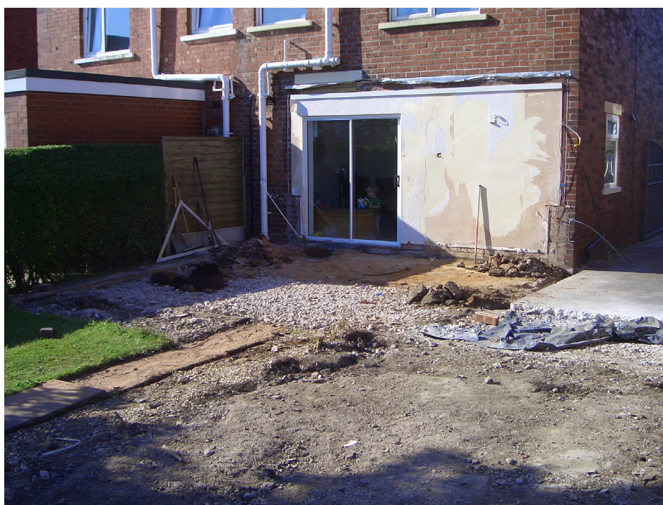
Plate 1: the rear of 53 Dowbridge prior to groundworks
