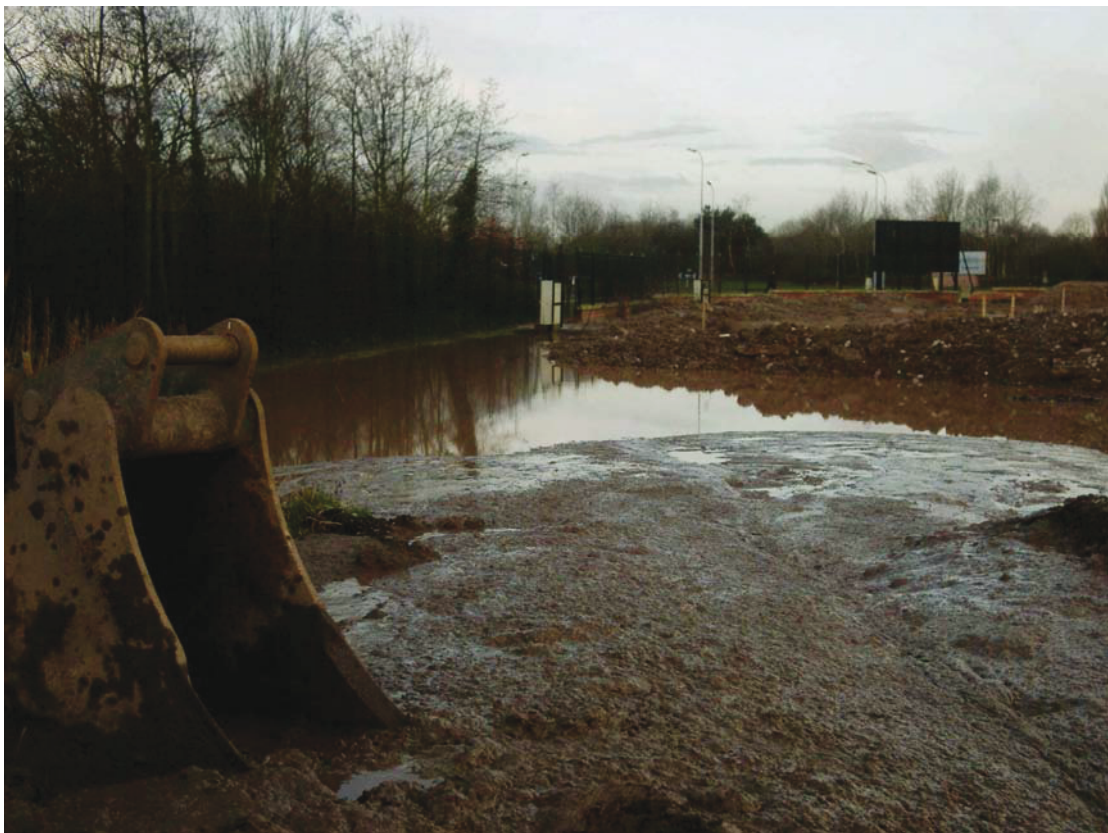
Plate 4: General shot of Site 13, looking west
