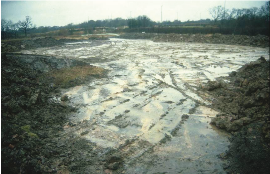
Plate 1: Shot of topsoil strip
