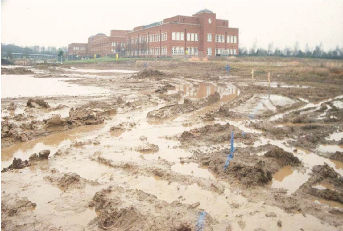
Plate 3: Shot of excavated watching brief area
