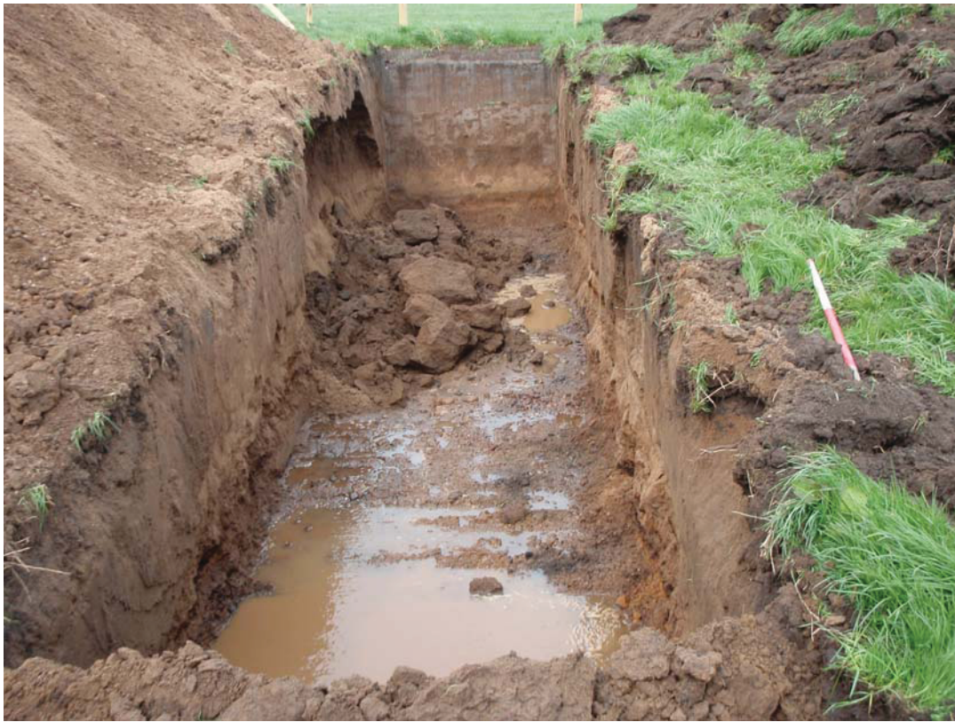
Plate 7: Trench 3, looking north-west
