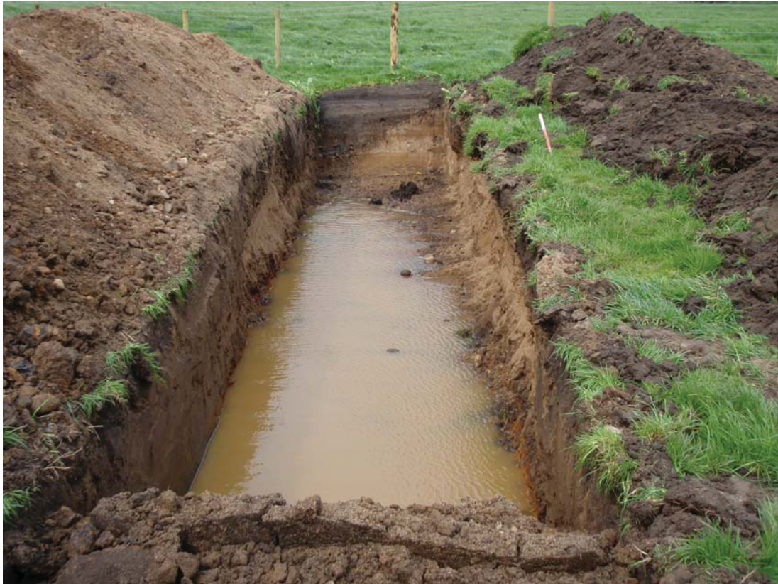
Plate 5: Trench 1, looking north-west
