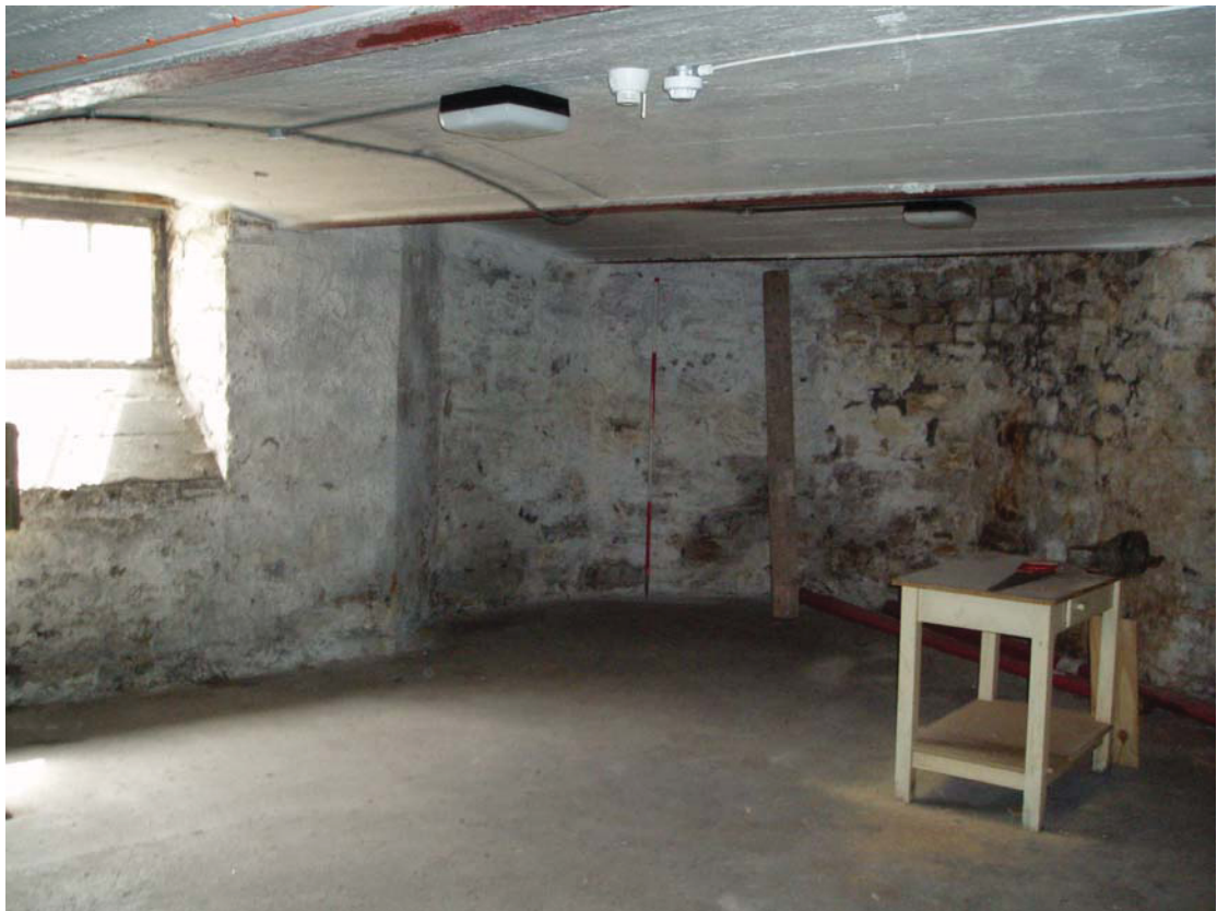
Plate 13: General view of one of the rooms within the sub-basement
