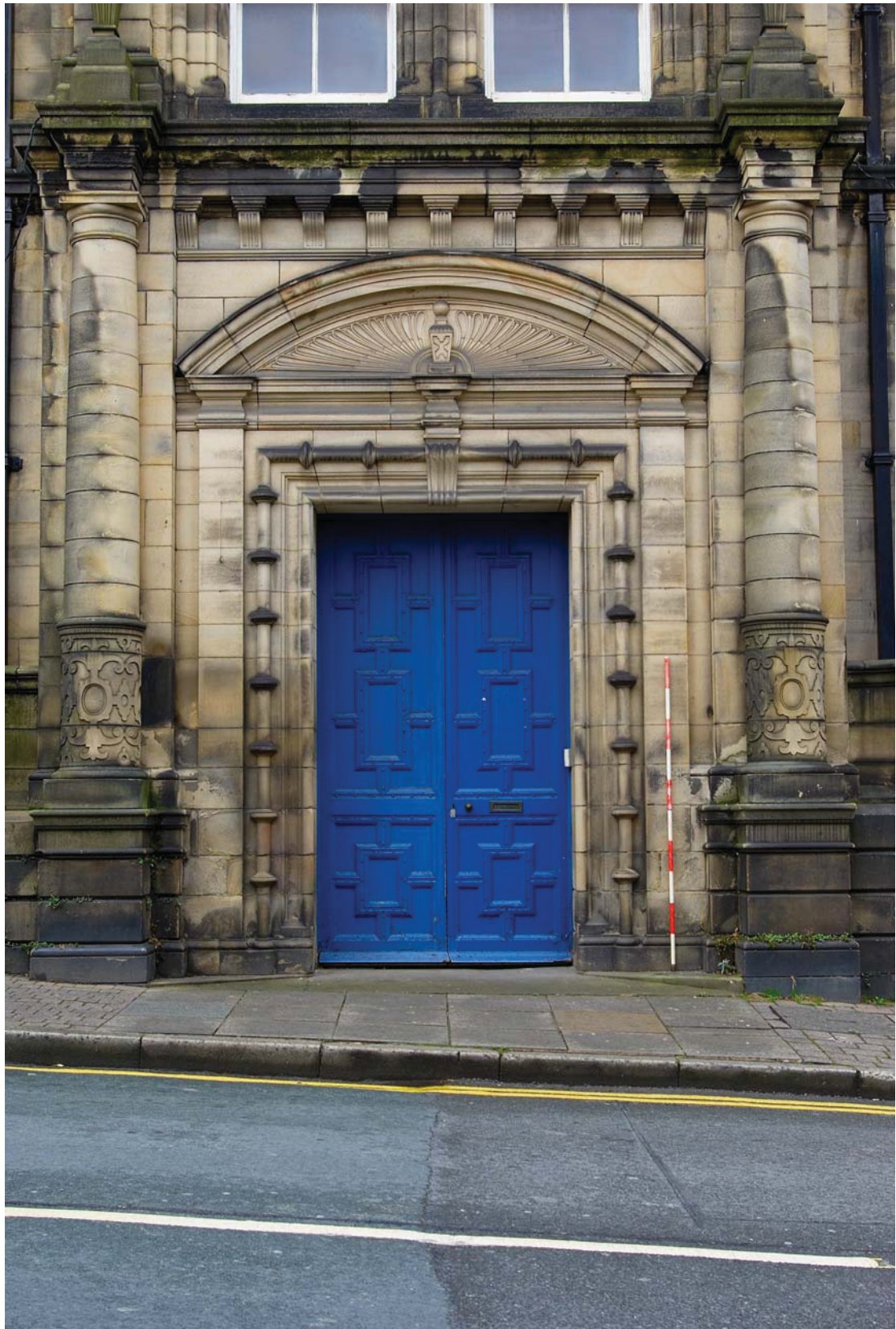
Plate 4: The formal entrance to the Storey Institute on Meeting House Lane (south elevation)
