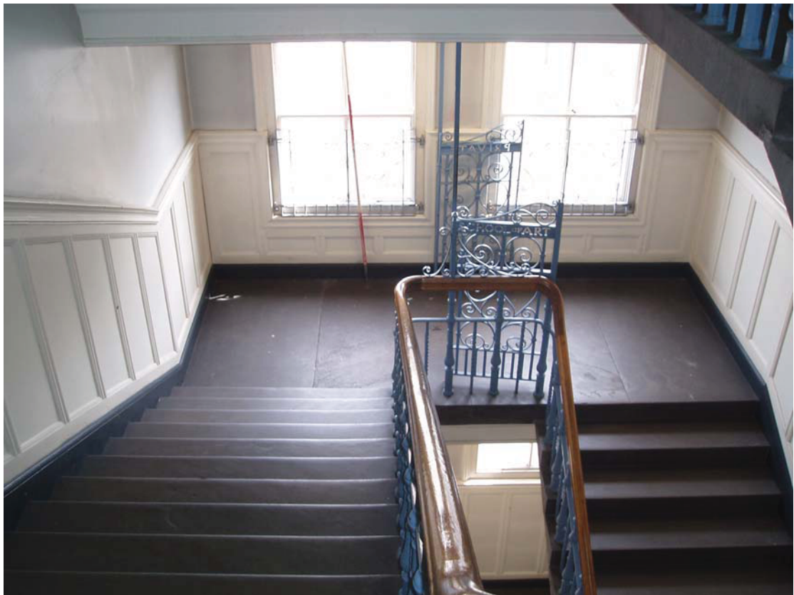
Plate 18: Detail of the staircase in the original phase of the building
