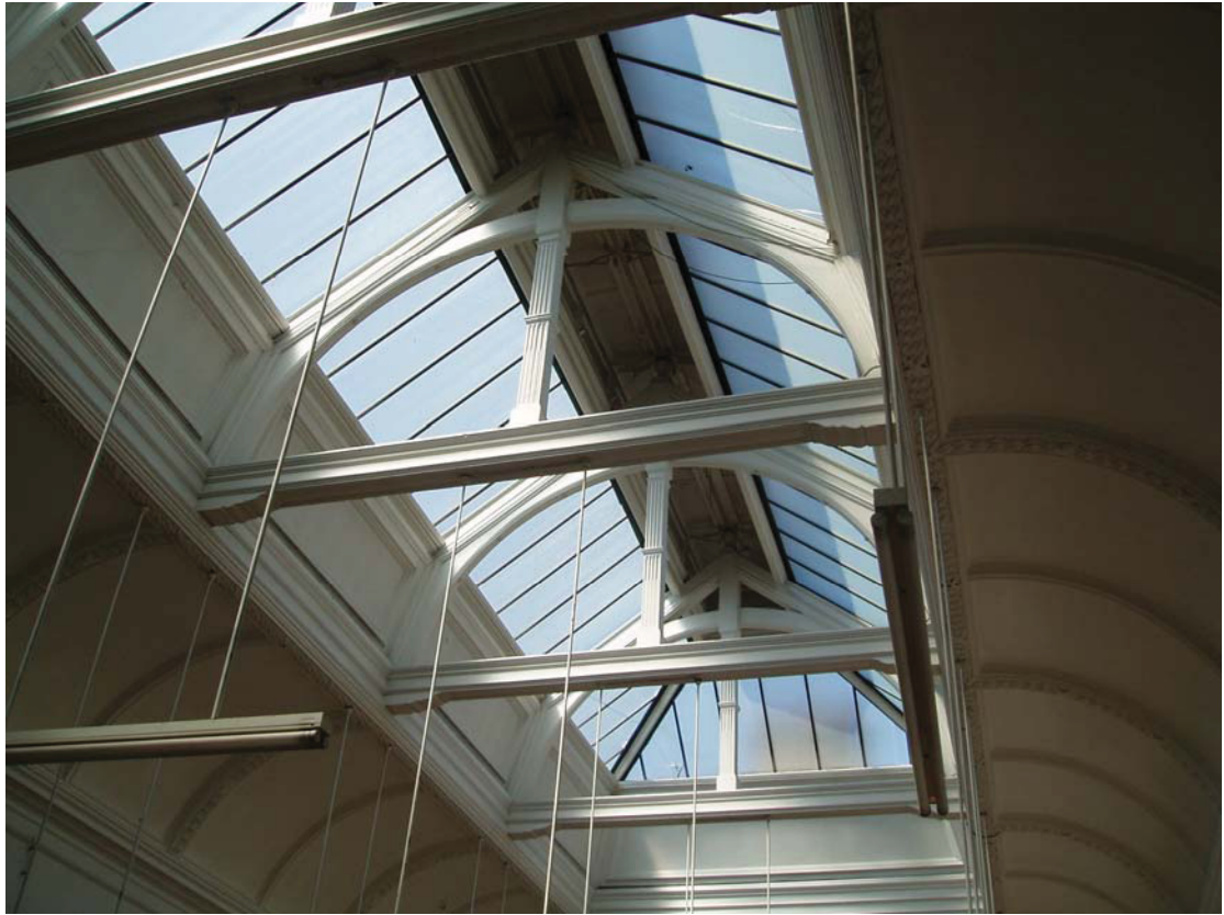
Plate 14: Detail of the ceiling within the gallery
