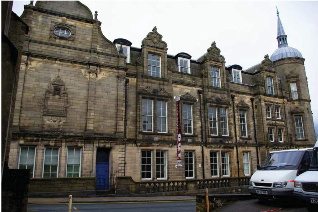
Plate 1: The south elevation of the Storey Institute
