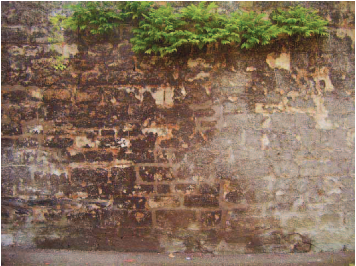
Plate 5: President's Lodgings Wall, Magdalen College: Coursing on north face, looking south
