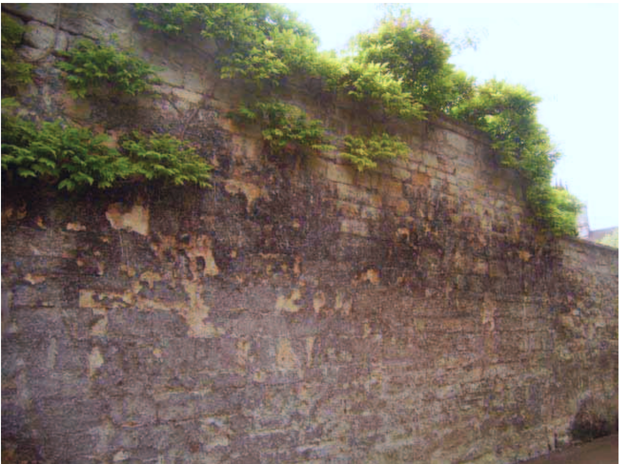
Plate 6: President's Lodgings Wall, Magdalen College: Coursing on north face, looking south west
