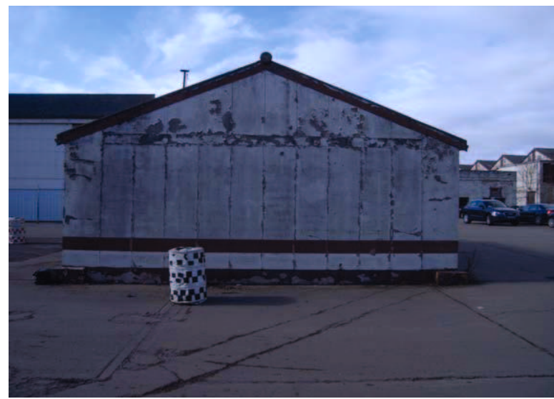
Plate 4: Building 81 East Elevation
