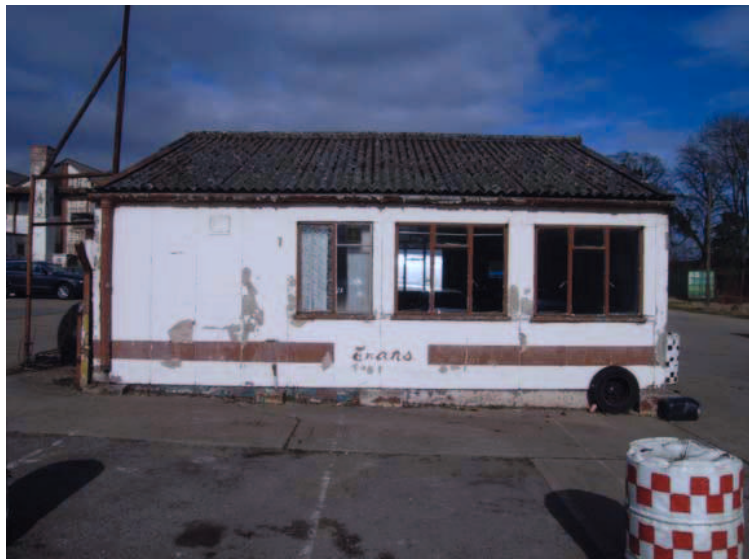
Plate 3: Building 81 South Elevation
