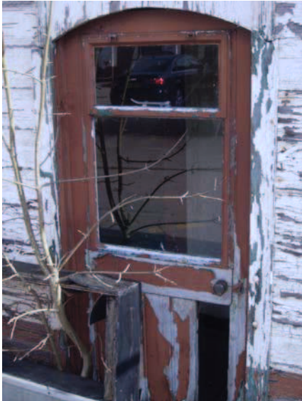
Plate 5: Door in West Elevation
