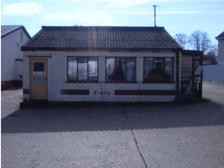
Plate 1: Building 81 North Elevation
