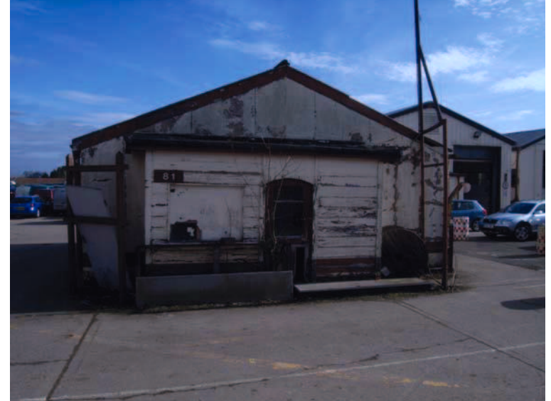
Plate 2: Building 81 West Elevation
