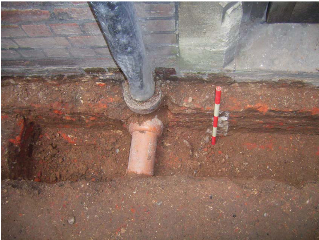
Plate 4: East - brick footing and ceramic pipe
