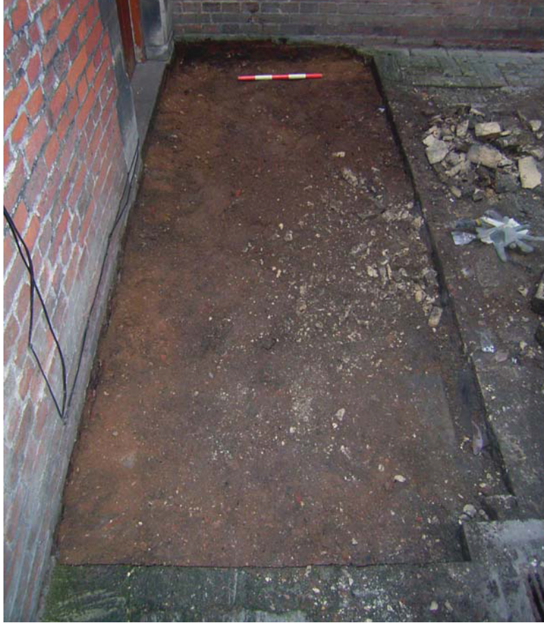
Plate 1: Removal of the paviers
