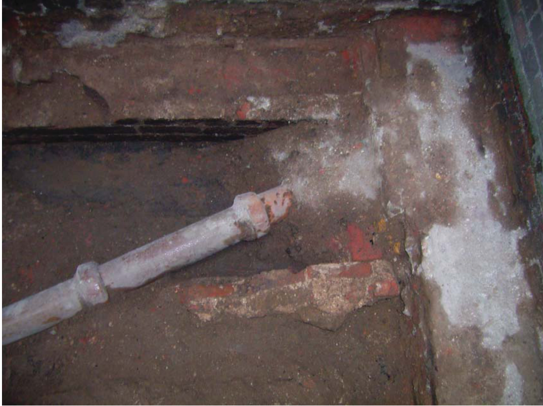
Plate 7: South east corner of excavation
