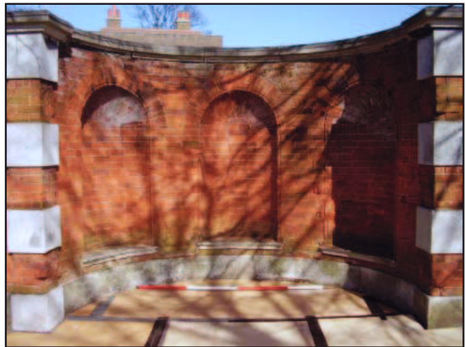
Plate 4: Recess in the wall containing niches
